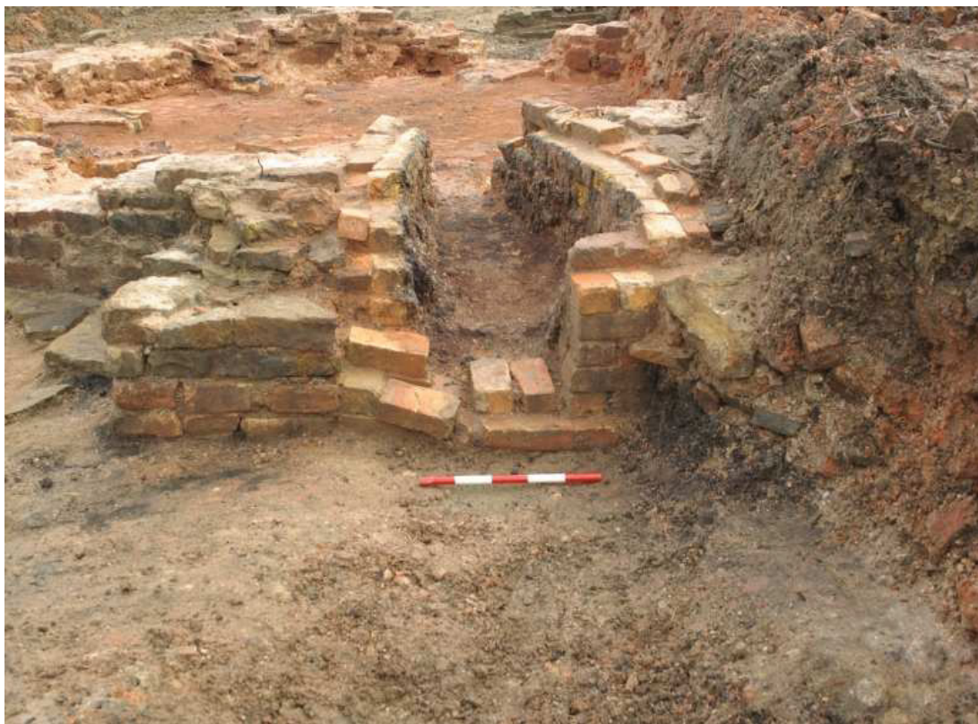
Plate 16: A typical flue showing refractory brick lining, and with a stone pier to the left
