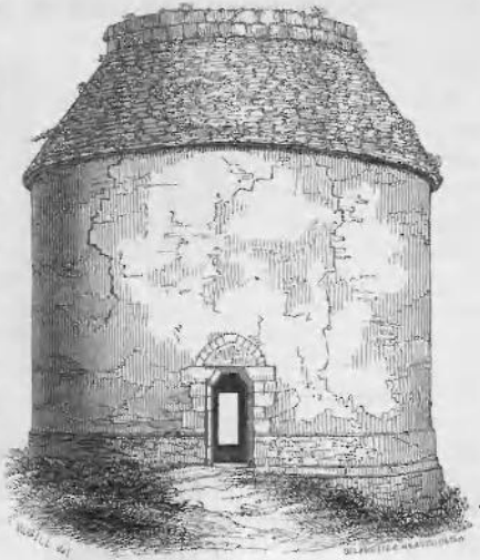
Exterior of Dovecot.
