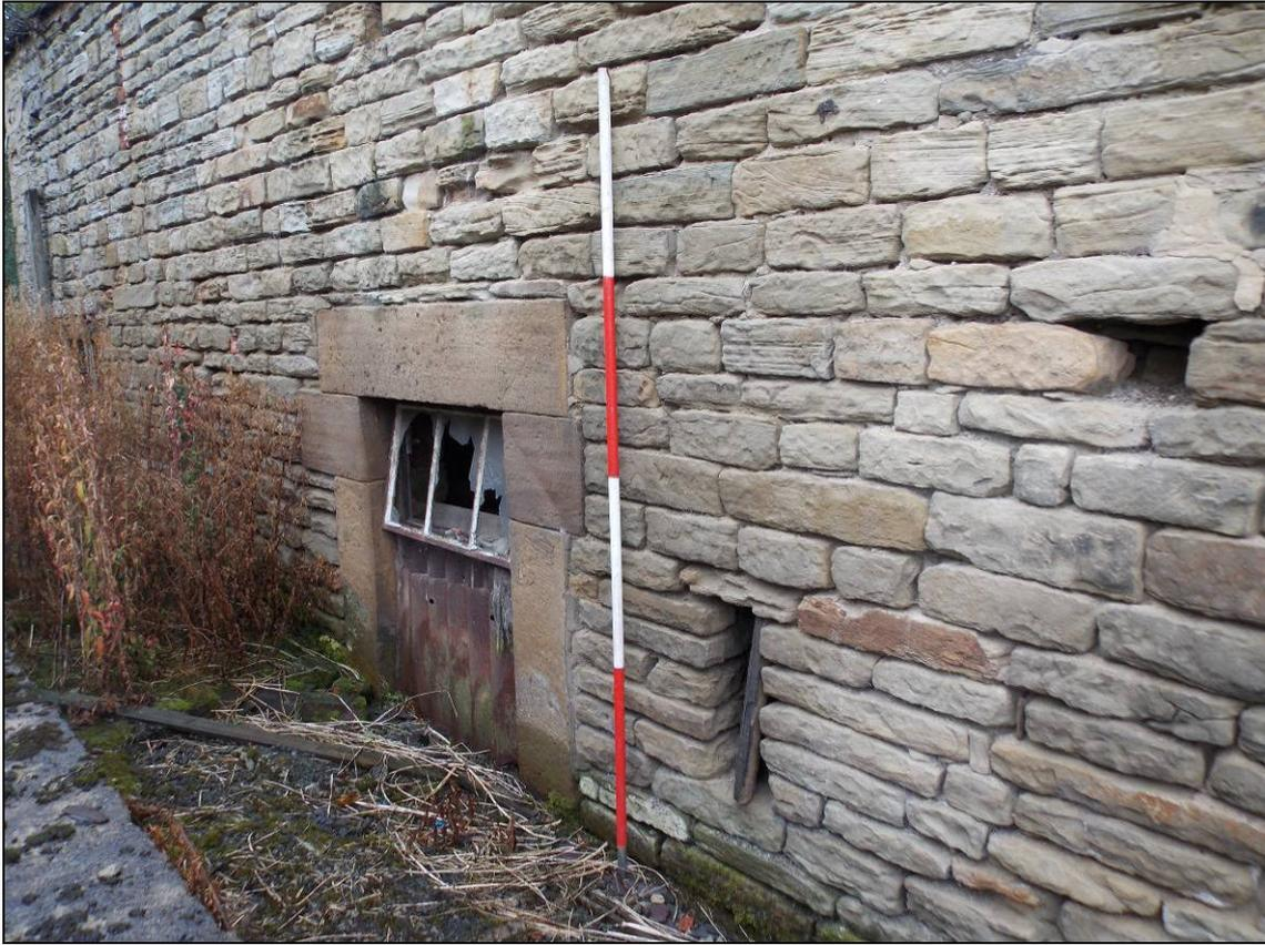
Figure 9: Detail of former doorway and ventilation slit within the south elevation
