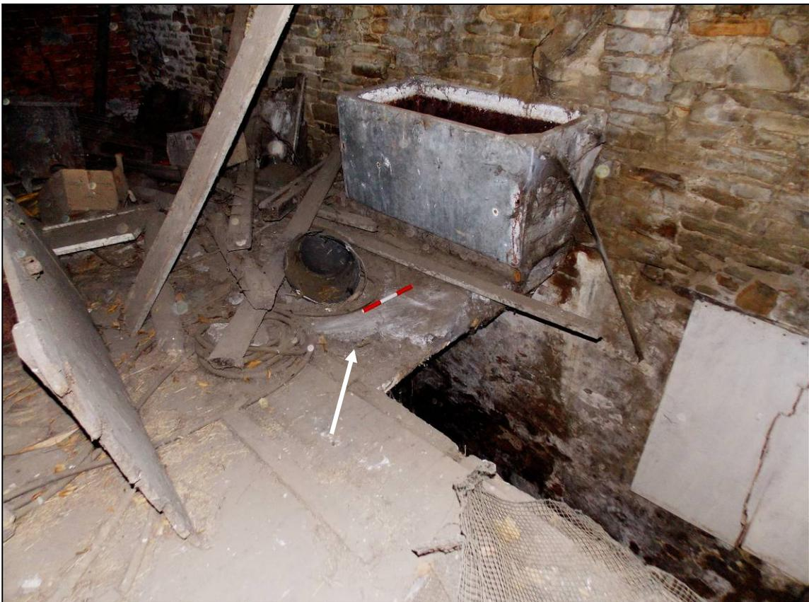
Figure 16: Western side of the first floor with remnants of former lime ash screed over floor boards (arrow)
