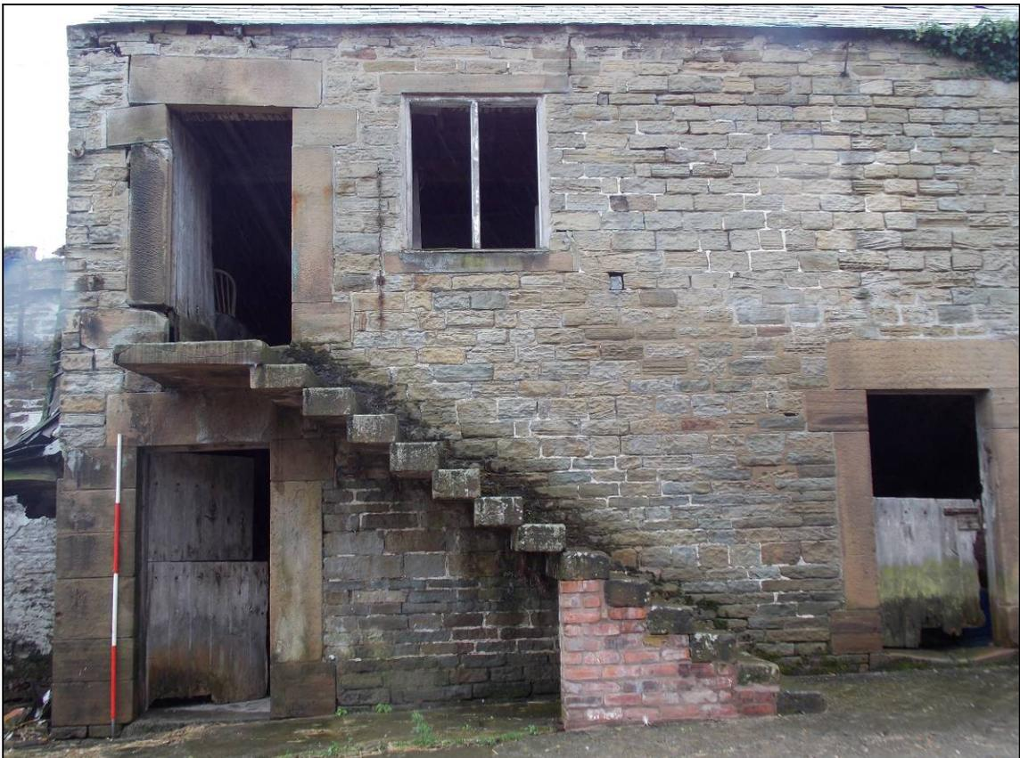
Figure 6: Eastern side of the north elevation with cantilever staircase
