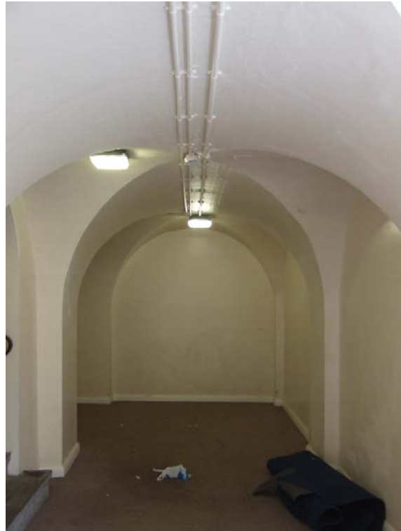
Plate 7: Block K, vaulted basement.
