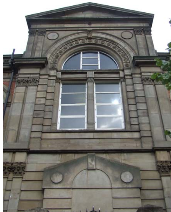
Plate 10: Block J, street elevation; central bay.
