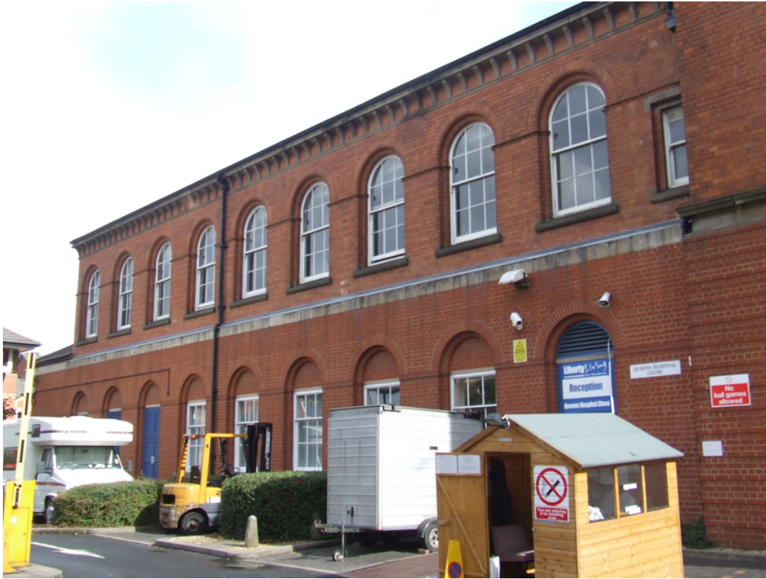
Plate 11: Block J, west elevation.
