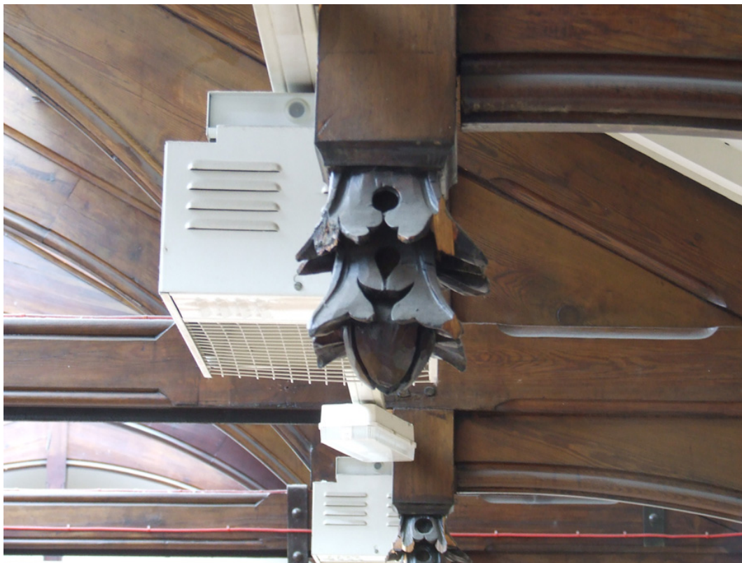
Plate 14: Block J, first floor, detail of carved hammer-beam pendant.
