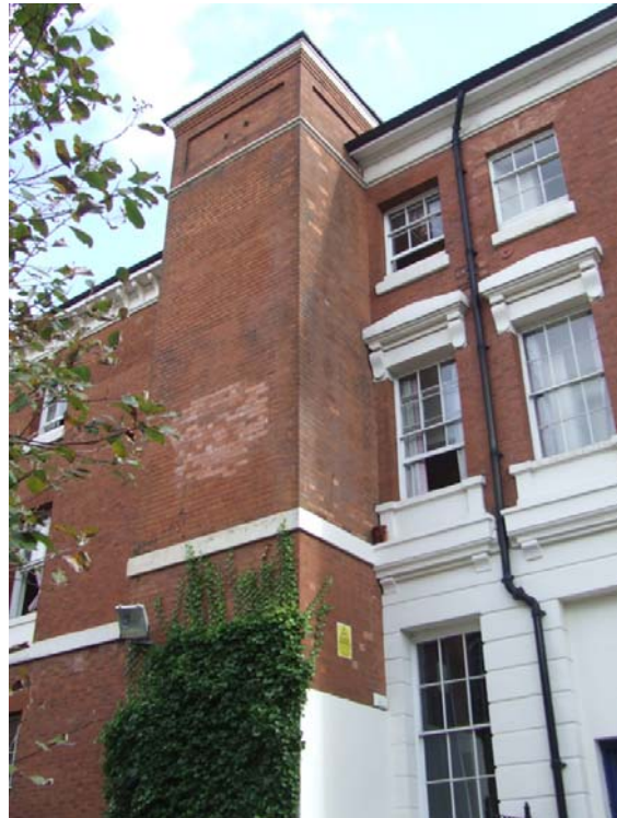
Plate 5: Block K, west elevation; secondary turret,.
