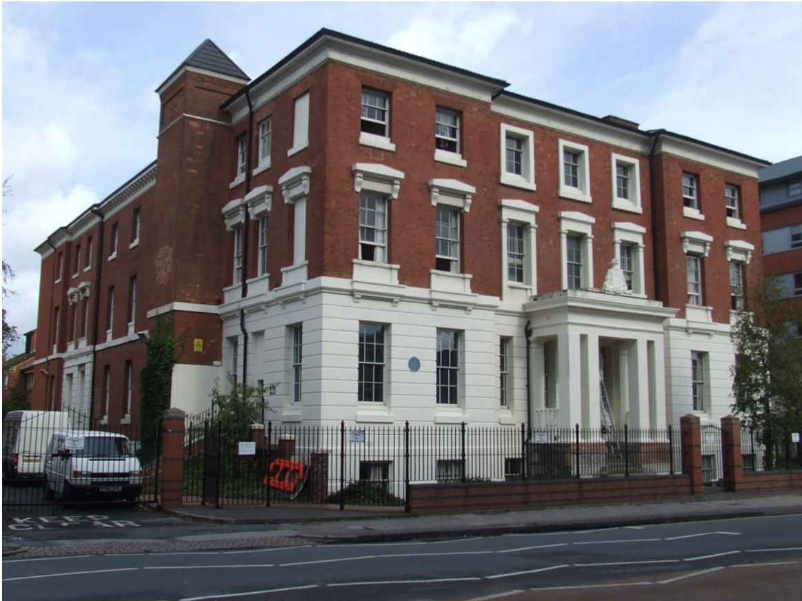
Plate 1: Block K, street (south) elevation.
