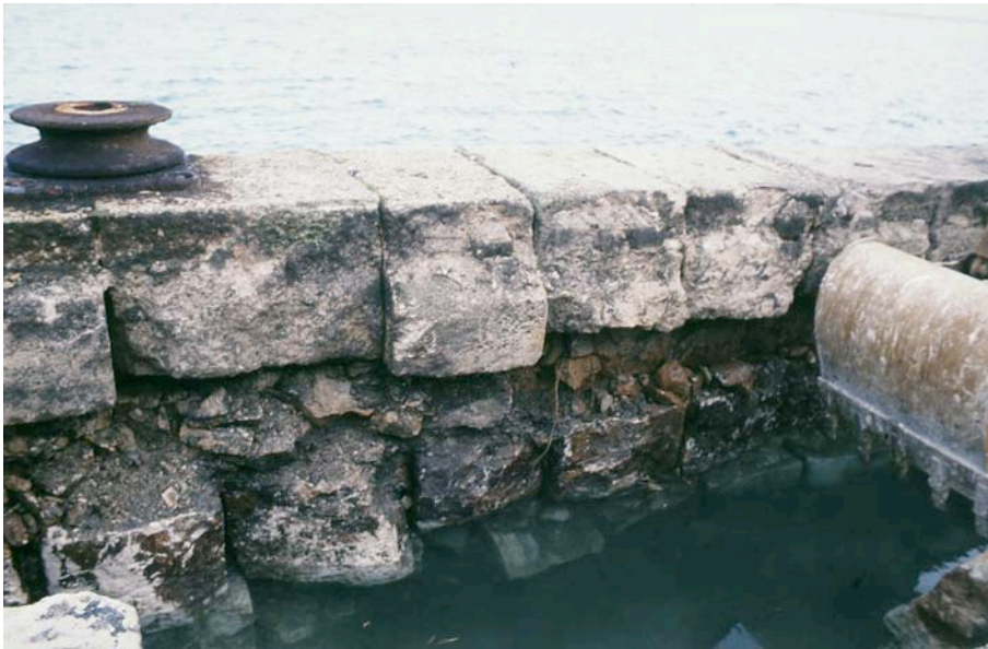
Plate 7: Abutment 2 showing details of the rear of the ashlar facing.
