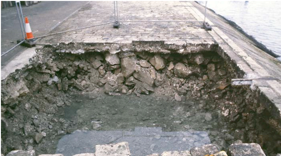
Plate 5: Mooring Point 5 showing rubble fill
