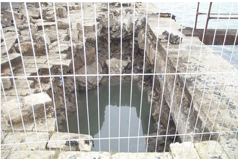
Plate 6: Abutment 3 showing rubble fill
