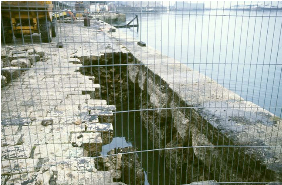
Plate 4 Abutment 1a with timber upright in foreground.
