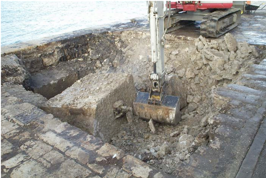
Plate 7: Mooring Point 4 showing inserted limestone block and tie bar.
