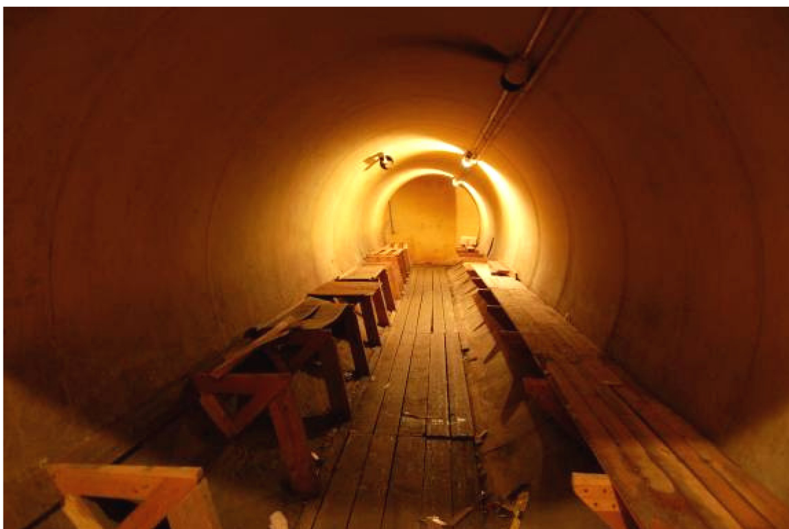
Fig. 27: The north gallery of a World War II air raid shelter below the Ecko Works, Southend, designed to withstand gas attacks (Photo: ECC)
