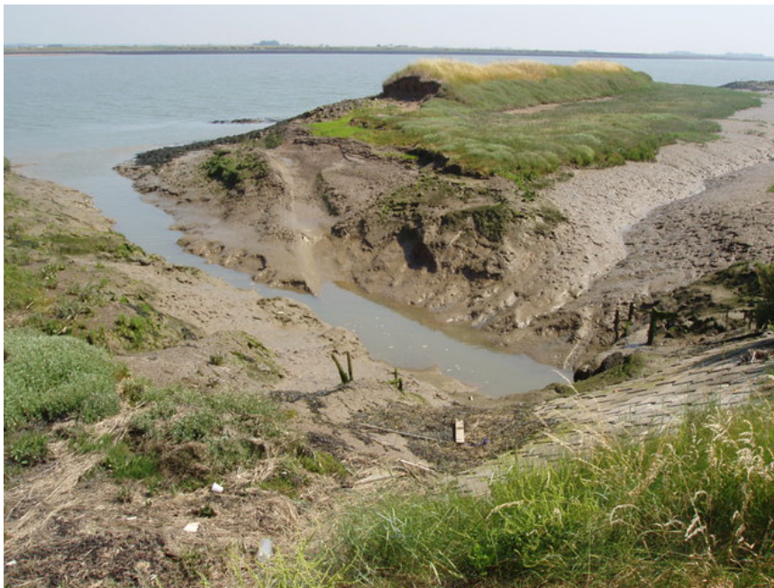
Fig. 19: Managed realignment at Wallasea; the cut through the seawall © Copyright David Williams and licensed for reuse under this Creative Commons Licence .
