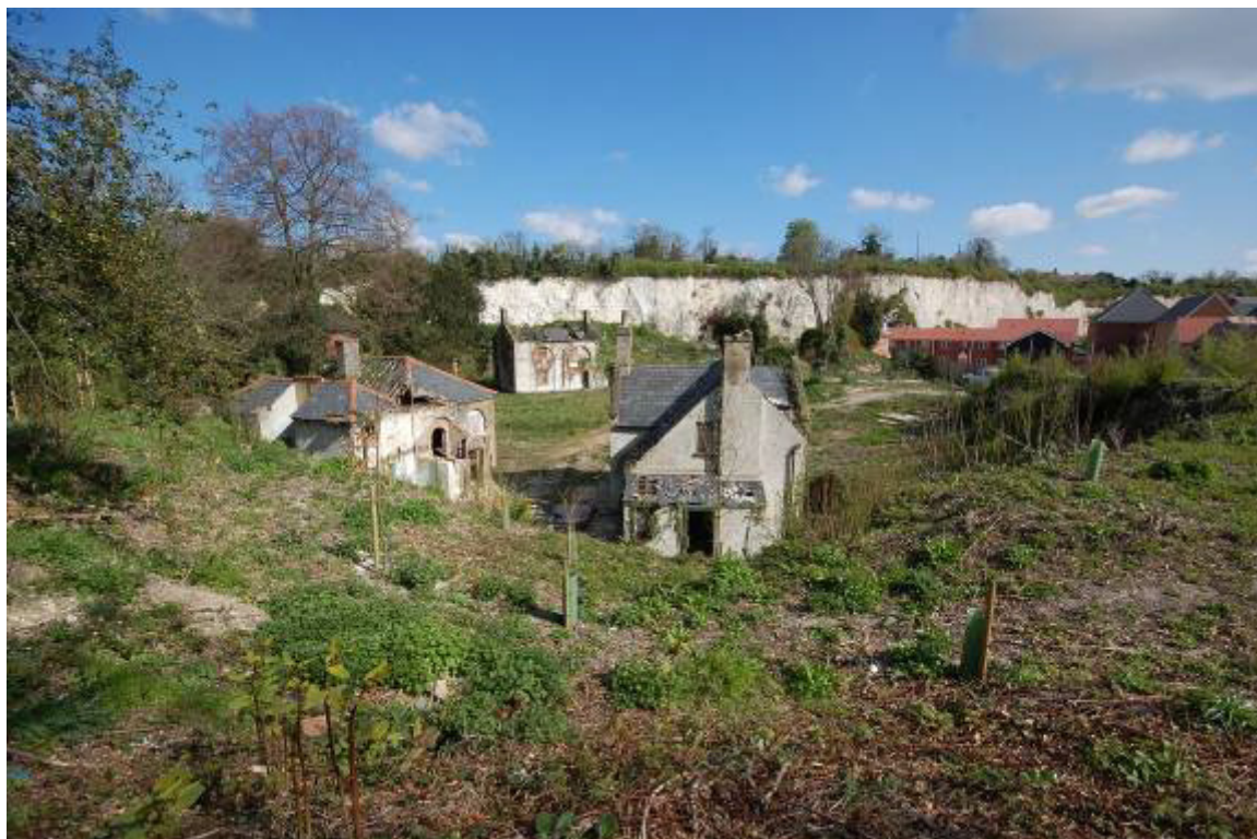
Fig. 31: Derelict historic buildings in Botany Pit (also known as Church Hollow) Purfleet. These are being recorded prior to renovation
