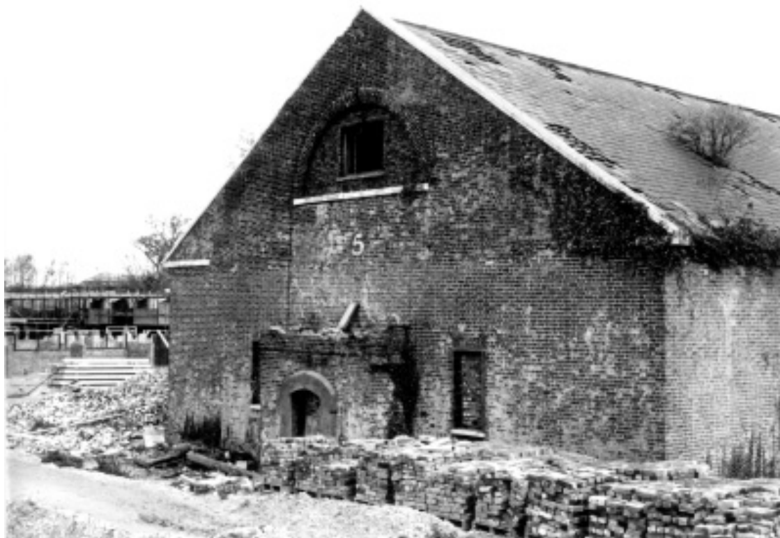
Fig. 30 Magazine No. 5, Purfleet. Constructed by 1765 this magazine would have held up to 9600 barrels of powder. This example is the only survivor of a group which were situated on the north bank of the Thames where the Mardyke enters it.
