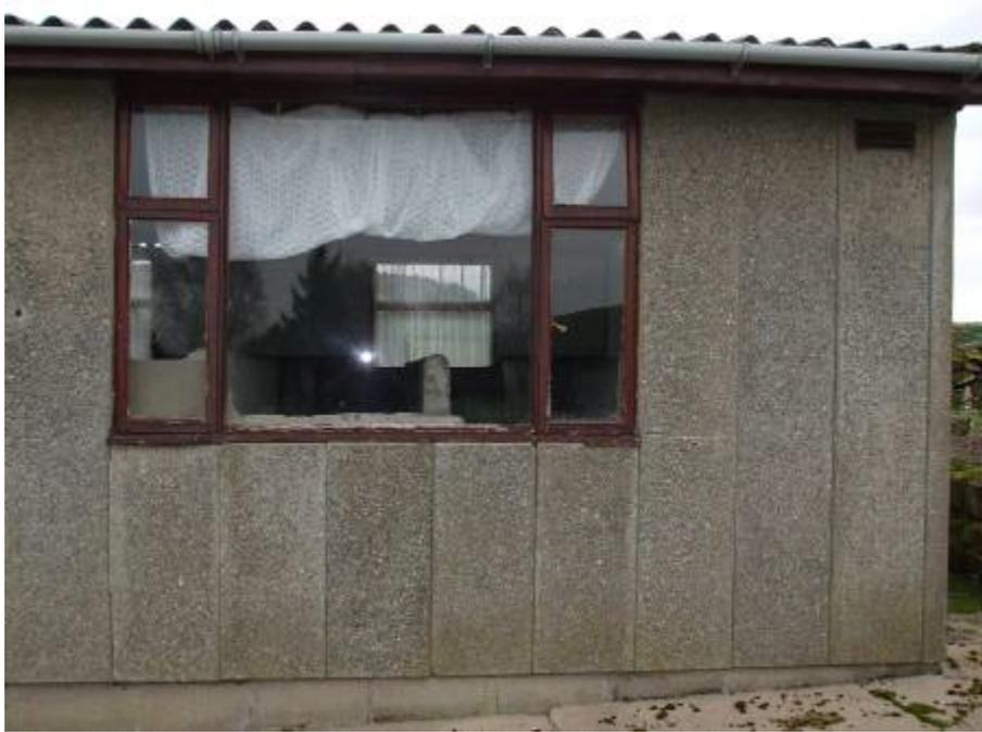
Concrete panels cut horizontally for the insertion of a window; SW wall
