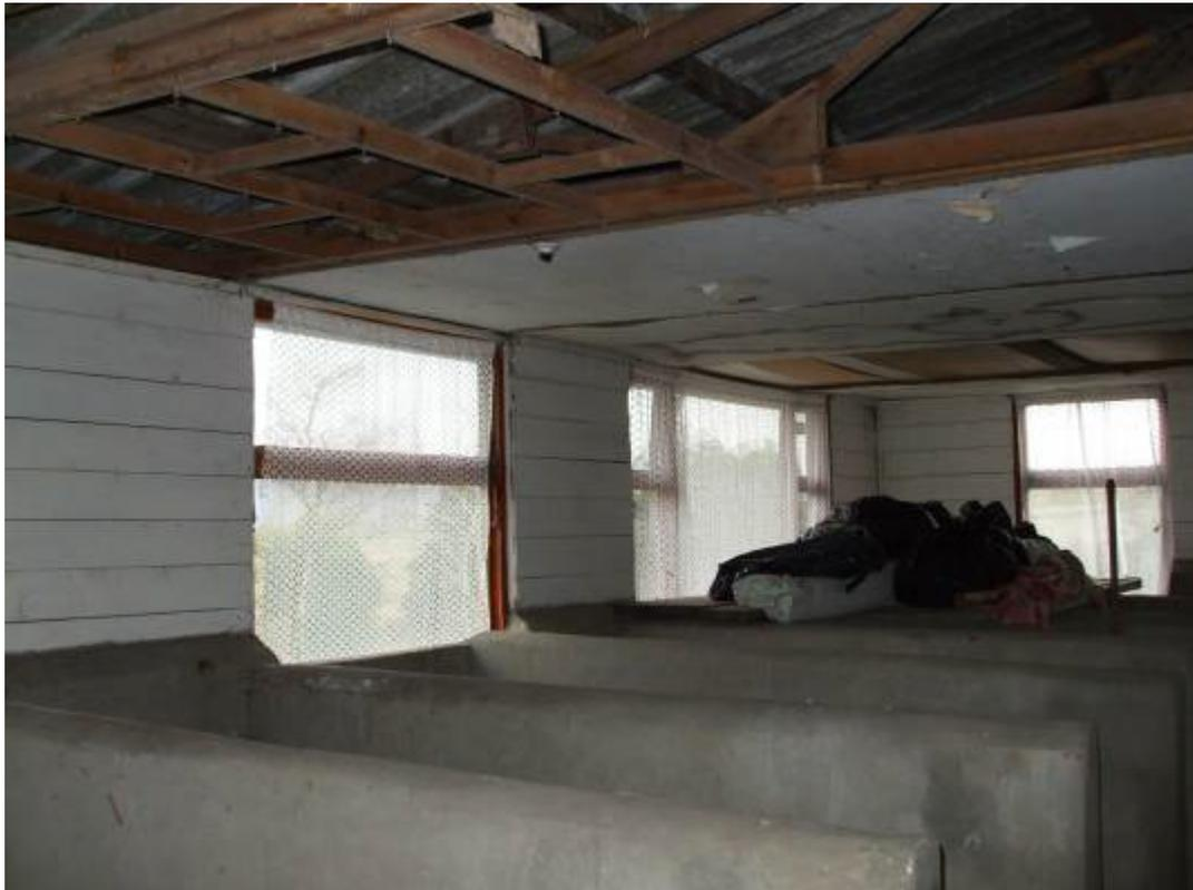
The wood paneling was covered by concrete stalls, probably for calf rearing
