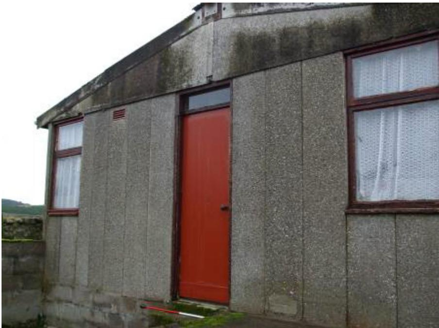
Concrete panels cut horizontally for the insertion of a window; NW wall
