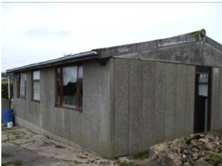
Facing N showing concrete base blocks to level the slope of the ground
