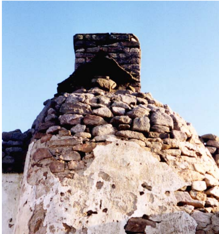
Fig 15 Eroded chimney breast, before conservation work
