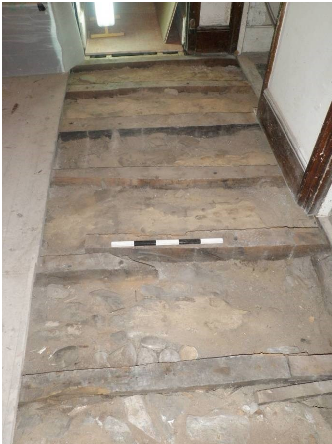
Fig 54 Remains of cobbled flooring revealed beneath the timber floor in the anteroom (former courtyard)
