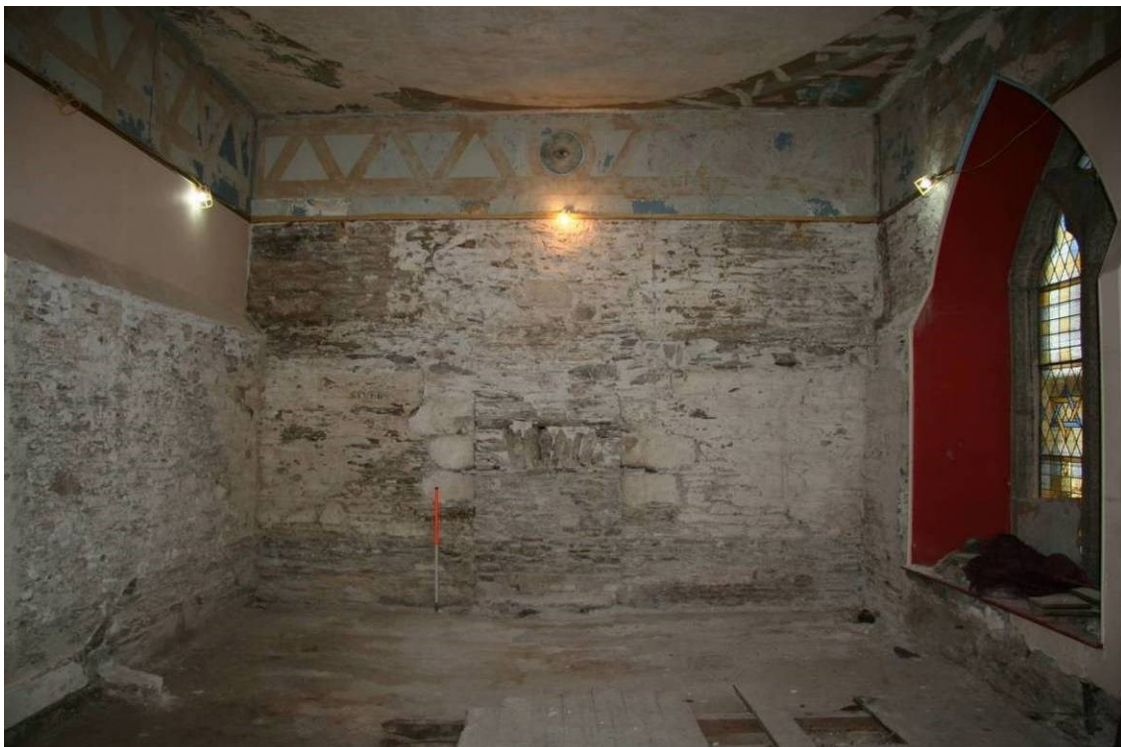
Fig 45 Removal of plaster at the north end of the same room has revealed the stone jambs of the original window, subsequently deepened to convert the opening to a fireplace
