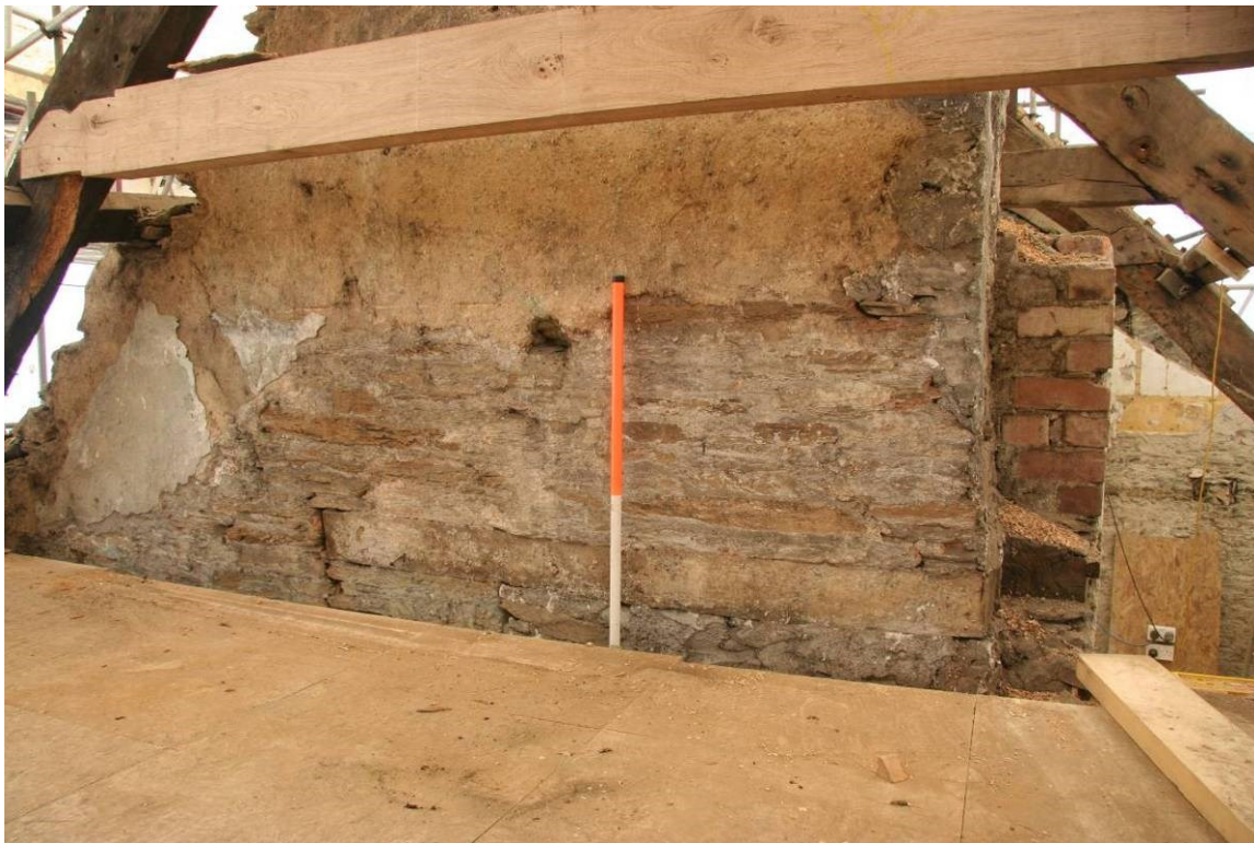
Fig 62 Early plaster survives on the north side of the cross wall; note also the wooden lintels of a former window
