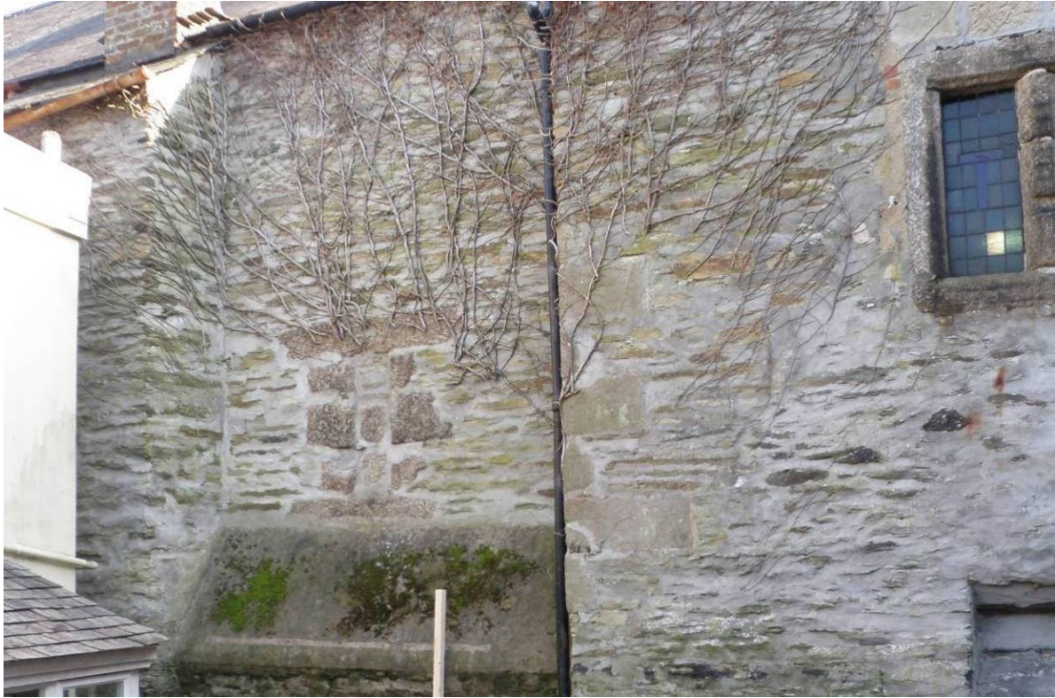
Fig 34 A blocked original granite-framed slit window in the west wall, and the original lateral chimney forming a buttress to the left.
