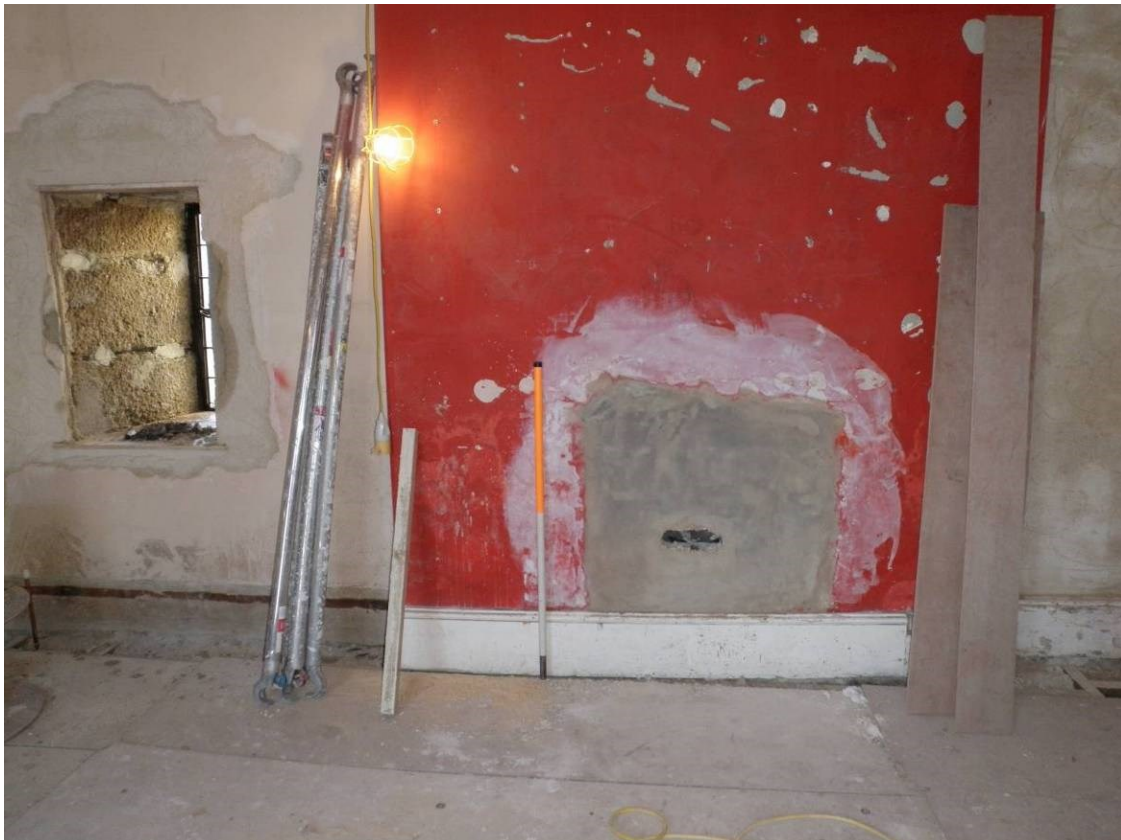
Fig 52 The original lateral hearth, since infilled with a Victorian fireplace
