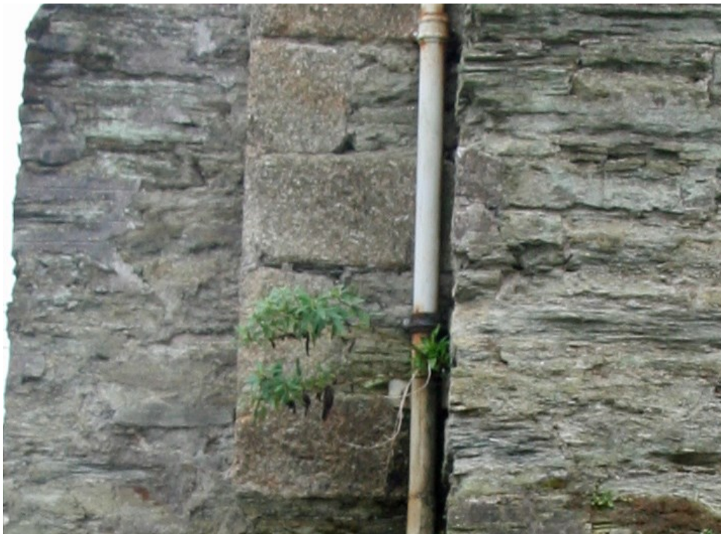
Fig 30 Chamfered detail on the granite quoins at the junction of Fore Street and Quay Street
