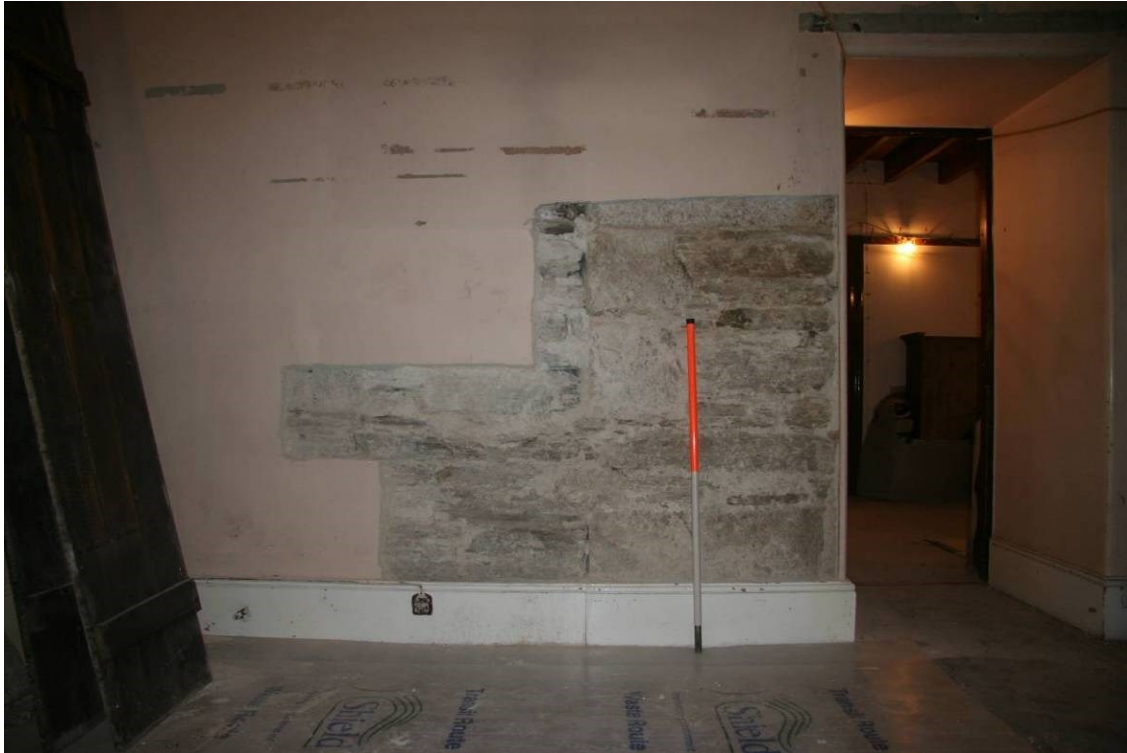
Fig 50 The right-hand jamb and base of a slit window in the S wall of the principal room This window, plus another higher up, are evidence that the space beyond was originally unroofed. The present roof structure was added after 1620, according to tree-ring analysis (Tyers 2010)
