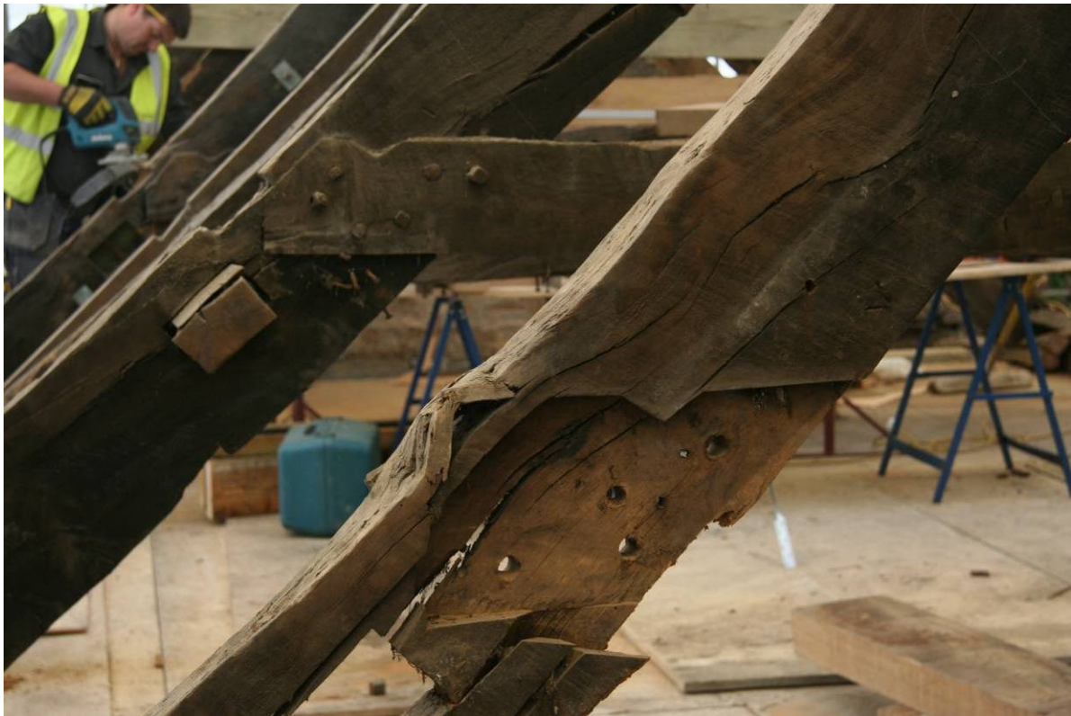
Fig 63 Example of a pegged collar joint on the 17 th century roof
