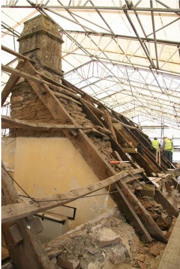
Fig 61 The cross wall is the only location where threaded purlins remain
