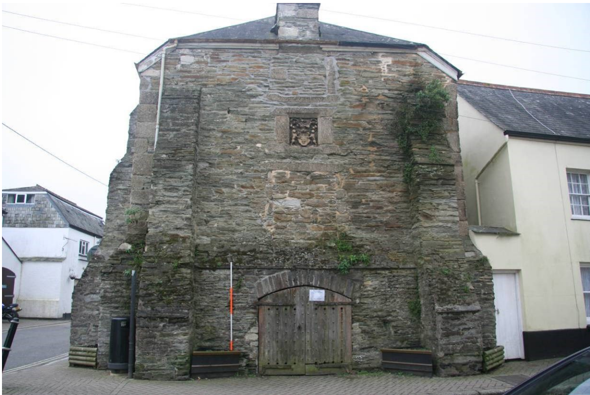
Fig 28 The north elevation of the building (facing Fore Street) shows many alterations including blocked windows in the original two upper floors
