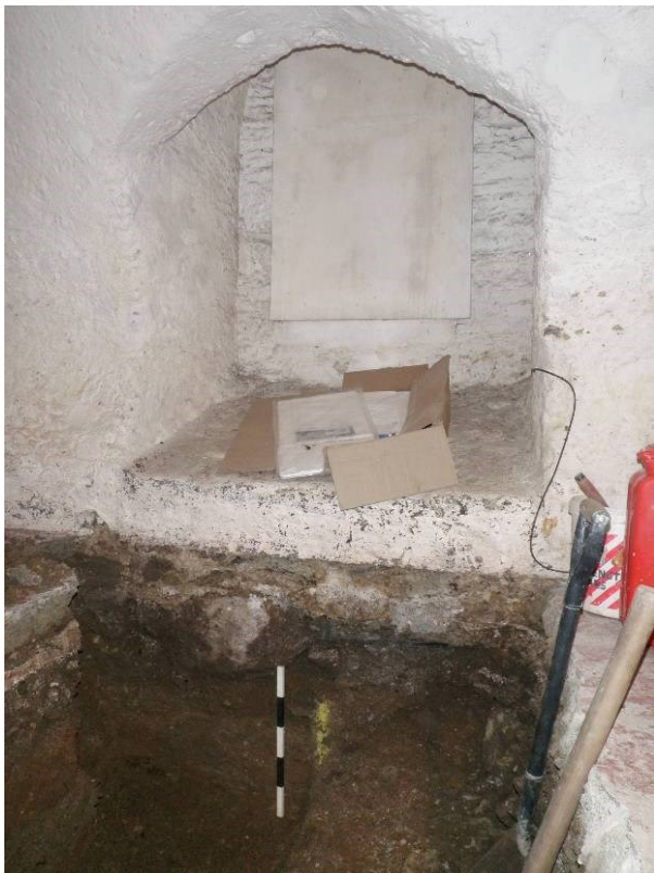
Fig 39 A small arched doorway in the E wall of the undercroft has been inserted through to a partially infilled recess, the internal jambs of the original recess can be seen to extend below the ledge of the lower infill walling by 0.8m. The inserted external opening had a new arched head added post-1878
