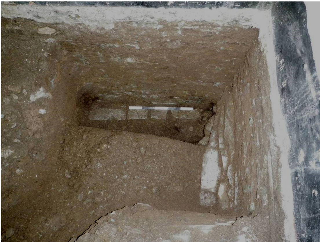
Fig 41 Excavation in the SW corner of the undercroft clearly reveals the foundation level of the Great Hall gable (centre), wall (26). The Convocation Hall foundations (27) (right) abut this wall and are set at a higher level
