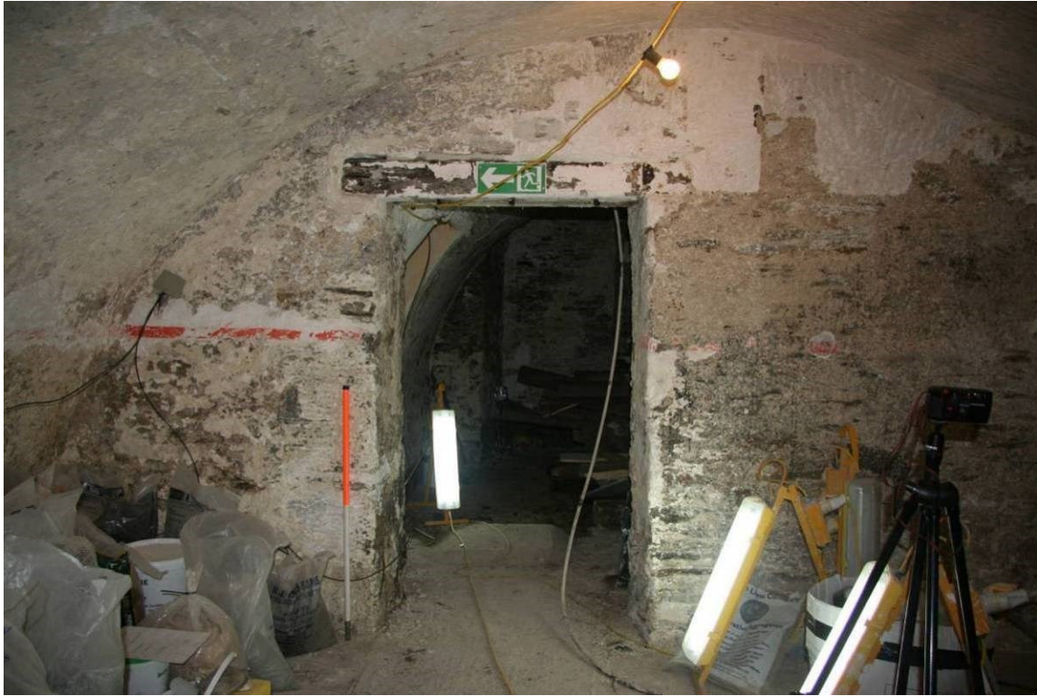
Fig 40 This internal doorway linking the two parts of the undercroft was altered to suit raised floor levels, by being widened (to the RH side) and a lintel inserted higher up. The original doorway set at a lower level was probably arched
