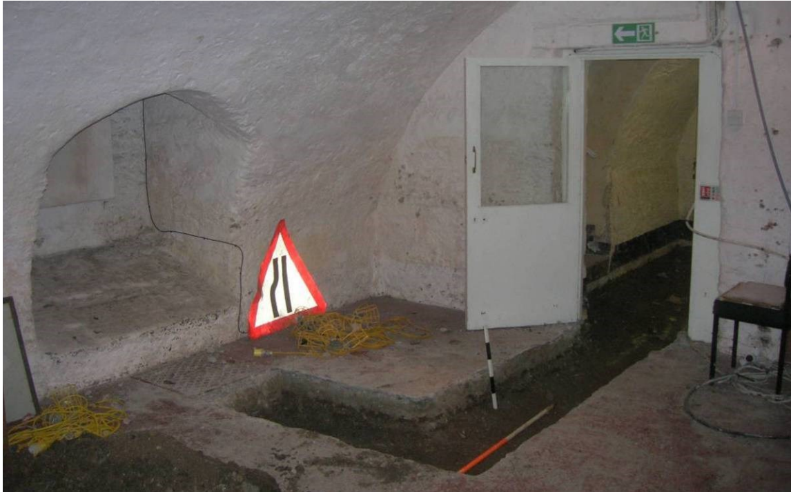
Fig 38 Excavation for new drains in the undercroft revealed a pitched slate rubble structure seen following the line of the far edge of the trench from the door opening in the partition wall and dog-legging to the front wall of the building to the jamb of the recess opening
