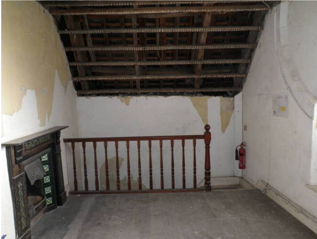
Fig 55 The upper floor room, showing a late 19 th century fireplace feeding into a flue cut into the face of the cross wall
