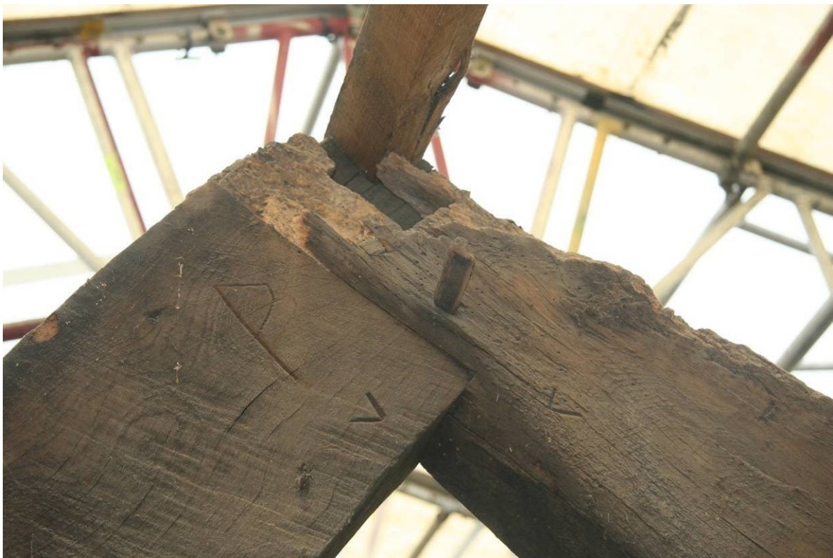
Fig 64 Example of a pegged apex joint on the 17 th century roof Carpenters marks are also clearly visible
