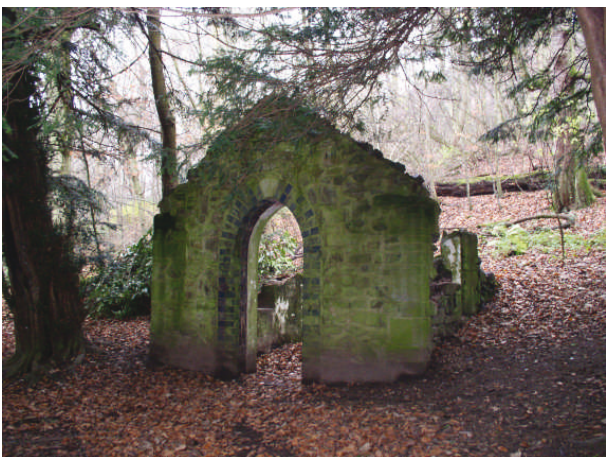
Site 10: the pumphouse
