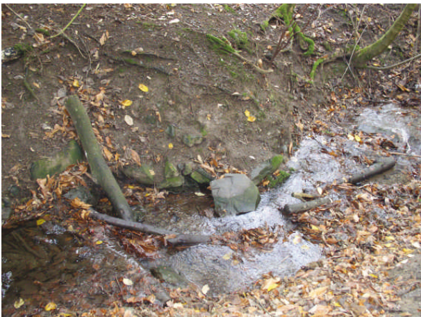
Site 6: footbridge abutment in the Townbrook
