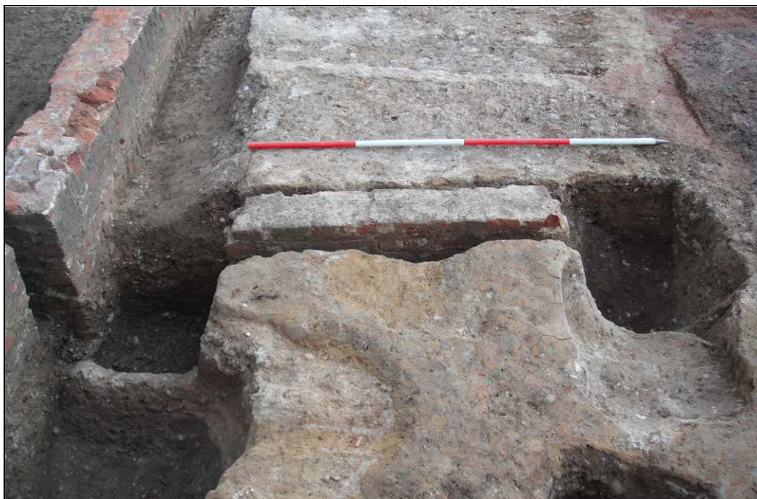
Plate 7: Phase 4d wall [230] with Phase 4e robber pits – looking east, 2m scale
