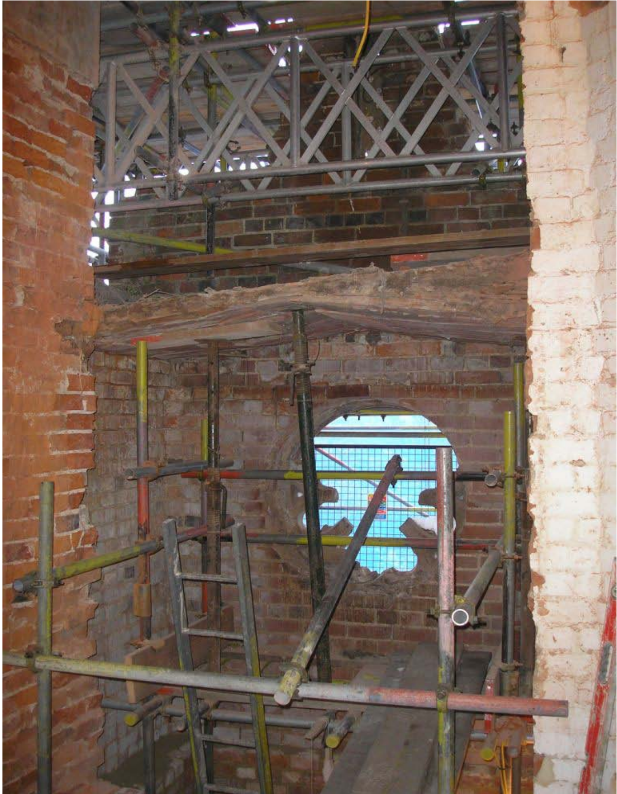
Plate 3. The recorded roof viewed from inside main tower, looking south.
