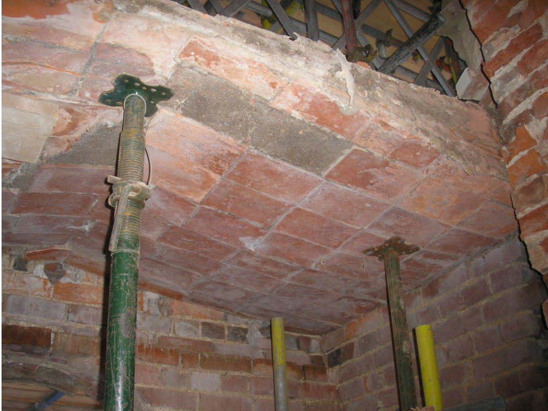
Plate 4. Peg tiles on the underside of the roof, looking southwest.
