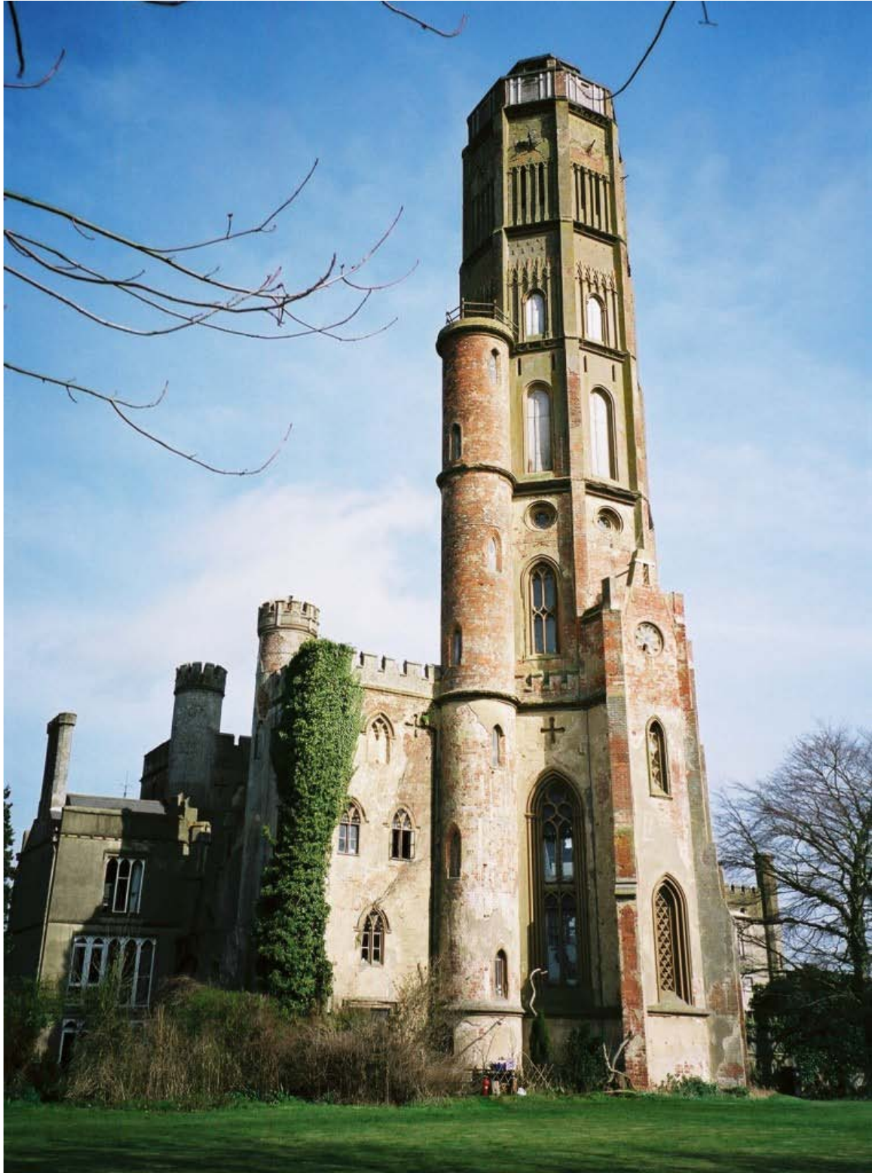
Plate 2. Hadlow Tower looking northeast.
