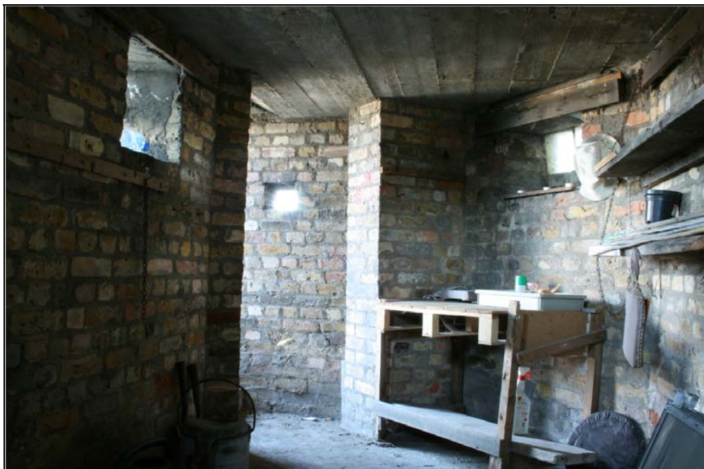
Plate 25 View of interior of pillbox, Building 6: OL-01907, looking north-west
