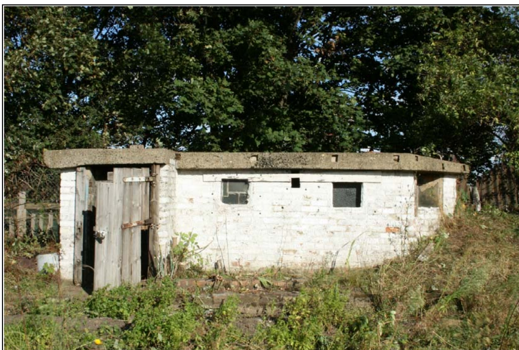
Plate 23 View of pillbox, Building 6: OL-01907, looking east
