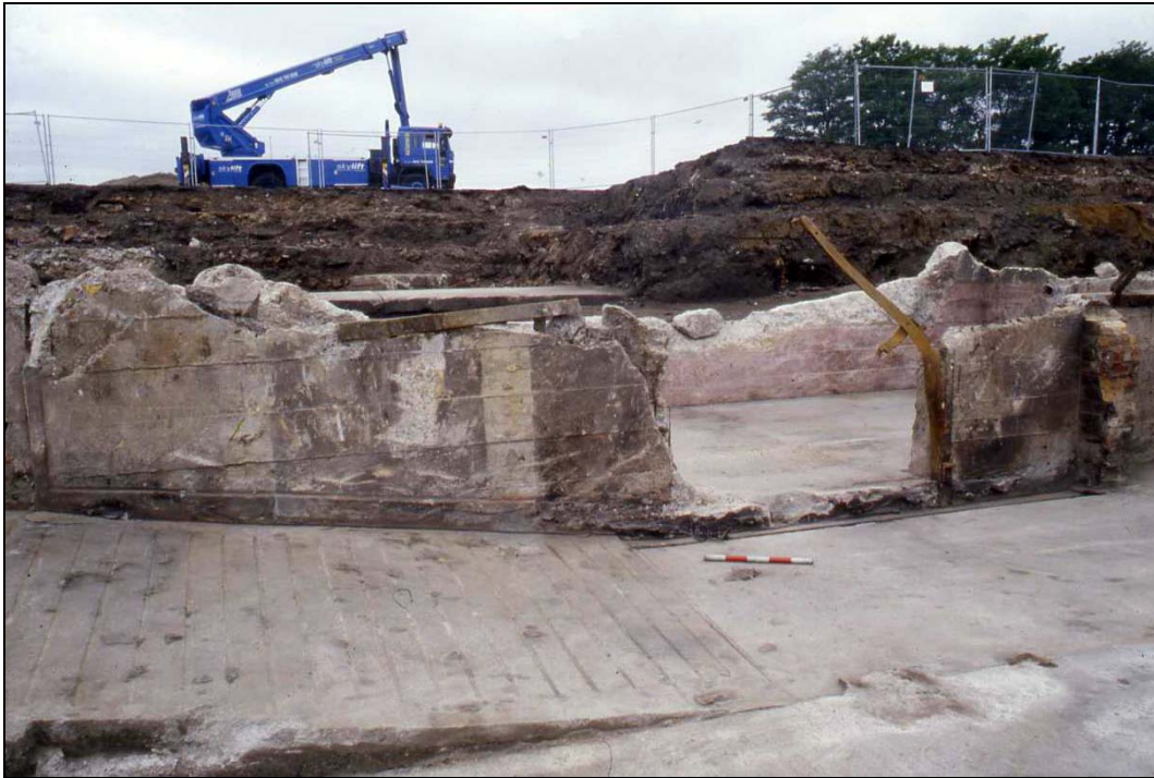
Plate 14 View of walkway and cordite store, Building 3: OL-01907, looking west
