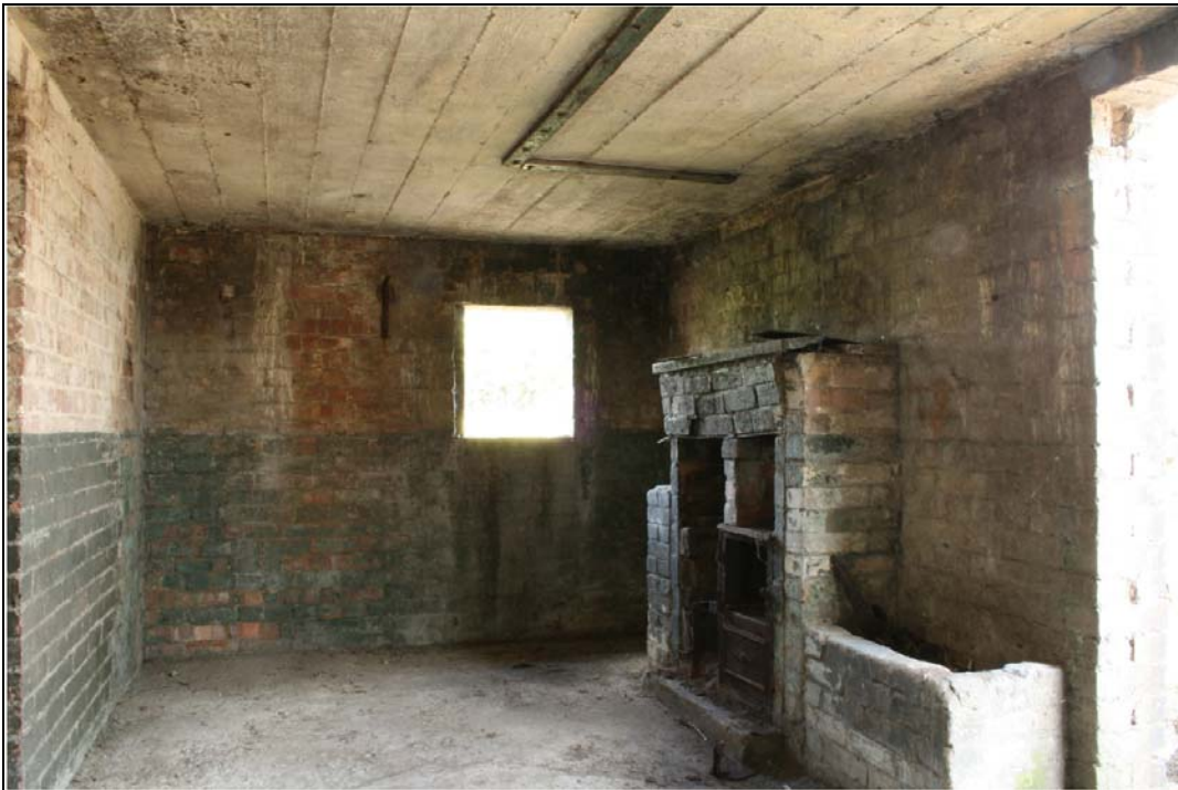
Plate 37 Internal view of G1, radar station, Building 10: OL-01907, looking north-east
