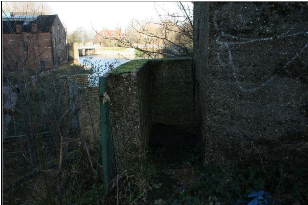
Plate 39 View of pillbox, Building 11, with Old Ford Lock in background: OL-08007, looking north
