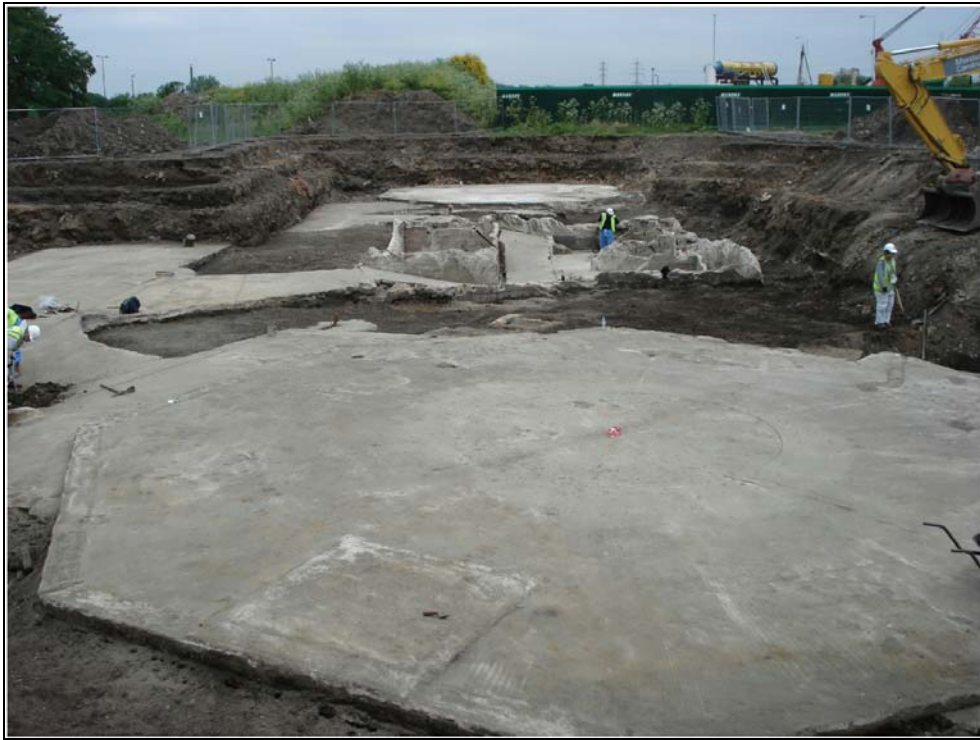
Plate 17 View of south gun platform, Building 4: OL-01907, looking north
