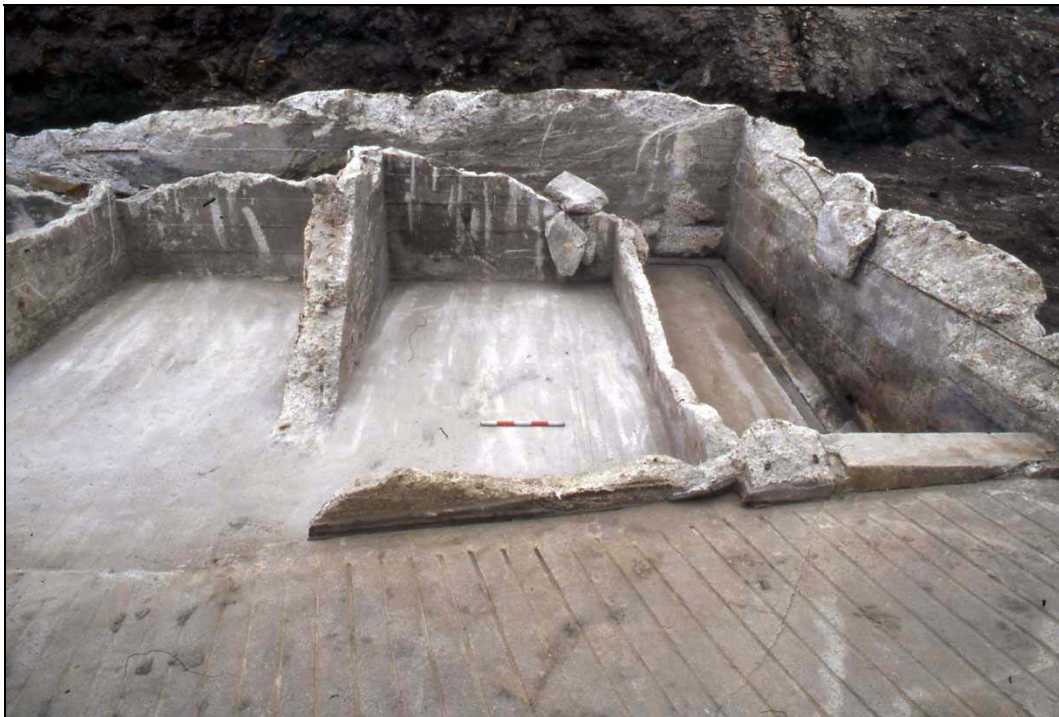
Plate 12 View of bays within magazine, Building 2: OL-01907, looking east
