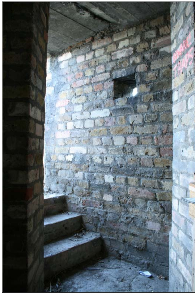
Plate 24 View of doorway from within pillbox, Building 6: OL-01907, looking north-west
