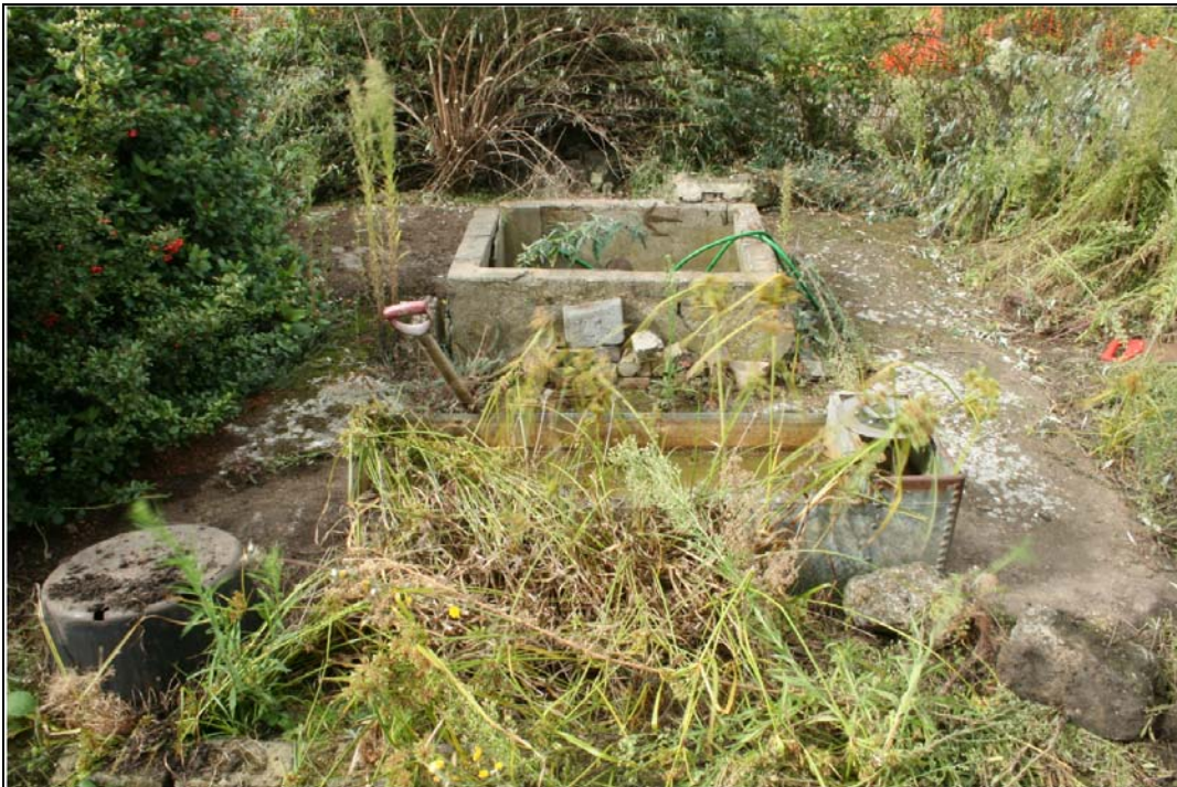
Plate 32 View of wind driven pump: OL-01907, looking west
