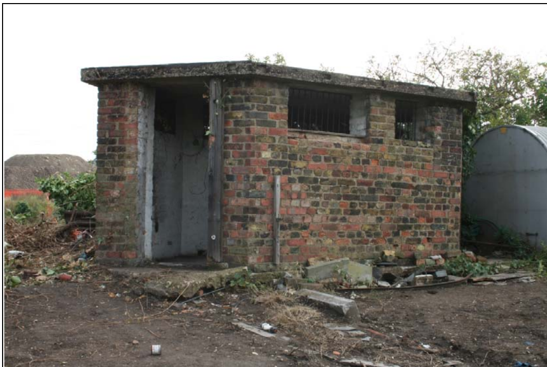
Plate 27 View of pillbox, Building 7: OL-01907, looking east
