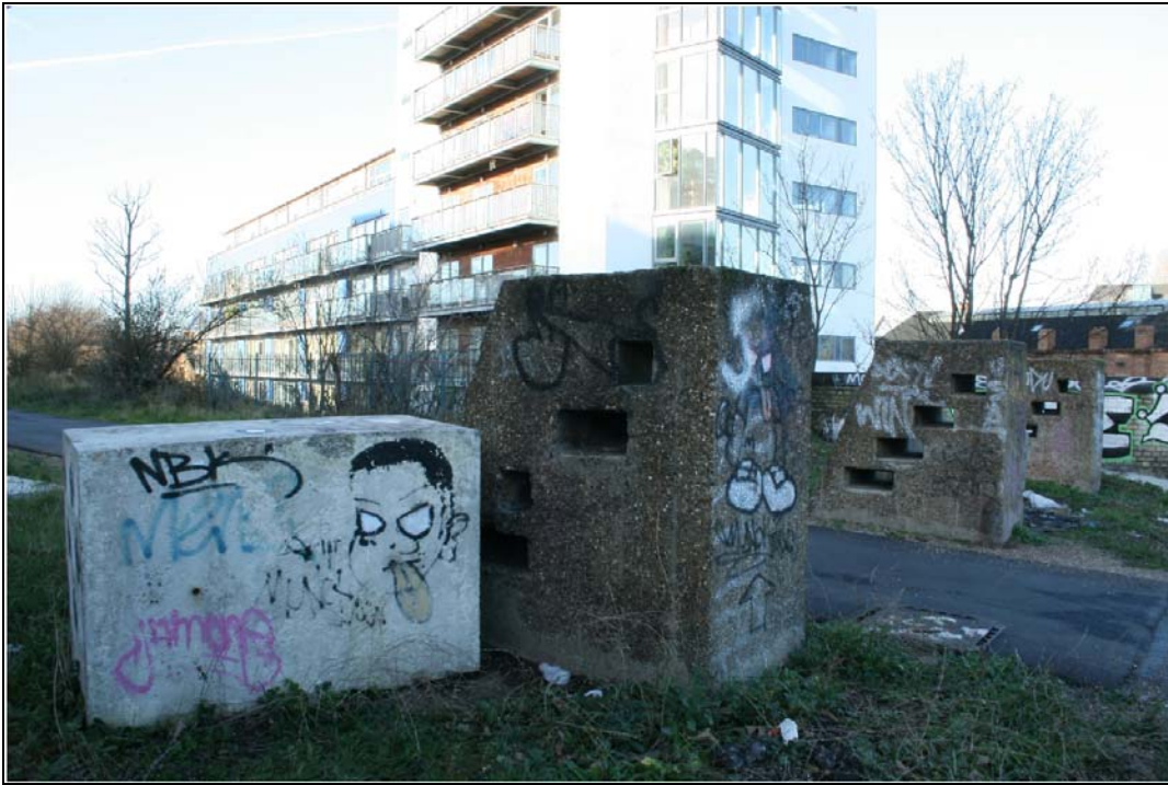
Plate 42 View of tank traps, Building 12: OL-08007, looking north-west
