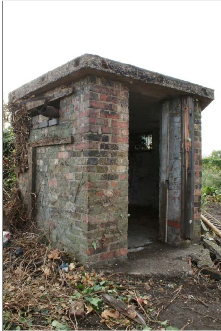
Plate 28 View of pillbox, Building 7: Ol-01907, looking south-east
