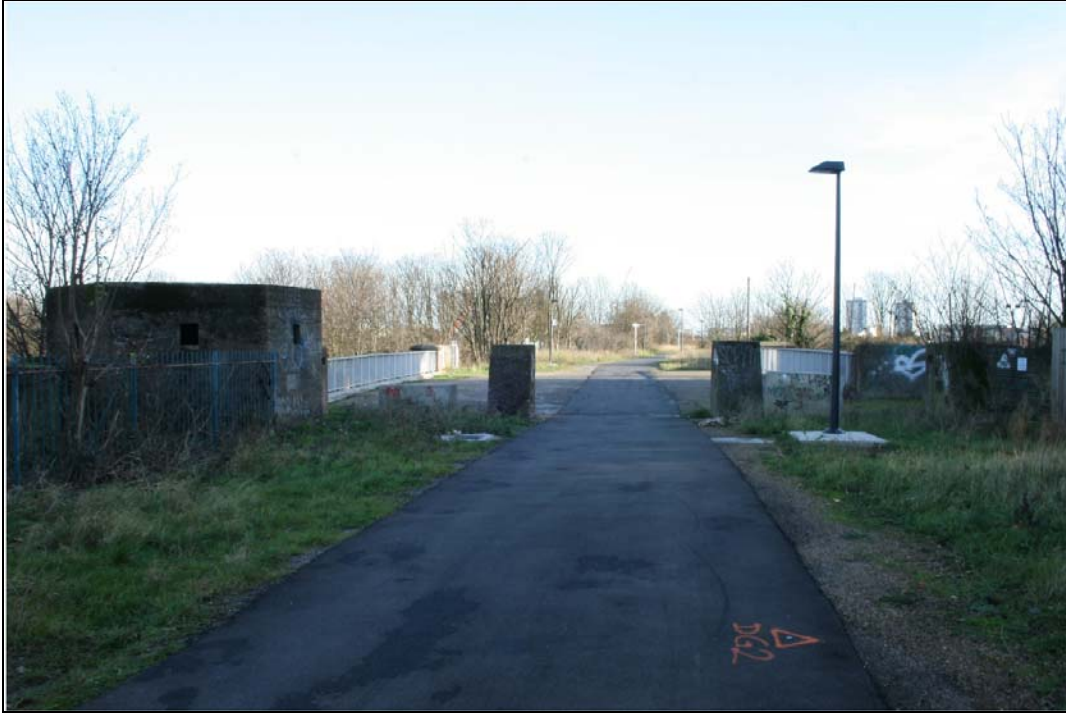
Plate 41 View of pillbox and tank traps, Buildings 11 and 12, showing location: OL-08007, looking east
