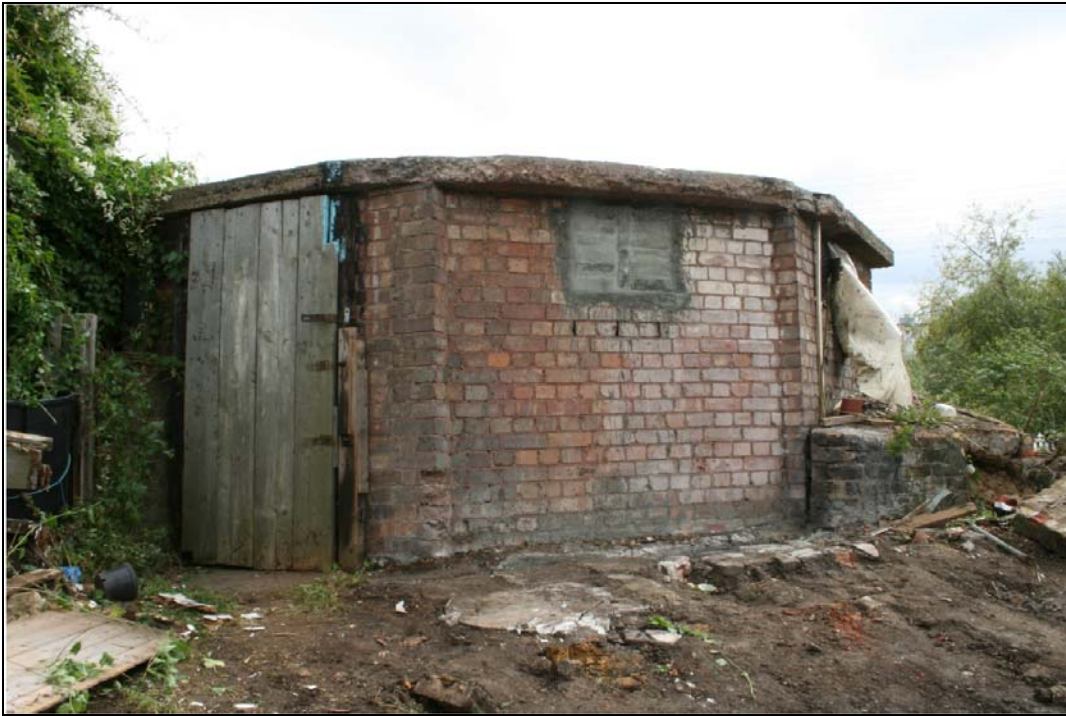
Plate 30 View of pillbox, Building 8: OL-01907, looking south-east
