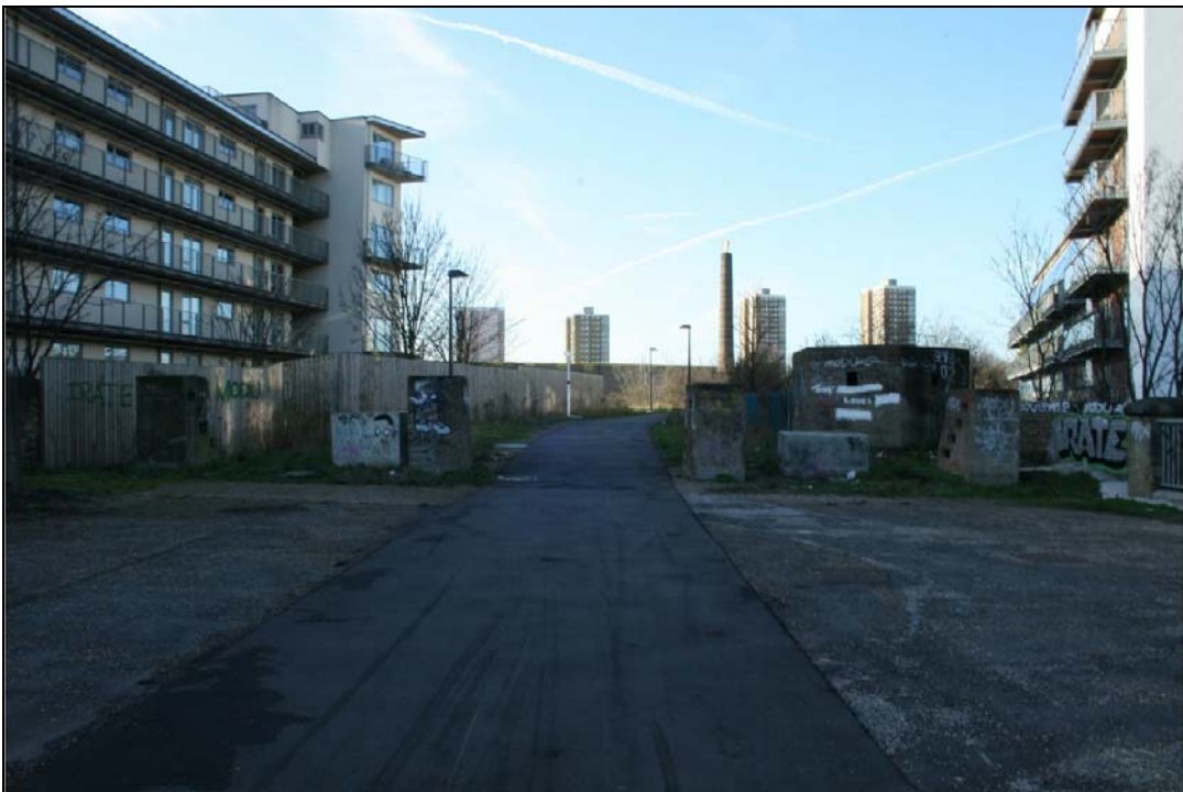
Plate 9 View of pillbox and tank traps, Buildings 11 and 12: OL-08007, looking west
