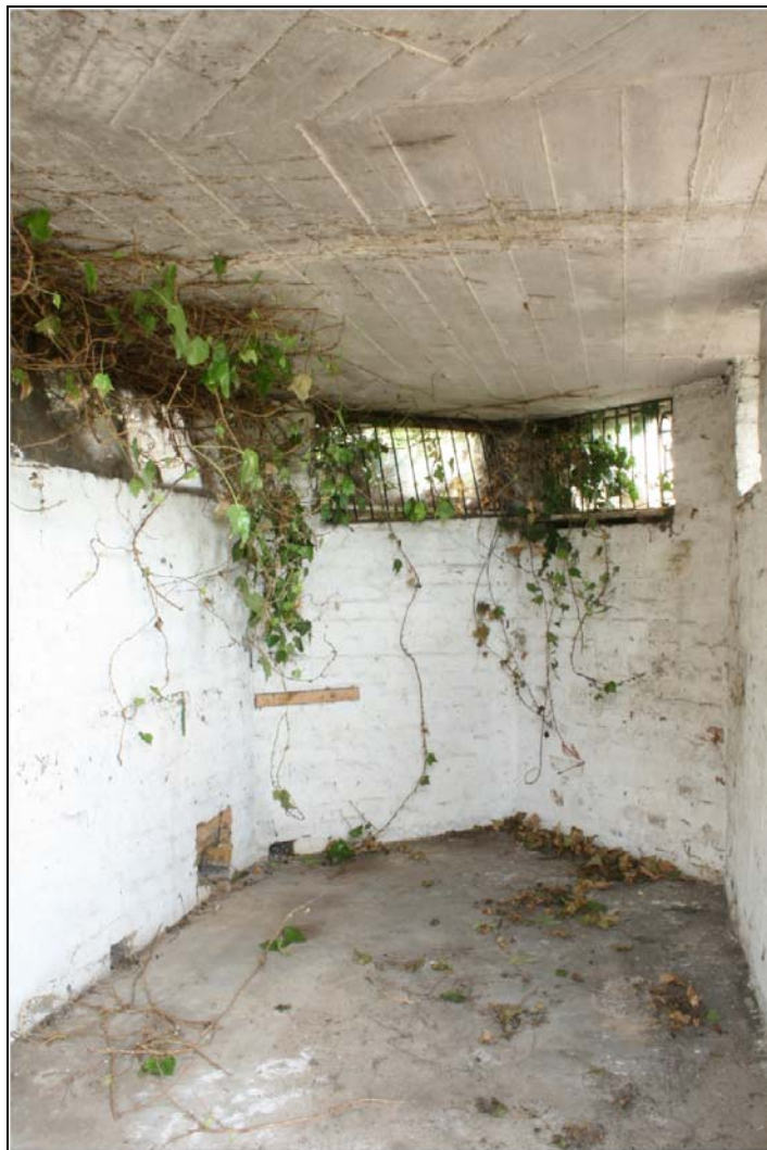
Plate 26 View of interior of pillbox, Building 7: OL-01907, looking south
