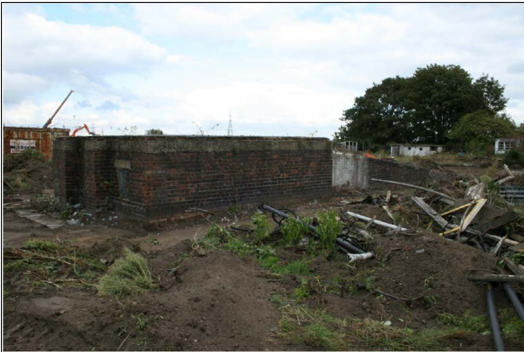
Plate 34 View of rear of radar station, Building 10, with pillbox, Building 6 in the background: OL-01907, looking north-east
