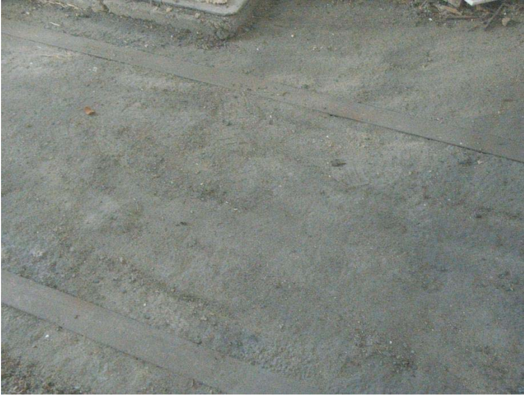
Plate 29: Culross Building filler joist floor with concrete laid between RSJs
