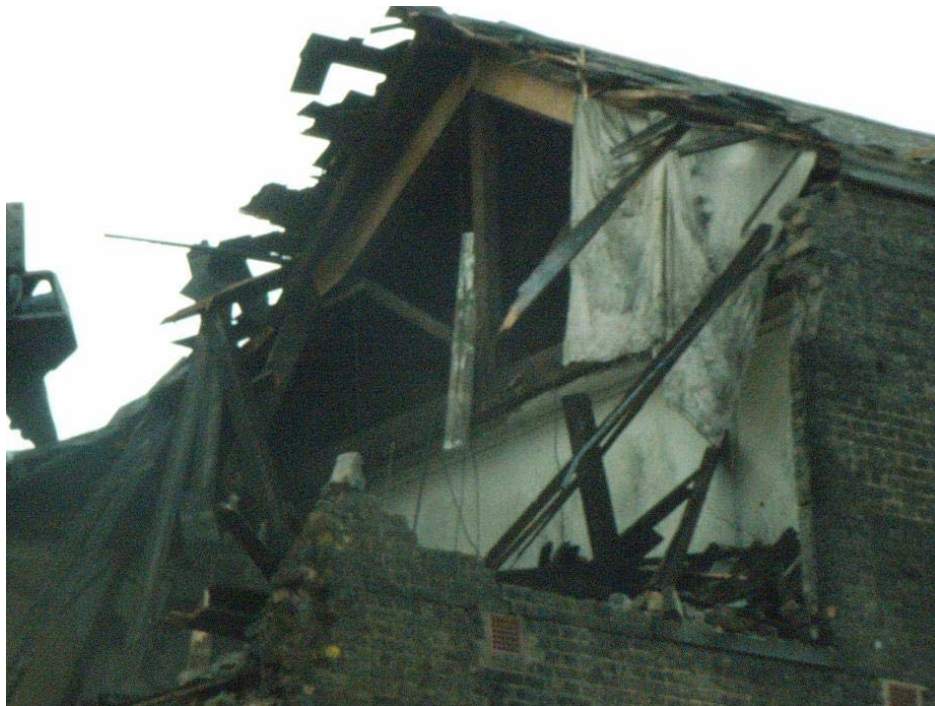
Plate 46: Roof truss of Culross Hall (looking north) exposed during demolition
