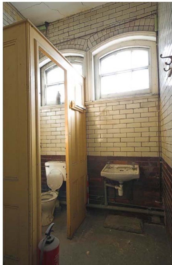
Plate 62: Timber partition in Toilet CH1E (Figure 15), Culross Hall
