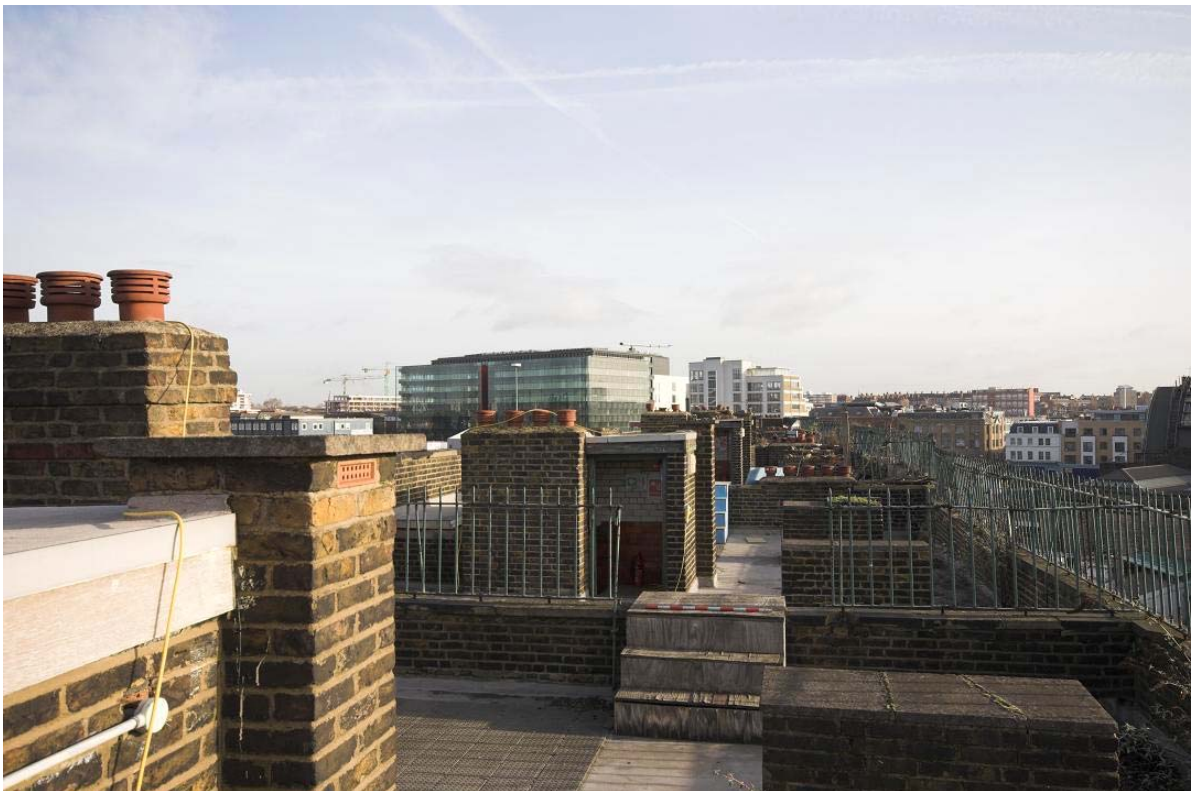
Plate 16: Roof of Culross Building (viewed from the south-west)
