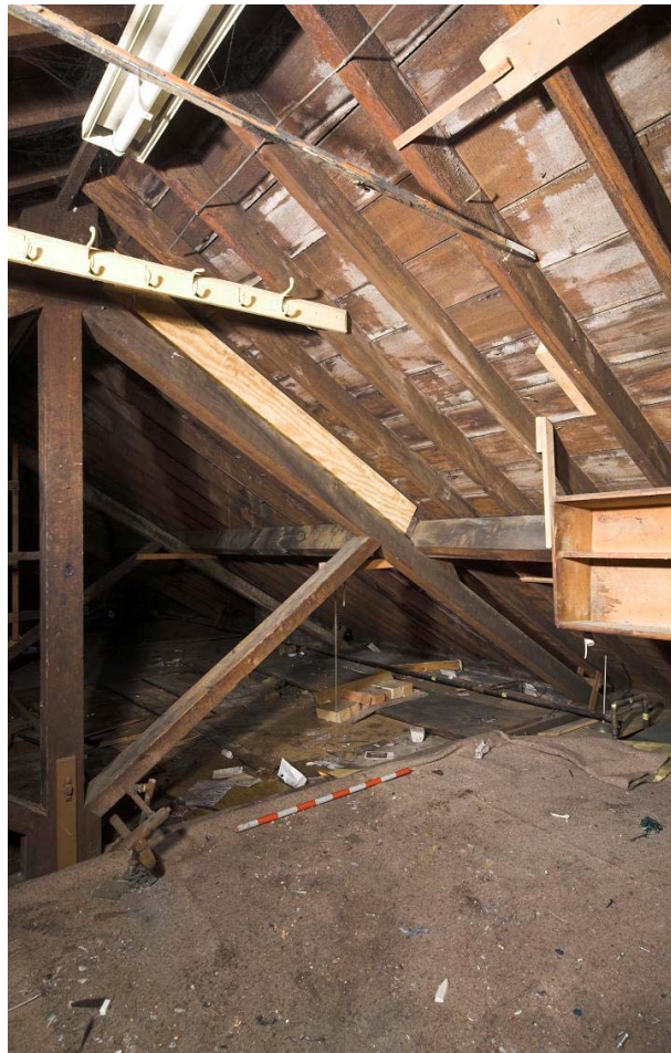
Plate 64: Attic of Culross Hall
