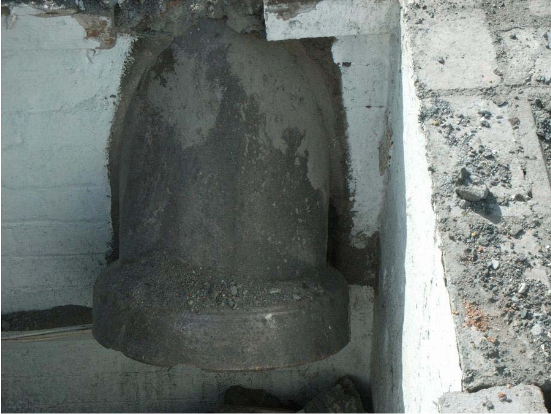
Plate 27: Foot of ash chute in Culross Building
