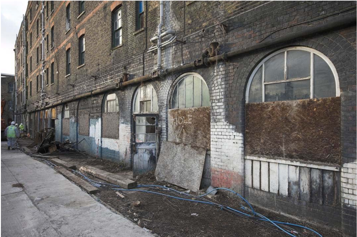
Plate 5: Rear (south-east) elevation of Culross Building
