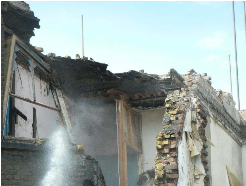
Plate 66: Roof structure of No. 41 Battle Bridge Road exposed during demolition
