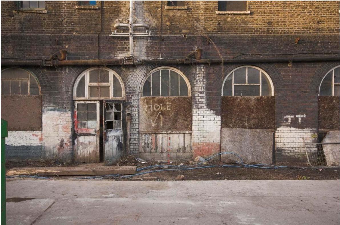
Plate 15: Rear (south-east) elevation of the basement of the Culross Building
