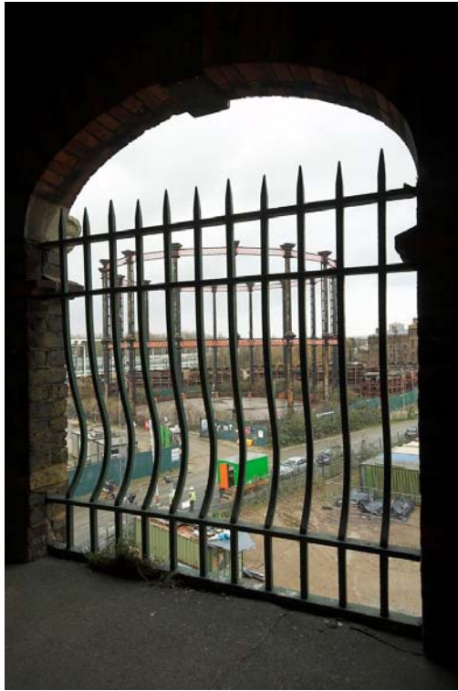
Plate 11: Iron railings in a stairwell of the Culross Building
