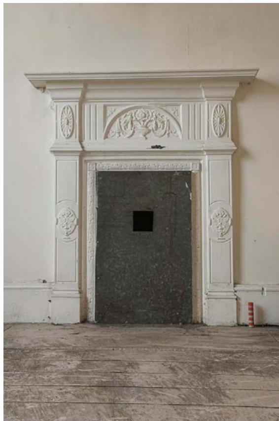
Plate 34: Cast iron fireplace (Figure 35) in Bedroom CB16F (Figure 17) in Culross Building
