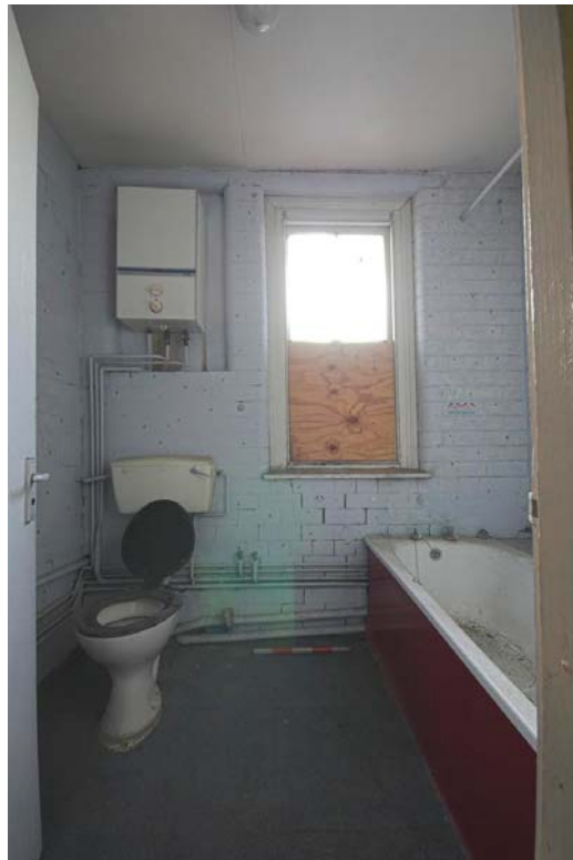
Plate 30: Bathroom CB7B (Figure 17) in Culross Building with blocked window behind water heater
