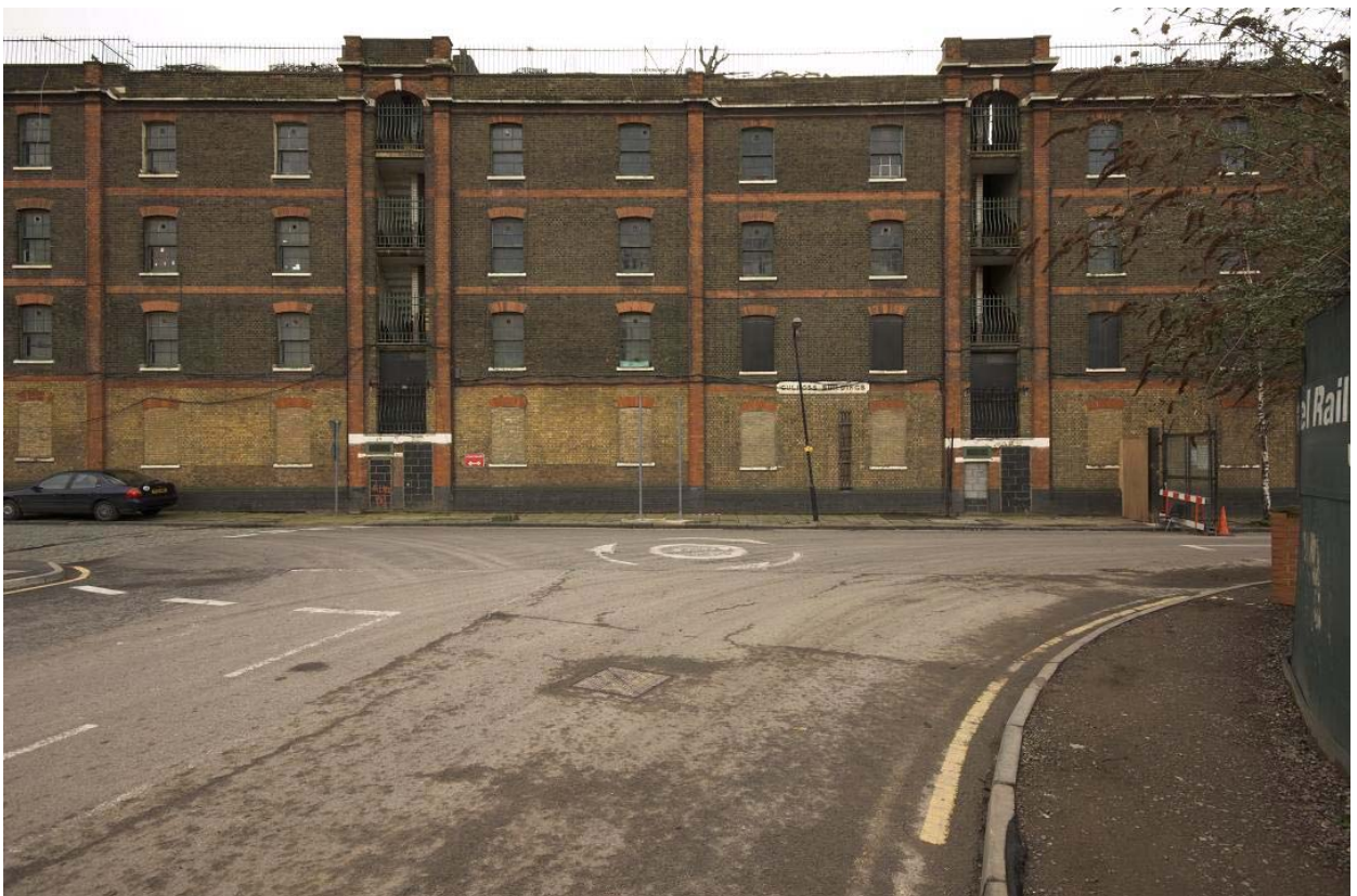
Plate 2: Front (north-west) elevation of the Culross Building
