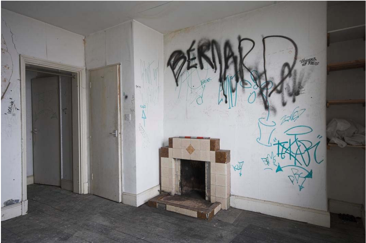
Plate 37: Living Room CB40D (Figure 17) in Culross Building with some original skirting board and architrave and 1930s or 1950s fireplace surround
