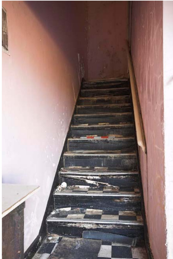
Plate 71: Stair CB41B leading to first floor of No. 41 Battle Bridge Road
