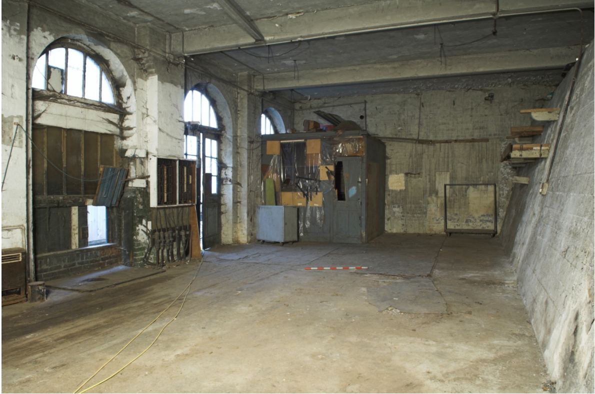
Plate 51: Basement Room CBB1 below Culross Hall viewed from the east
