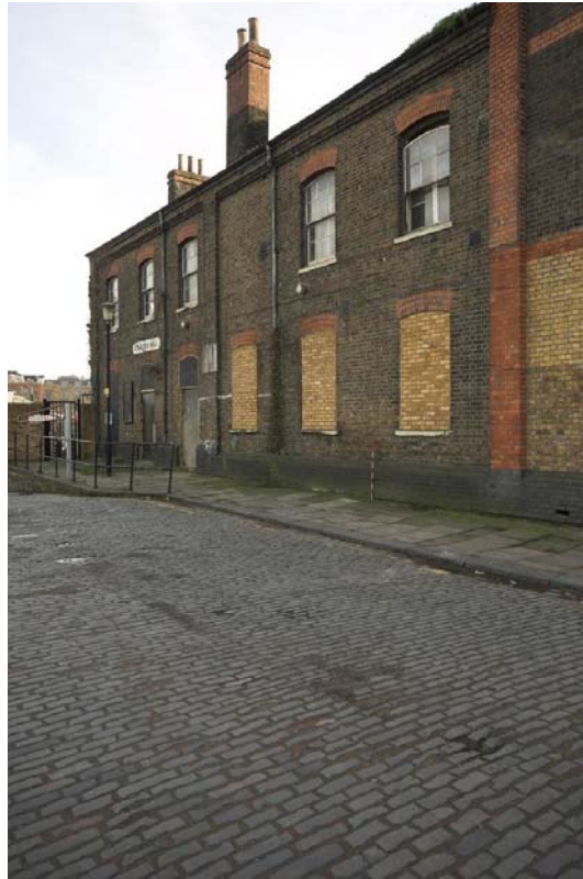
Plate 3: Front (north-west) elevation of Culross Hall
