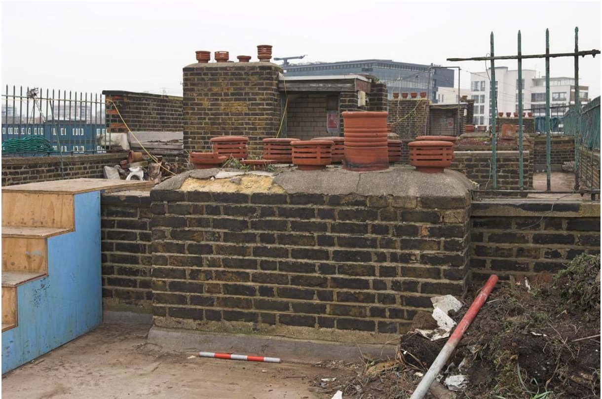
Plate 23: Chimney stack on roof of Culross Building
