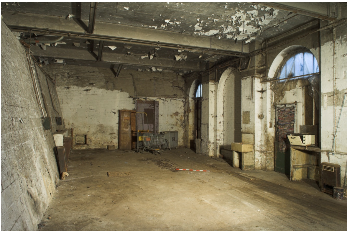
Plate 50: Basement Room CBB1 below Culross Hall viewed from the west
