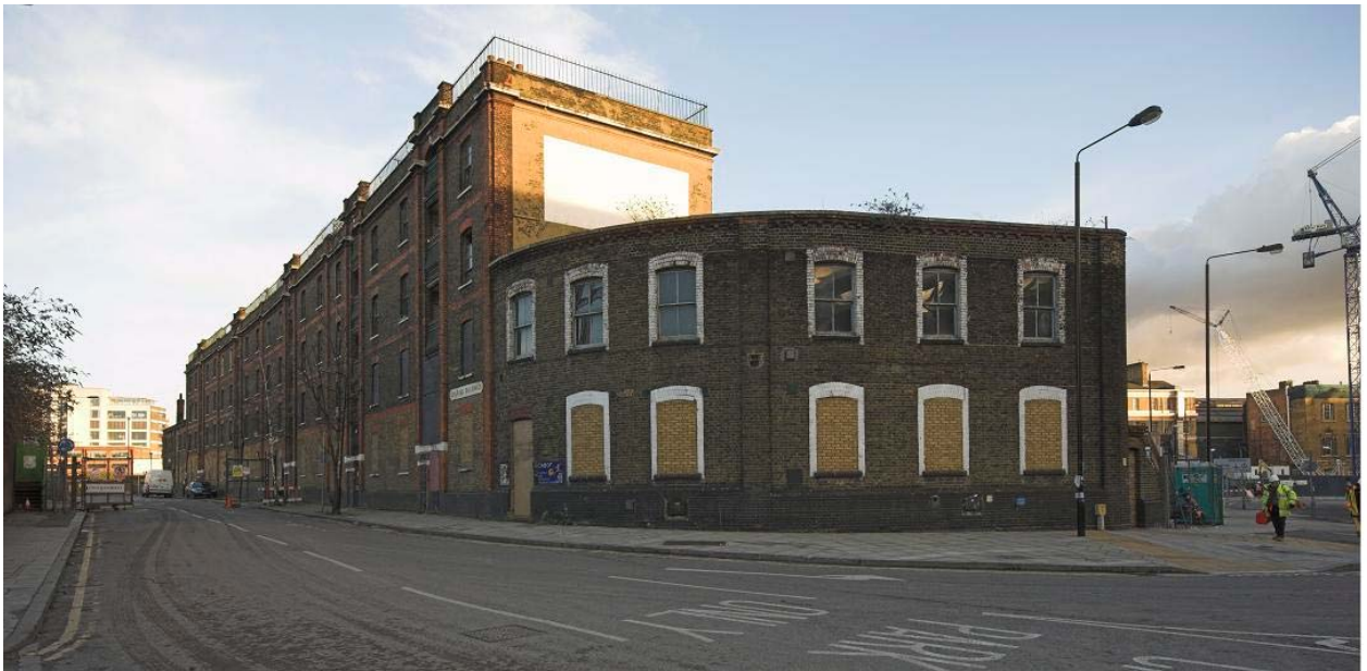
Plate 1: Front (north-west and south-west) elevations of the Culross Buildings with Culross Hall to the north-east (far left), Culross Building (left) and No. 41 Battle Bridge Road to the south-west (right)
