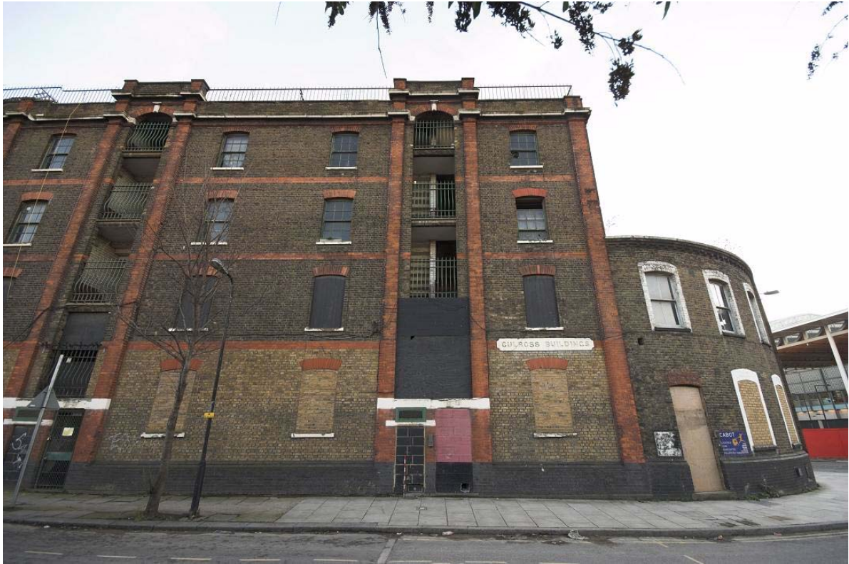
Plate 7: South-west end of the front (north-west) elevation of the Culross Building
