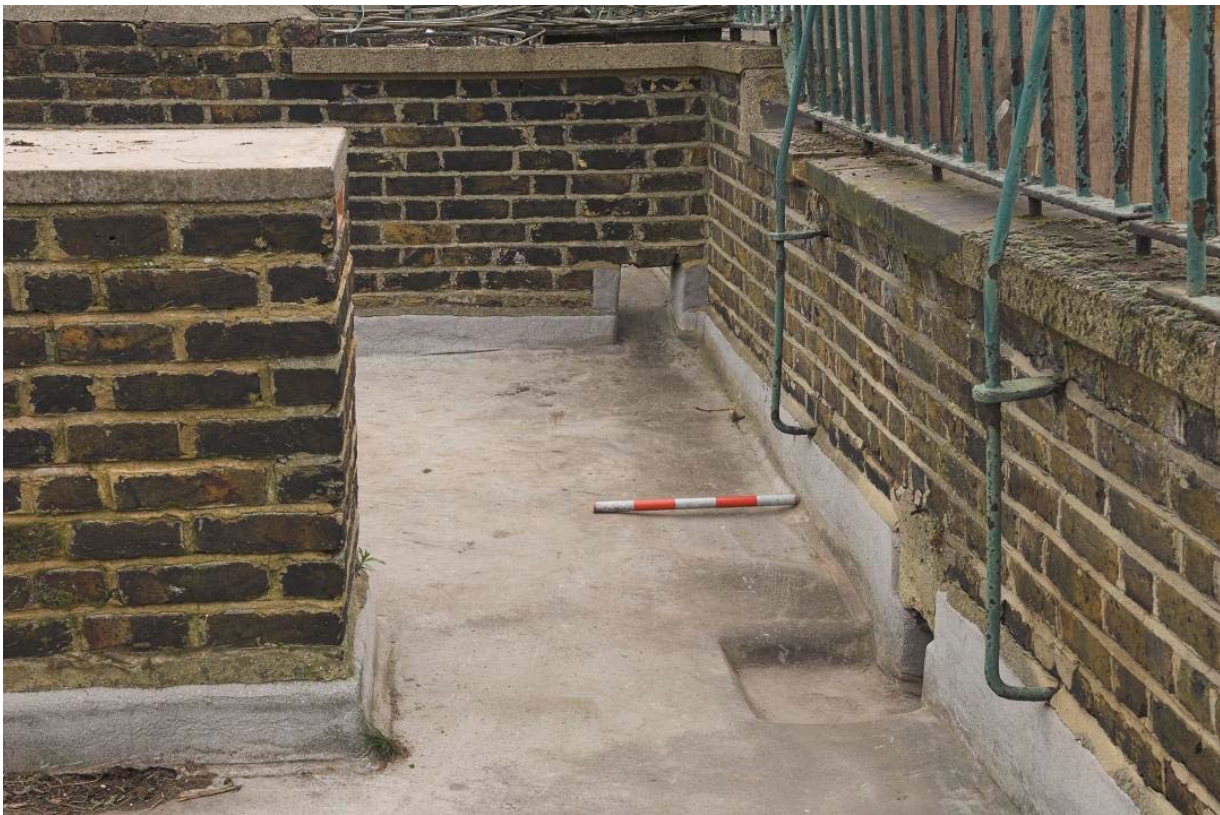
Plate 24: Drainage hole in roof of Culross Building
