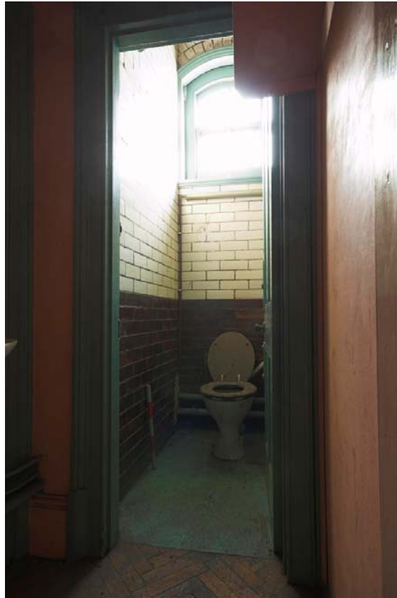
Plate 61: White and brown glazed brick walls of Toilet CH1D (Figure 15), Culross Hall
