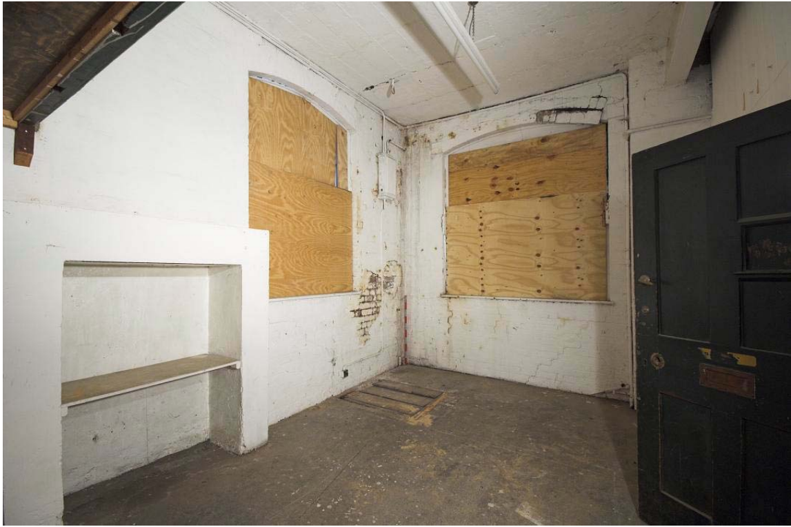
Plate 53: Hatch in floor of Room CHGD (Figure 14), Culross Hall, leading to basement
