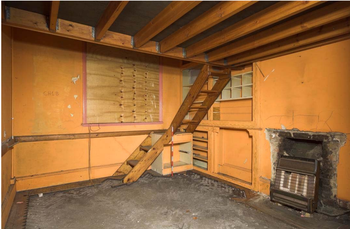
Plate 63: Room CH1B, Culross Hall, with stairs against north-west wall
