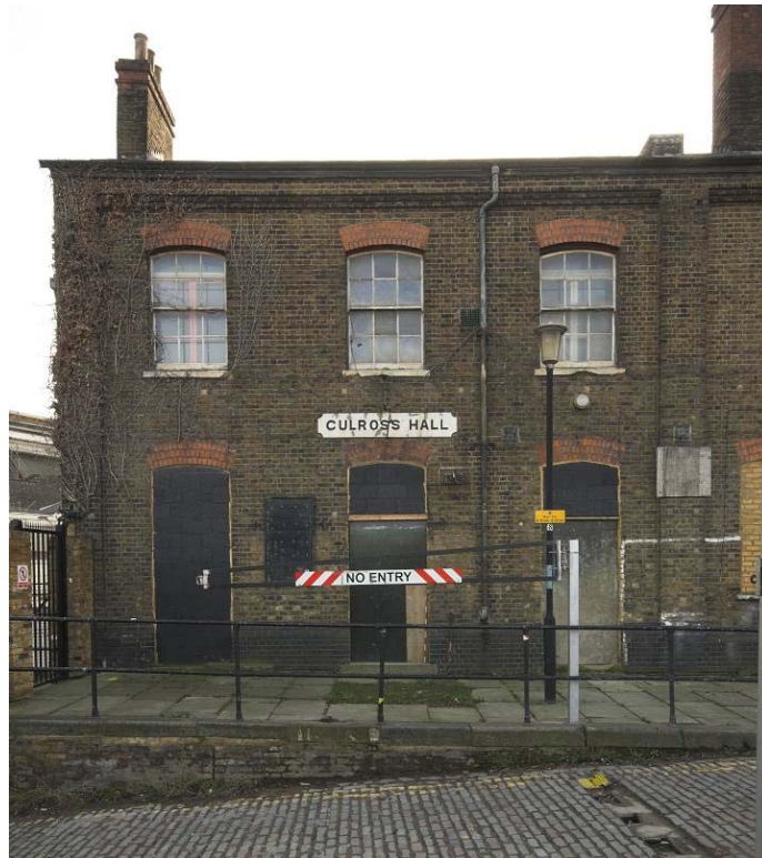
Plate 47: North-east end of front (north-west) elevation of Culross Hall
