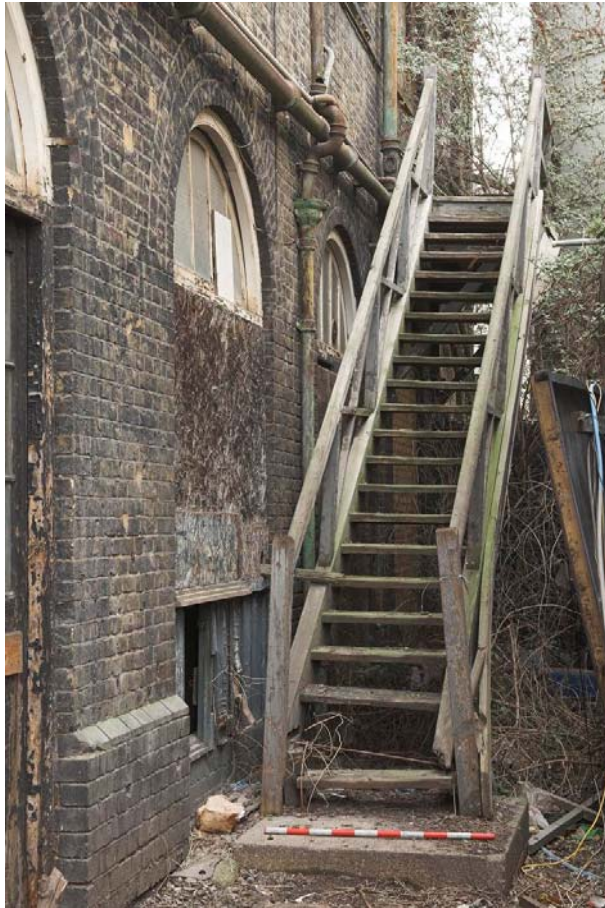
Plate 49: Timber staircase on rear (south-east) elevation of Culross Hall
