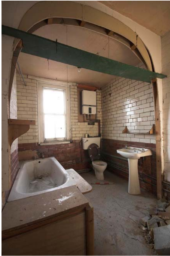
Plate 33: Glazed brick walls in Bathroom CB8B (Figure 17) in Culross Building
