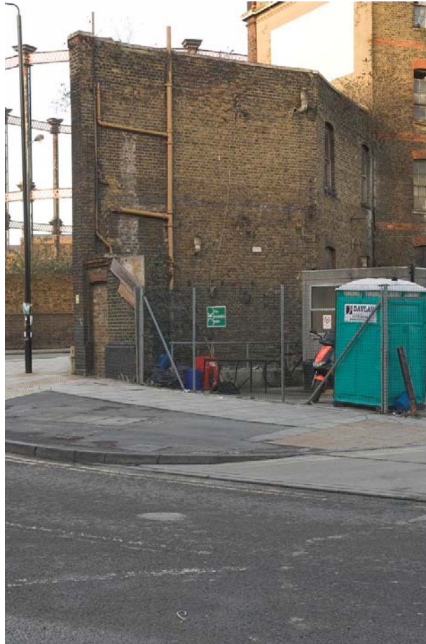
Plate 67: South-east elevation of No. 41 Battle Bridge Road
