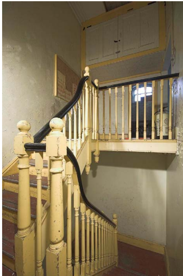
Plate 52: Timber staircase (CH1A) leading from ground to first floor, Culross Hall
