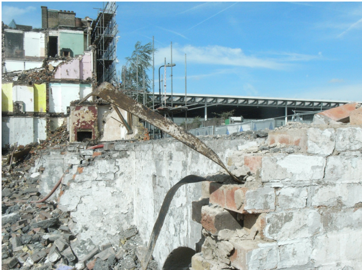
Plate 6: Hoop iron in a mortar joint within the brickwork of a basement dividing wall under the Culross Building, viewed from the east
