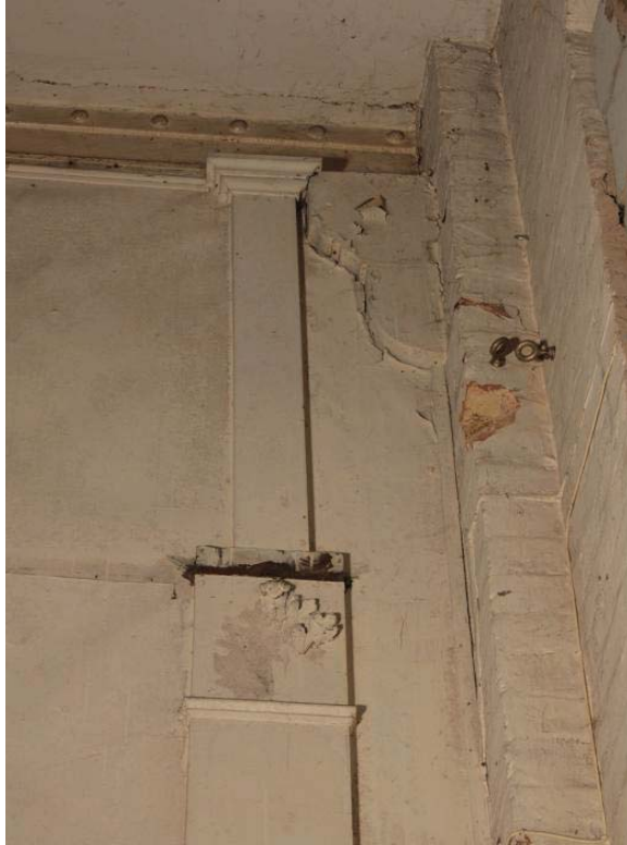
Plate 19. Detail of pilaster of stage façade showing classical mouldings and remnants of acanthus leaf embellishment to capital. Note the moulded corbel supporting a steel ceiling joist.
