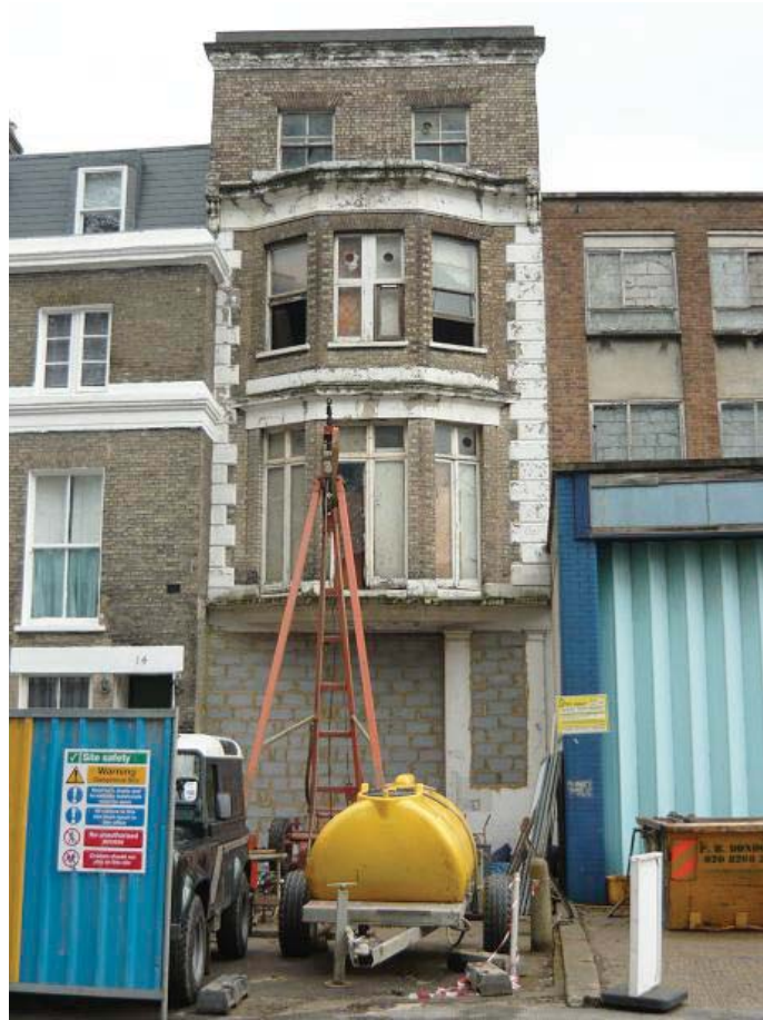
Plate 3. West elevation of 13 Paddington Green.
