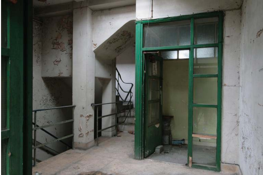
Plate 28. First floor landing F4, looking west.
