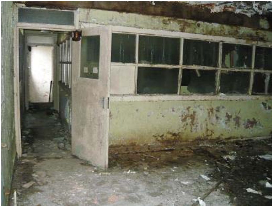
Plate 31. Second floor office S1 with glass partitions between offices.
