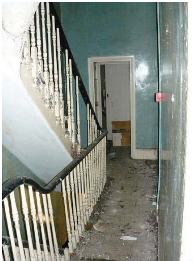
Plate 36. First floor landing 13 Paddington Green, looking west.
