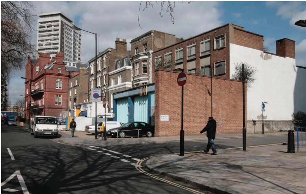
Plate 4. West and south elevations of 11-12 Paddington Green.
