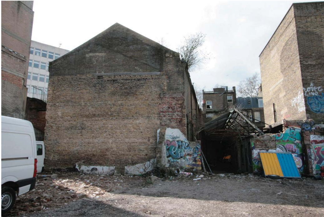
Plate 5. East/rear elevations of 11-13 Paddington Green.
