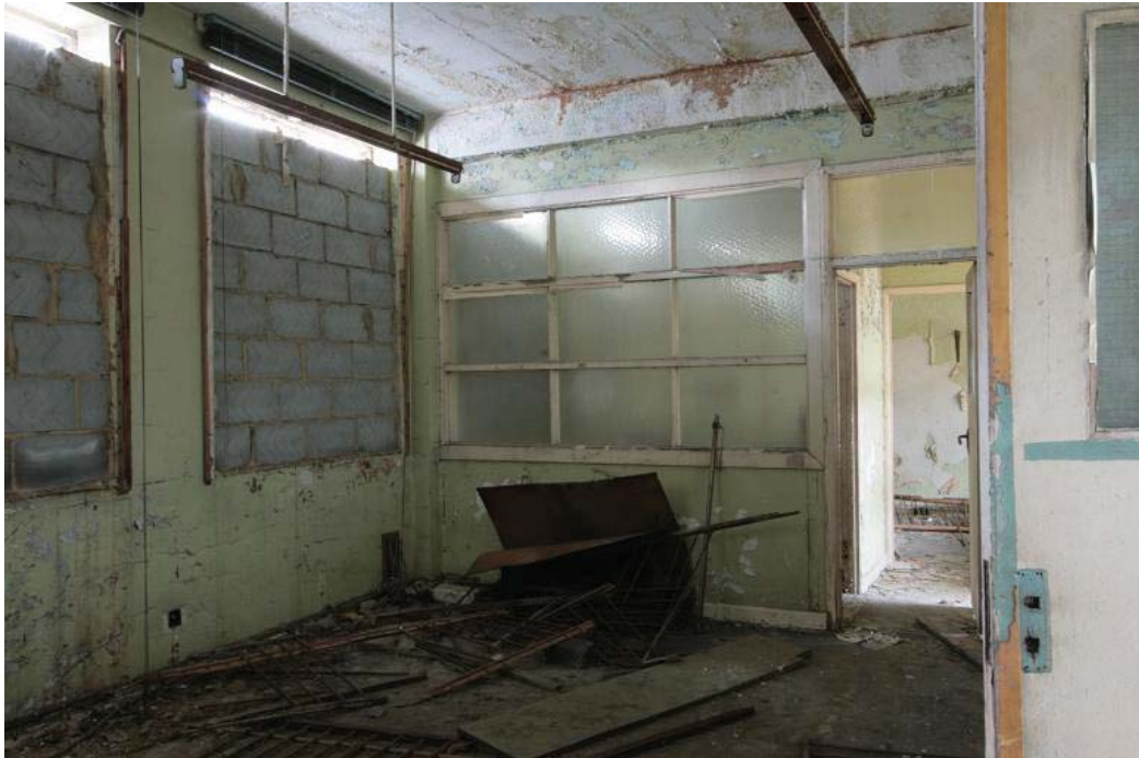
Plate 29. First floor office F9, looking north, with glass partition between offices.
