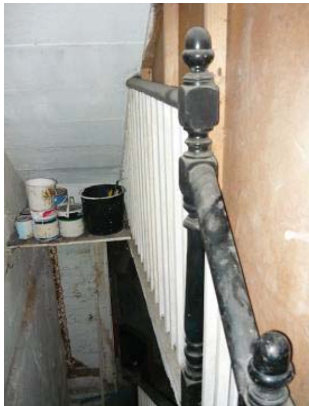
Plate 32. Decorative banister from ground floor to basement.
