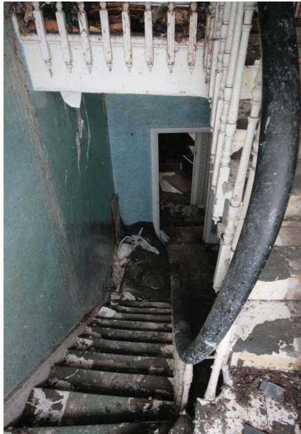
Plate 40. 13 Paddington Green curvilinear banister from third to second floor.
