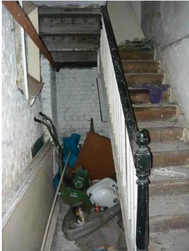
Plate 33. 13 Paddington Green basement looking east.
