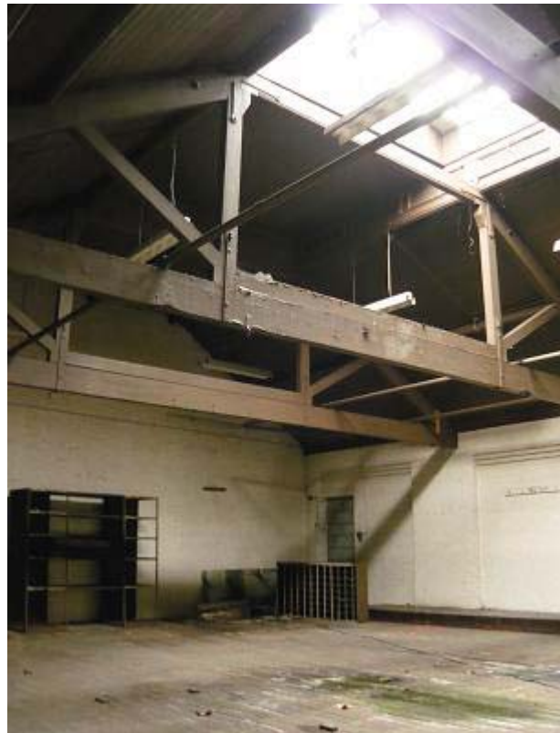
Plate 24. Detail of roof truss with skylight, first floor gymnasium.
