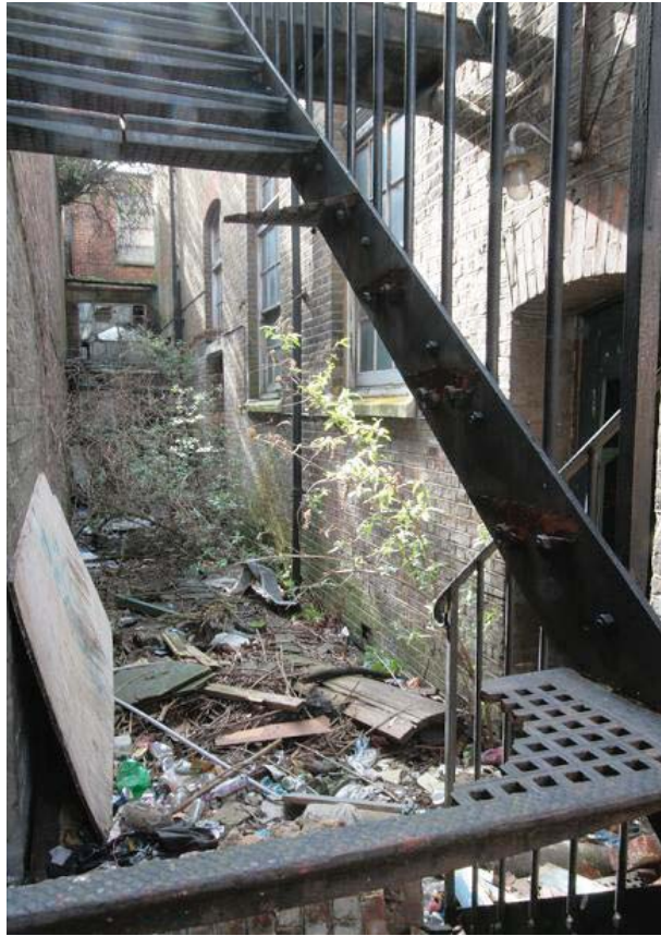
Plate 9. South elevation of theatre to rear of 11-12 Paddington Green, looking west.
