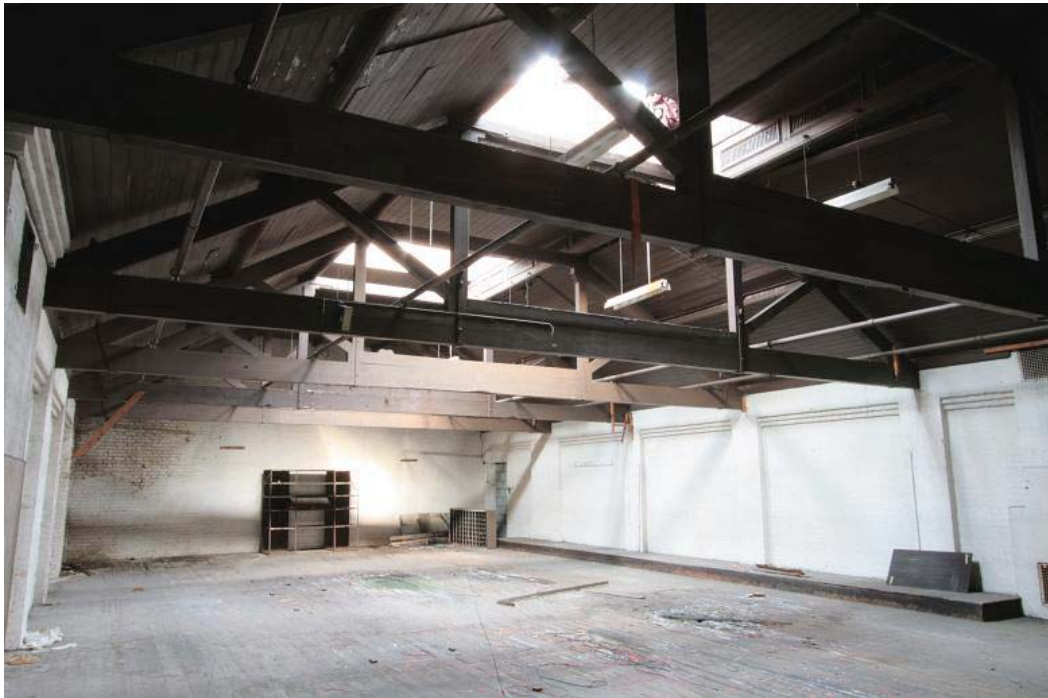
Plate 23. First floor gymnasium above theatre, looking south east.
