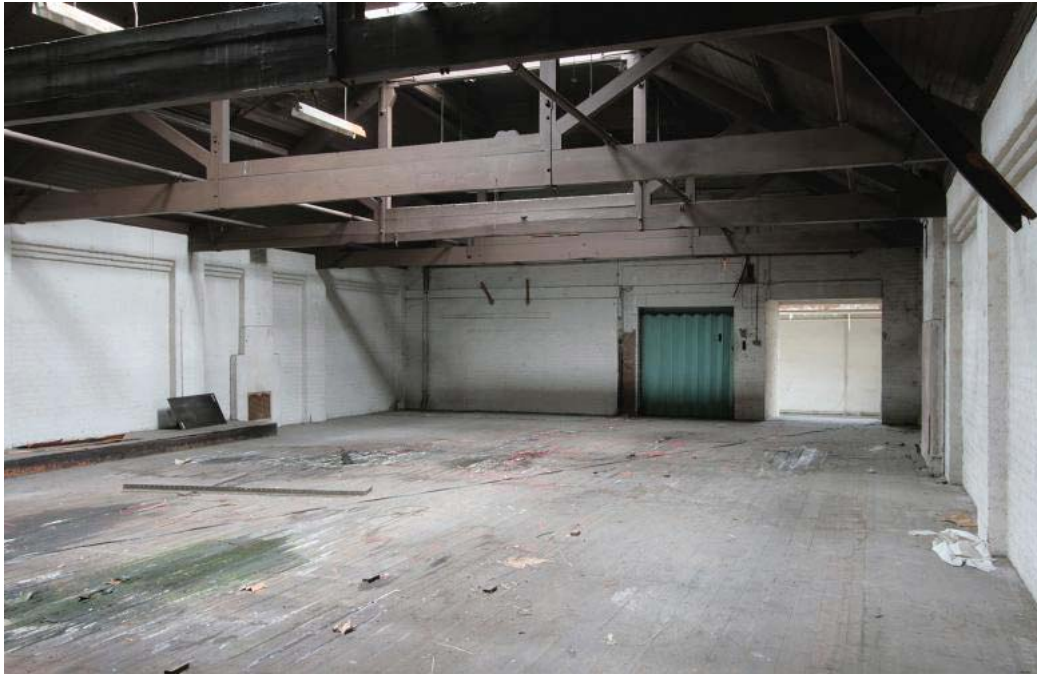
Plate 25. First floor gymnasium above theatre, looking south west.
