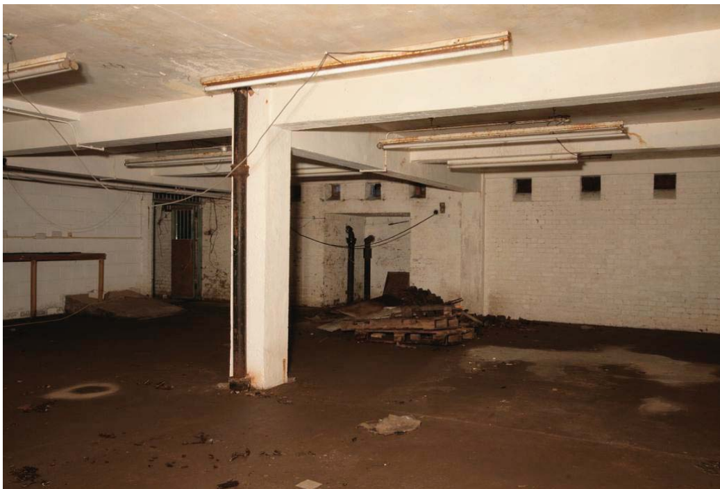
Plate 14. Basement of 11-12 Paddington Green looking south west.
