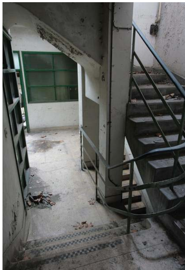
Plate 30. View of first floor landing F4, from stairs to second floor.
