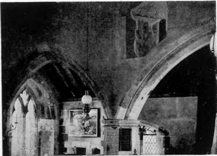
2. COCKING CHURCH : SOUTH AISLE AND ARCADE, WITH NORMAN WINDOW OVER.
