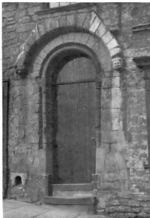
b. LINCOLN : 'AARON THE JEW'S HOUSE', DOORWAY IN W. FRONT, 1946 (p. 160)
