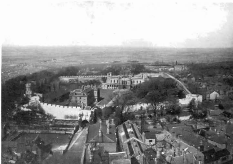
a. LINCOLN CASTLE : VIEW FROM THE EAST TAKEN FROM THE NW. TOWER OF THE CATHEDRAL, 1947 ; COMPARE THE PLAN FIG. 1, p. 157
