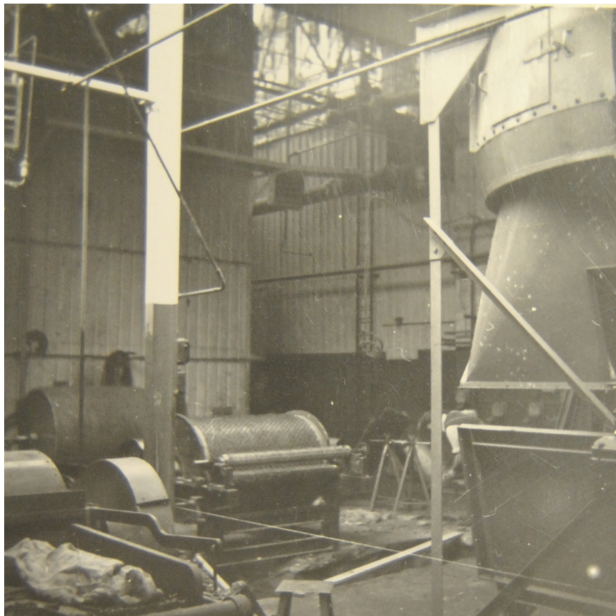
(b) 'New Centriblender being erected, 1953'; same location.
