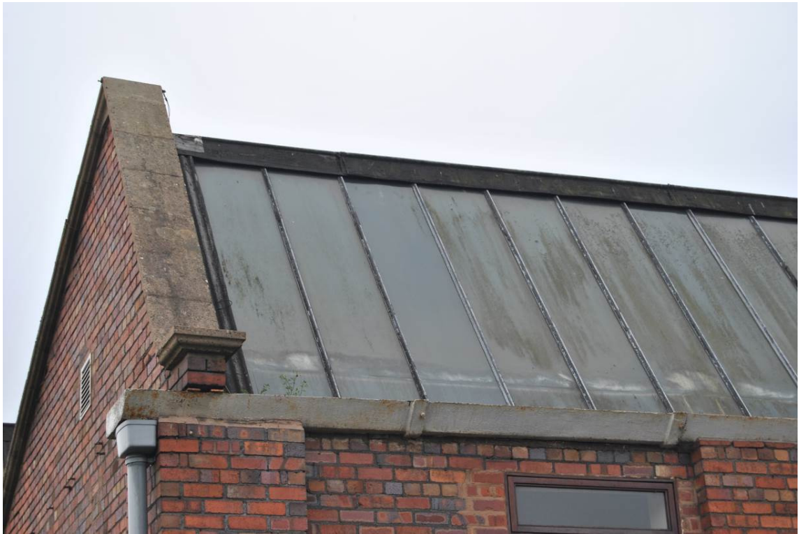
Plate 12: Detail of glazed north-light roof.
