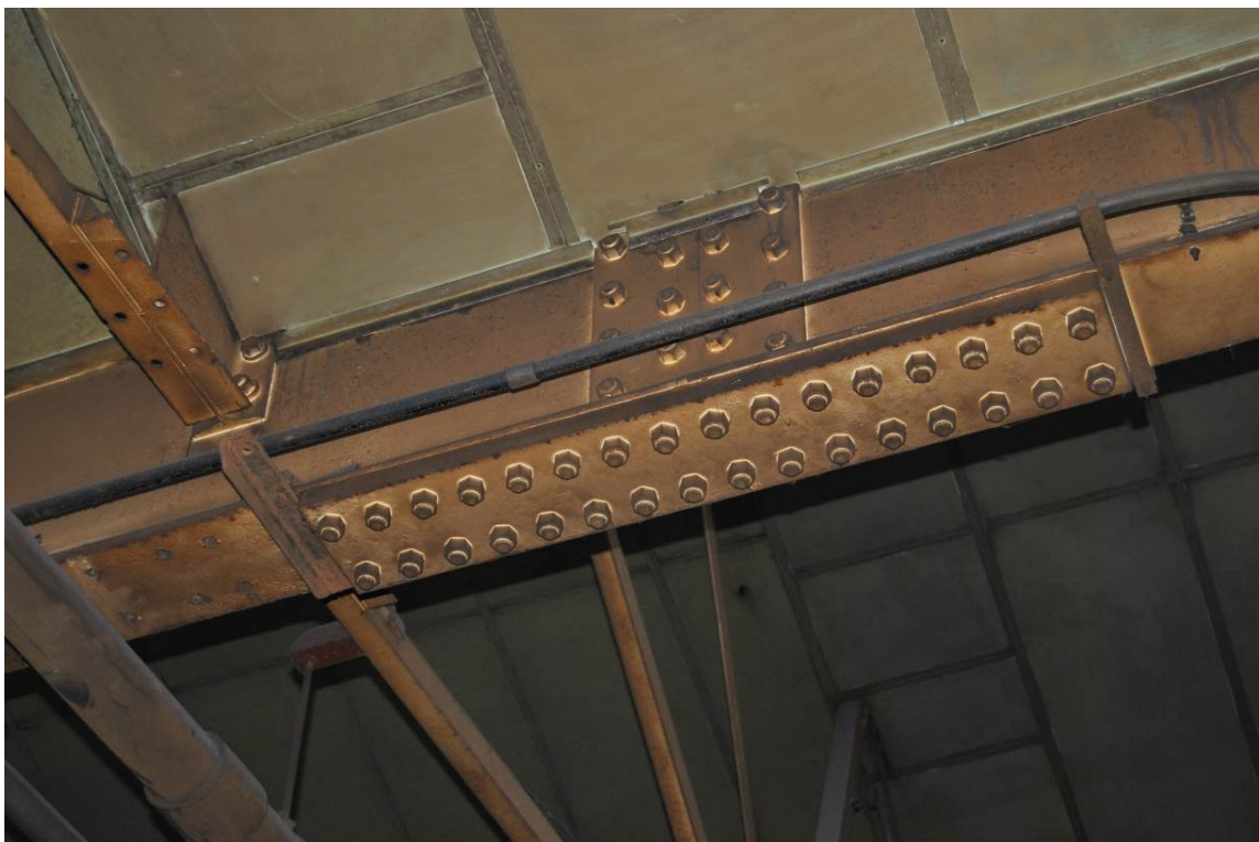
Plate 33: Jointed valley beam evidencing junction of Phase III (pre-1955) and Phase V (pre-1969) westwards extension of 'Zone C' spinning sheds.
