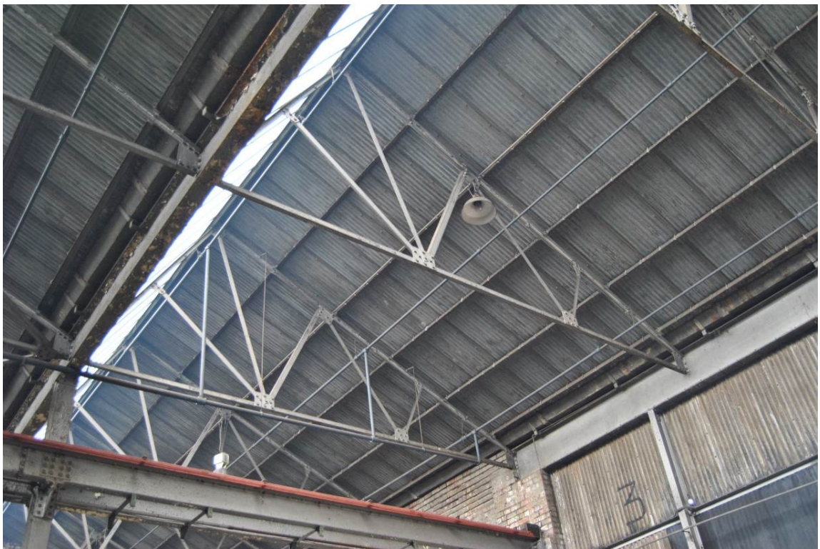
Plate 22: Asymmetrical 'north-light' roof structure, 'Zone A'.
