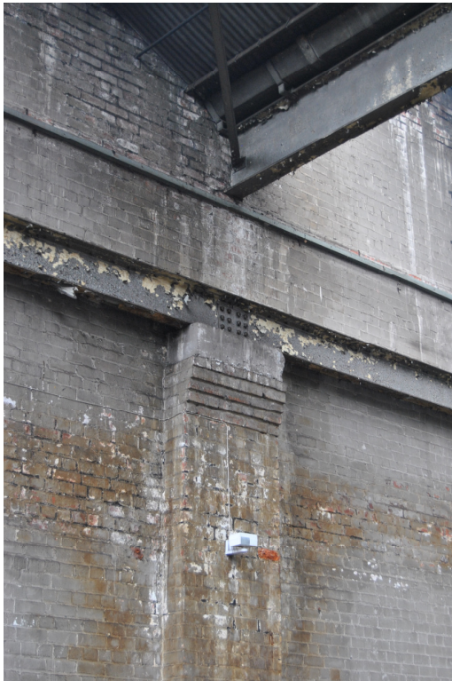
Plate 26: 'Zone A' high level rail for gantry crane supported on corbelled brick pier.
