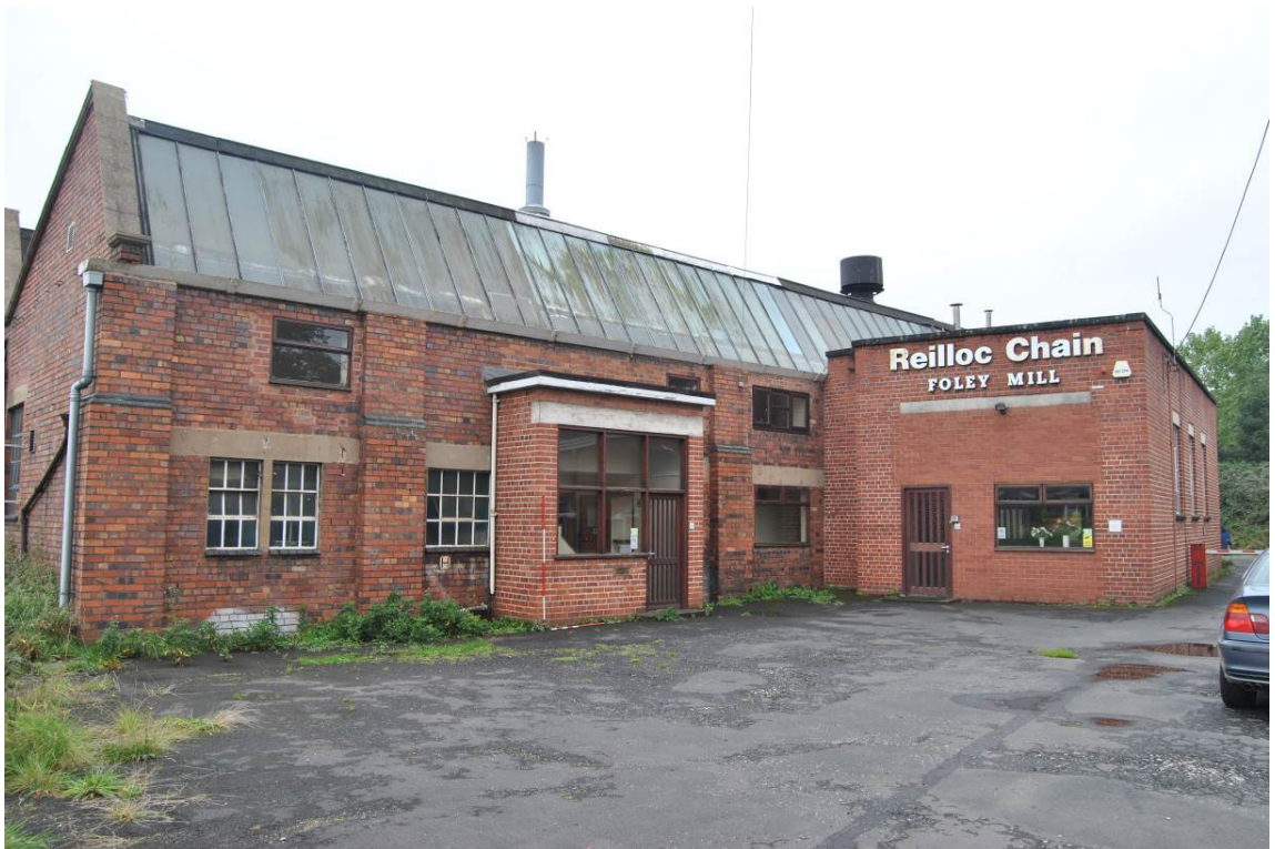
Plate 11: North elevation with secondary porch and former garage building, both c.1960. The porch would appear to have originally functioned as a covered loading bay (see Figure 12b). NB: Inserted windows to first floor offices.
