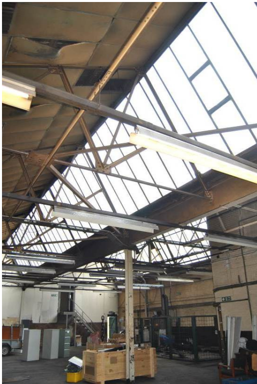
Plate 34: Detail of north-lit roof.
