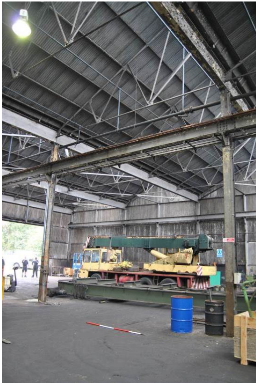
Plate 20: 'Zone A', Bays 1-3 looking south-west. NB: high level rails for gantry crane.
