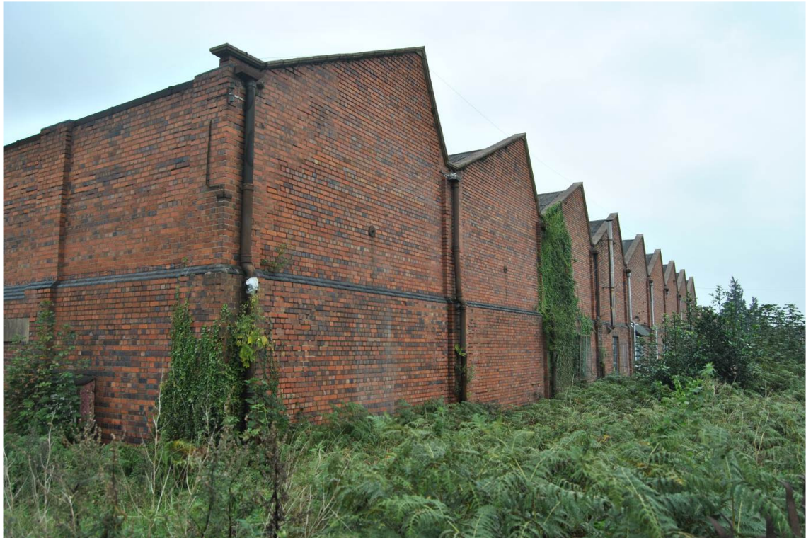
Plate 6: Detail of taller bays ('Zone A/B') looking north NB: offset of lower wall with blue-brick coving.
