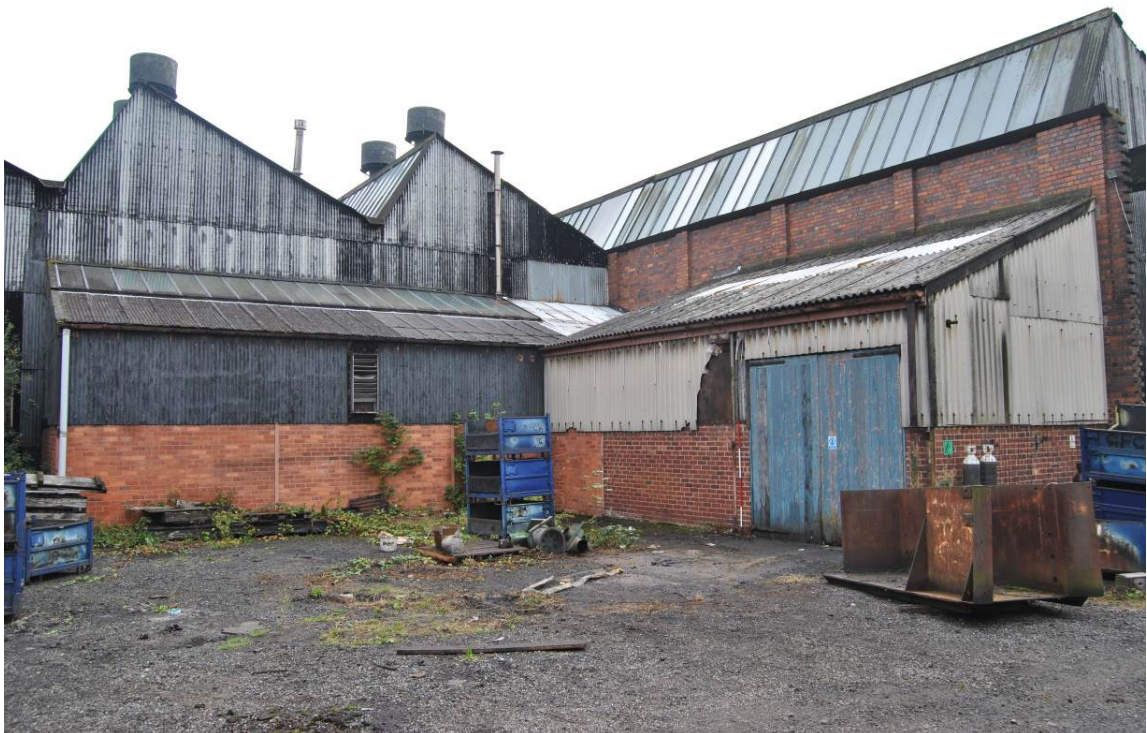
Plate 15: Phase I 'Zone A' (right) and 'Zone B' (left with north-light roof) ranges with Phase II, III and V lean-to extensions.
