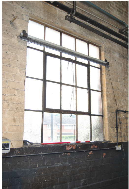
Plate 35: Typical steel-frame window with central opening panel.
