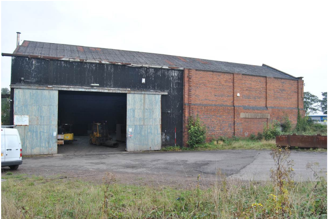
Plate 10: South elevation with wide, loading bay doors within framed shell (left) and blocked doorway within brickwork walls (right).
