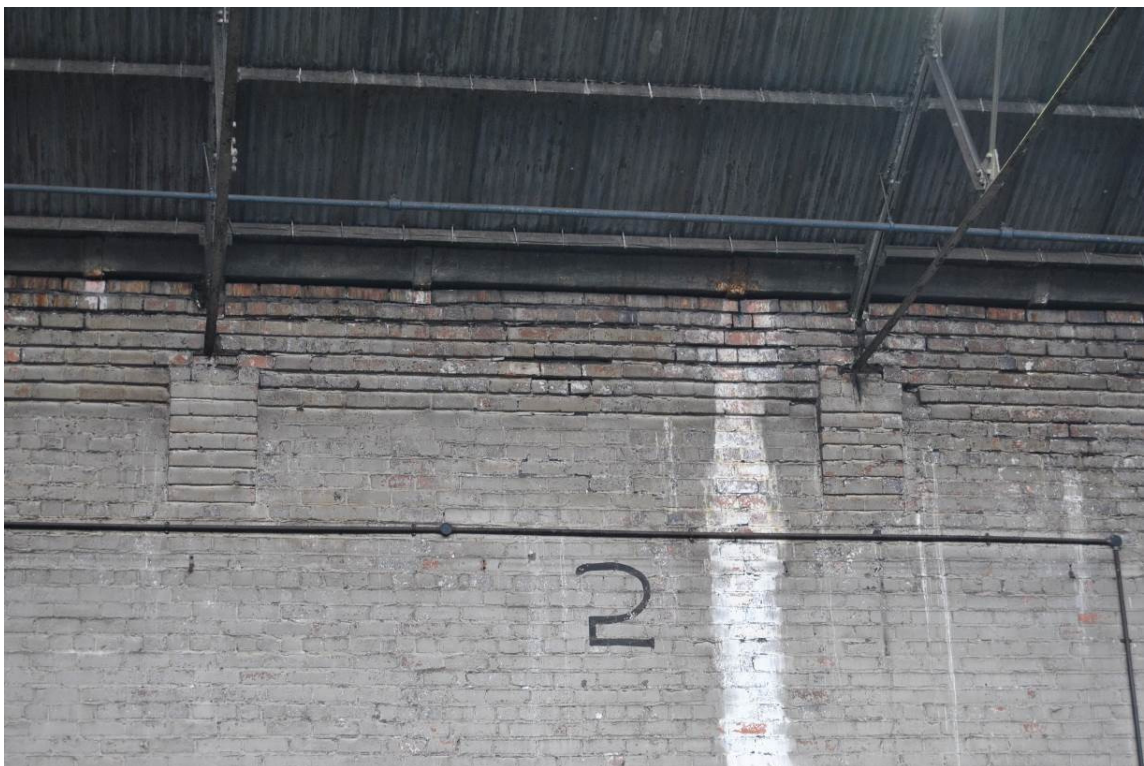
Plate 25: Roof trusses supported on corbelled brickwork.
