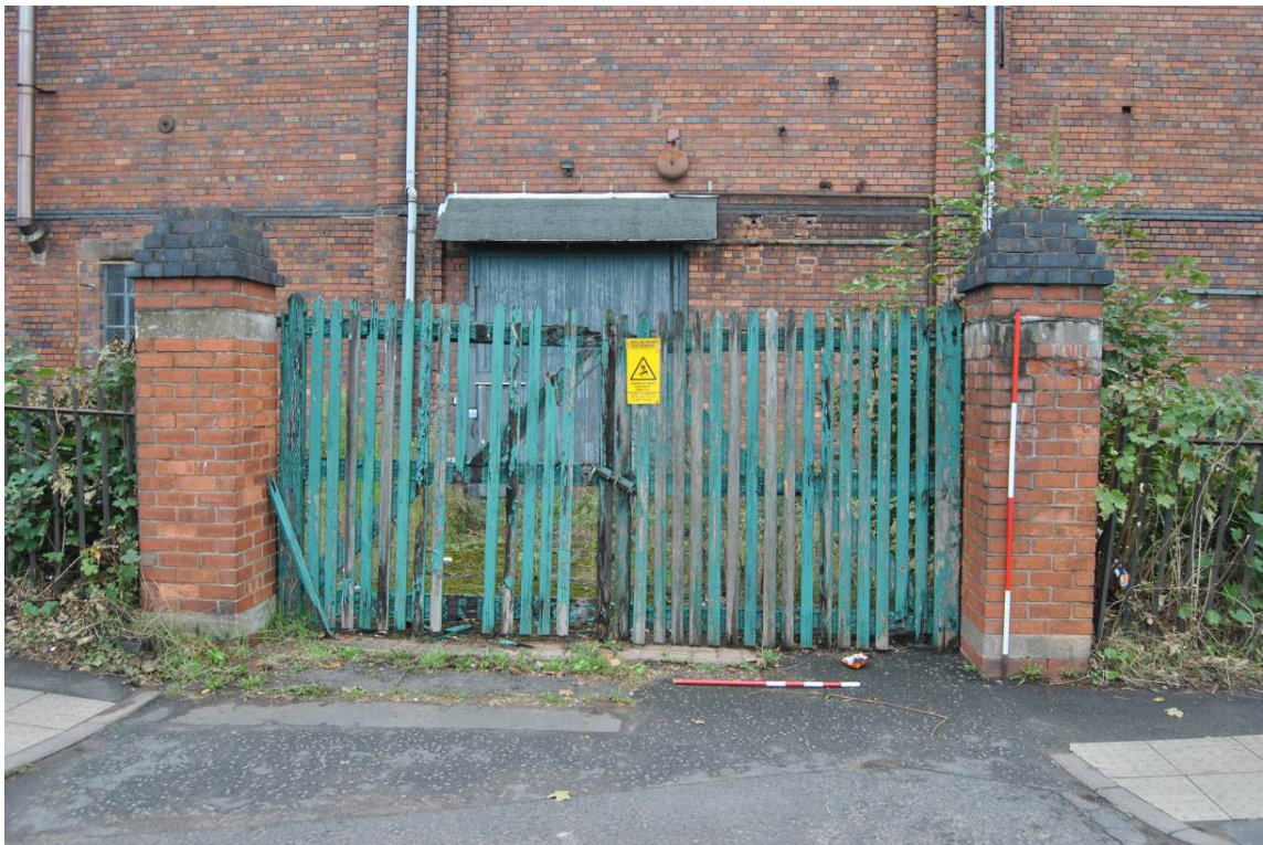
Plate 5: Original gate posts with stone hinge-blocks and blue-brick copings at Bay 5.
