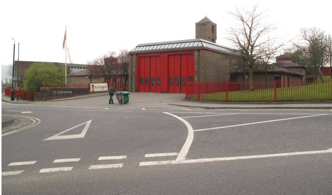
Plate 31 Fire station, Chapel Street, Mossley Brow
