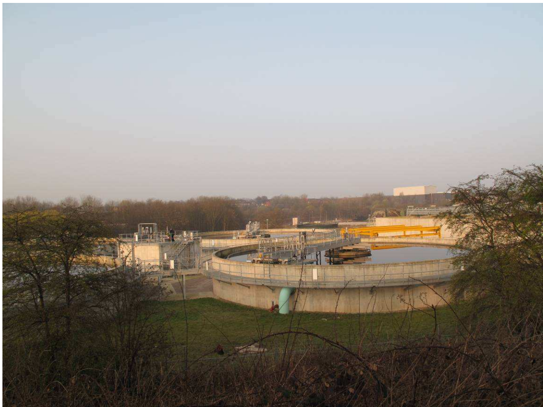
Plate 24 Sewage works off Gate Street, Hooley Hill
