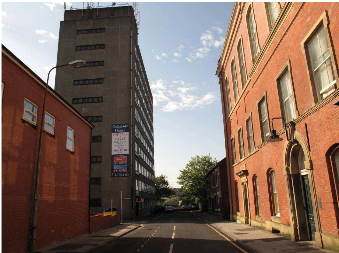
Plate 30 Booth Street, Ashton-under-Lyne – former government offices
