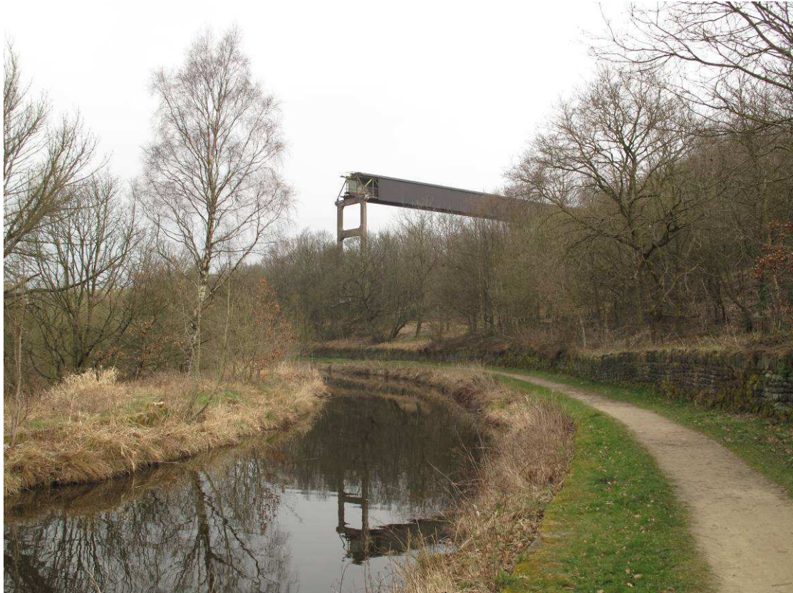
Plate 45 Huddersfield Canal and remains of mid 20 th century coal conveyor associated with former Hartshead power station site
