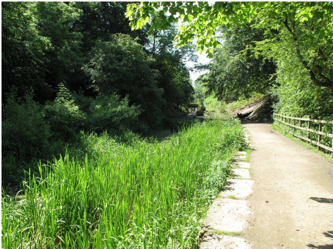
Plate 46 Section of the Hollinwood Branch of the Ashton Canal, Daisy Nook Country Park. Canal reused as green way
