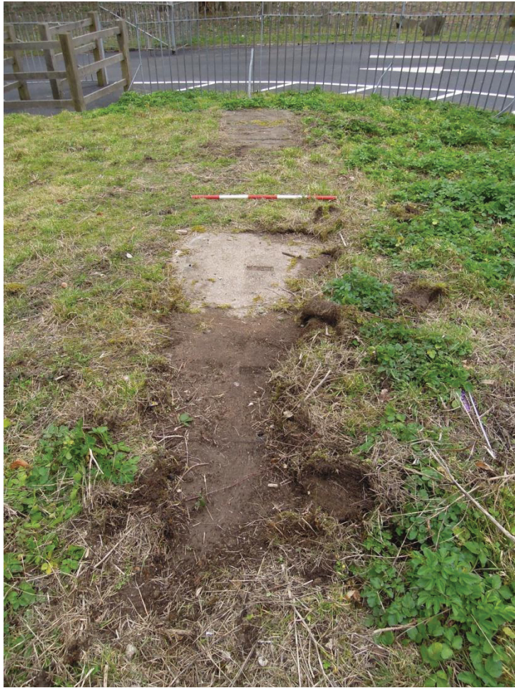
Plate IX , General view of concrete covers of two modern inspection chambers F.1, looking south (scale, 1m)
