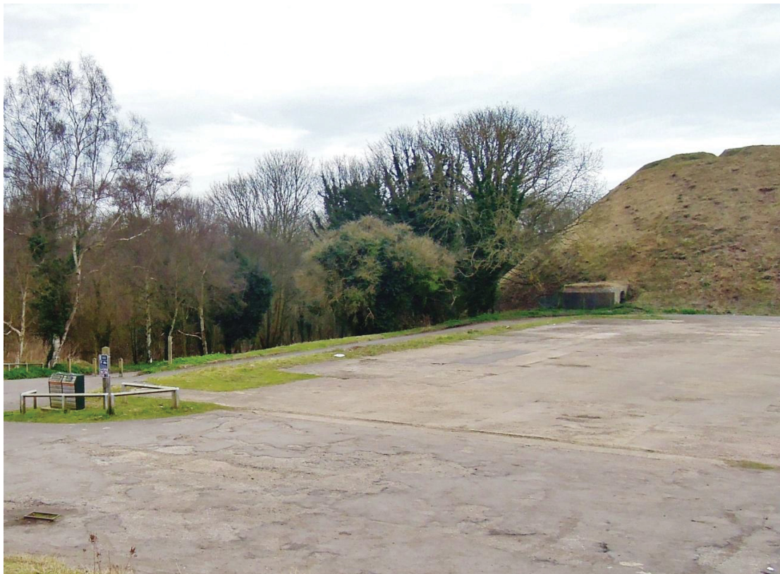
Plate XX , Anti-tank pillbox set into base of Horseshoe Bastion, looking south-east
