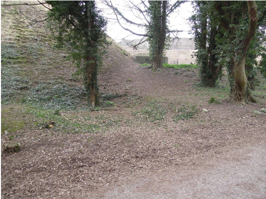
Plate XIX , Terminal of ditch F. 10 at foot of Horseshoe Bastion, looking south-west
