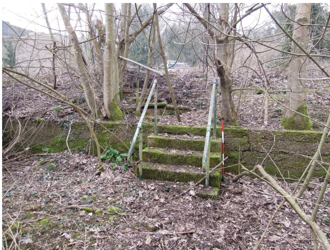
Plate XIV , Lower steps and concrete retaining wall relating to former building F. 8, looking north-west (scale, 1m)
