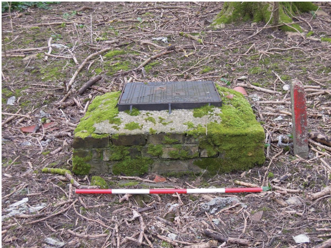
Plate XXII , Brick and concrete man-hole F. 11, looking west (scale, 1m)
