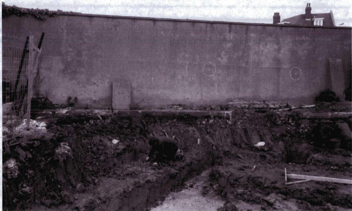
Figure 5: View of the excavation area looking north-east showing edge of the cleared area. Trench Two is at the centre of the photograph. The wall in the background of the photograph is part of the medieval town wall with some stone work visible at its base. As a direct result of evidence from the excavation, the wall has been listed by the De-
