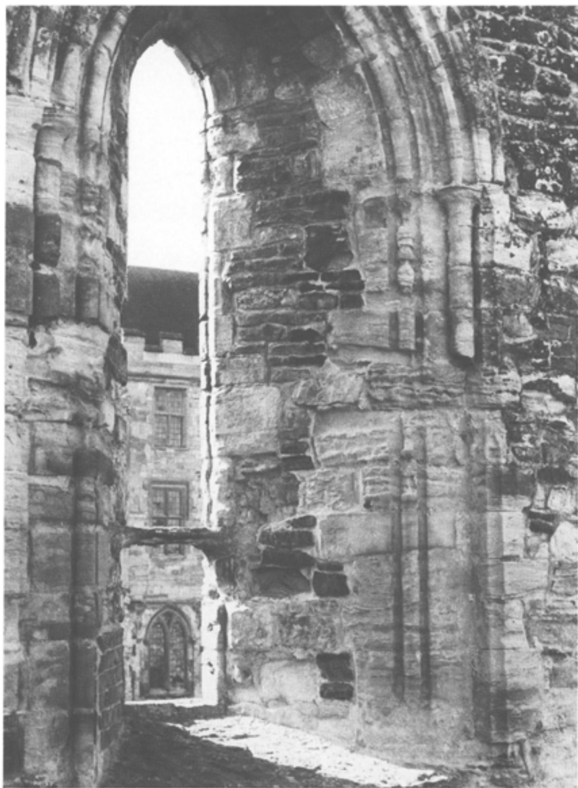
Plate 10 The dormitory: window moulding, and evidence for glazing and shuttering.
