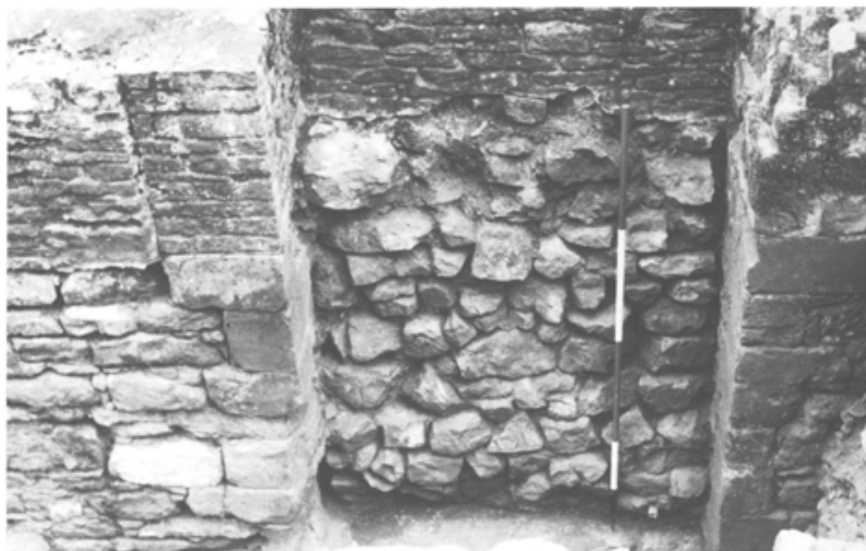
Plate 25 The blocking of the easternmost arch of the reredorter arcade, viewed from inside,
