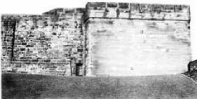
Fig 22 The south-east corner of the inner ward curtain wall showing the reconstructed section of Queen Mary's Tower (photo: Carlisle Archaeological Unit)
