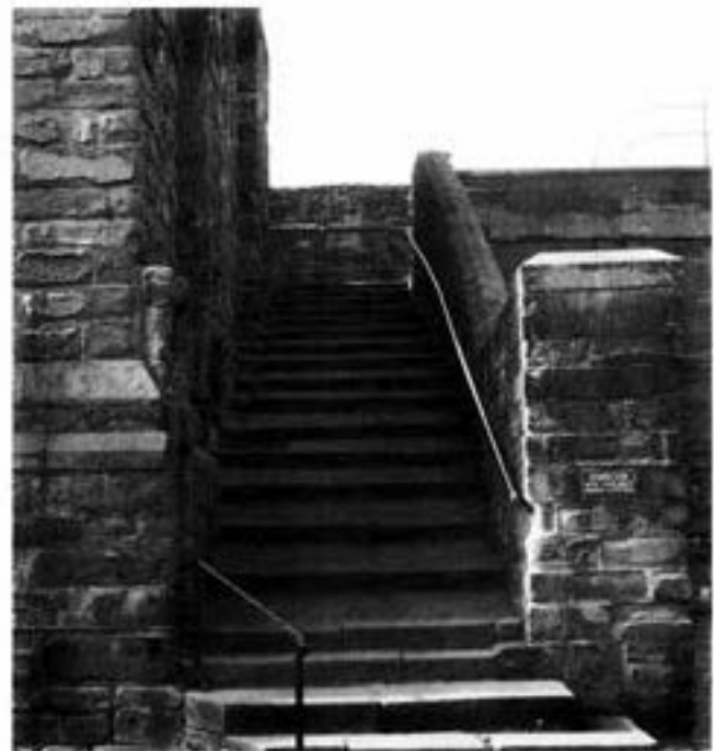
Fig 17 The ramp from the inner ward to the wall-walk (photo: Carlisle Archaeological Unit)
