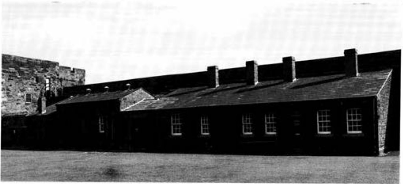
Fig 121 The north elevation of the Garrison cells showing the former Gun Shed and the Barrack Serjeants' Quarters (photo: Carlisle Archaeological Unit)
