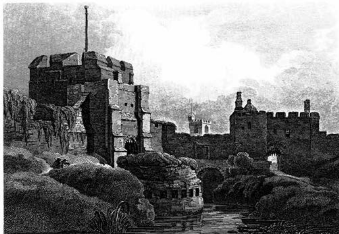
Fig 56 The half-moon battery, inner gatehouse and the inner ditch by Luke Clennel, 1813 (photo: Cumbria County Library)
