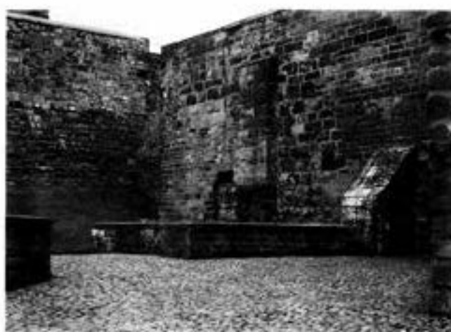
Fig 26 The south curtain wall over the inner bridge (photo: Carlisle Archaeological Unit)
