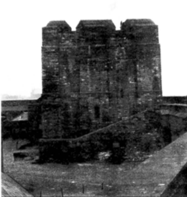
Fig 67 The north elevation of the keep showing the ramp (photo: Carlisle Archaeological Unit)
