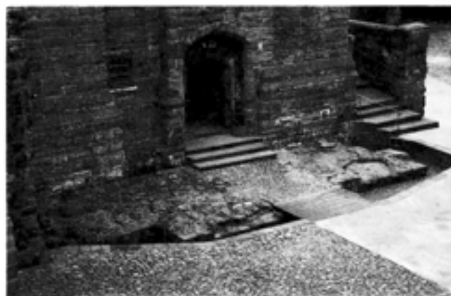
Fig 71 The forebuilding foundation
