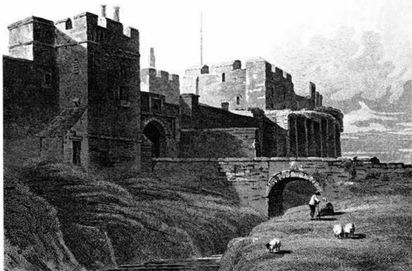
Fig 12 The outer stone bridge and outer gatehouse by Luke Clennel (photo: Cumbria County Library)
