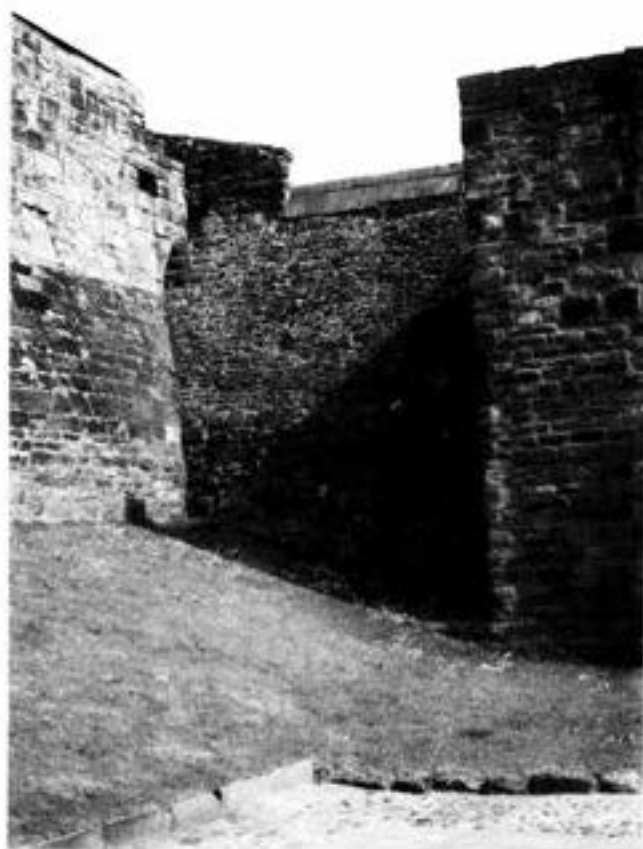
Fig 25 The junction of the south curtain wall with the inner ward west curtain (photo: Carlisle Archaeological Unit)
