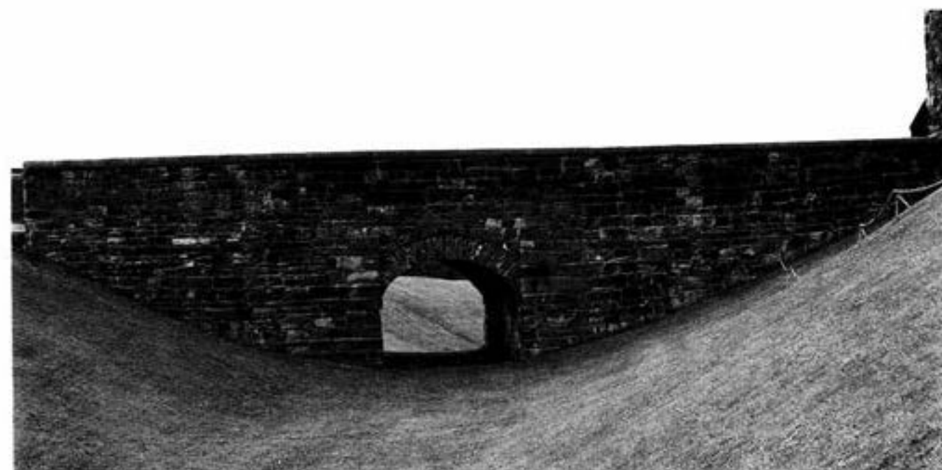
Fig 13 The outer bridge showing the east elevation (photo: Carlisle Archaeological Unit)
