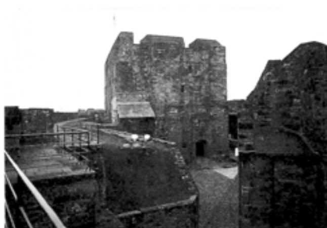
Fig 72 The east elevation of the keep and forebuilding
