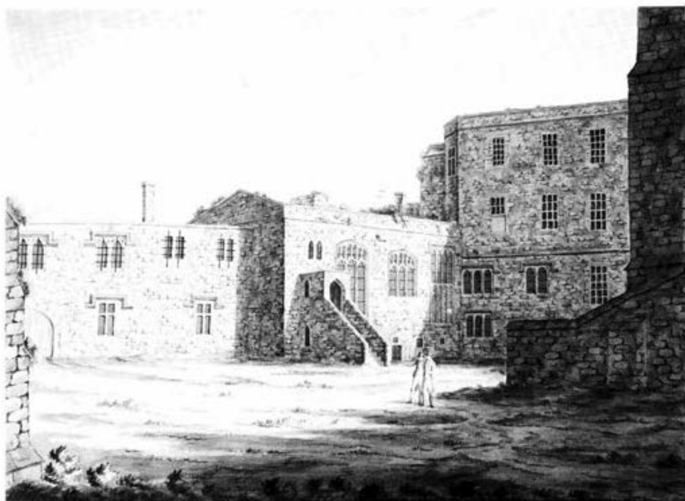
Fig 107 The inner ward showing the Great Hall (Regimental Museum) centre and the Elizabethan range (right), by Robert Carlyle c 1791 (photo: Carlisle Museum and Art Gallery)
