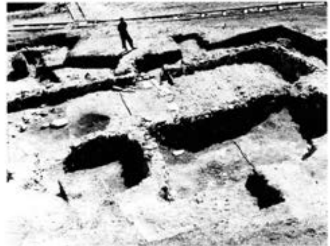
Fig 37 General view of Courtyard House 2
