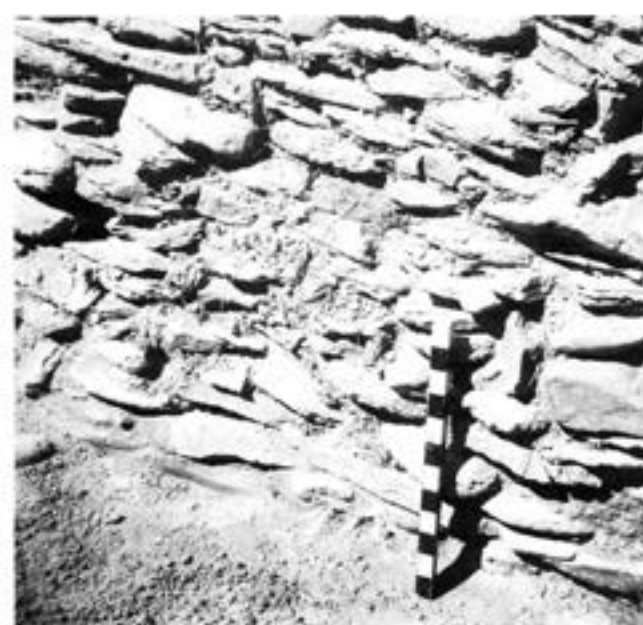
Fig 17 Courtyard House 1, Room 5: masonry and shillet plaster construction
