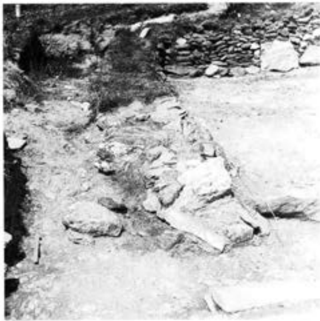
Fig 42 Courtyard House 2, Room 1: damaged wall west of south door
