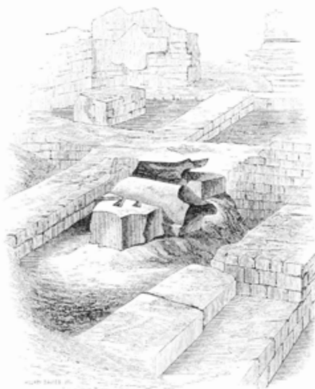
Fig 6.8 Rooms 9D and 9C looking north (Wright 1867, facing 157)
