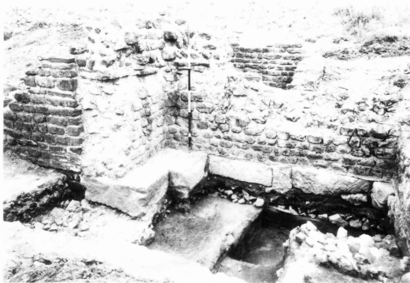
Fig 2.44 Room 5A; view east
