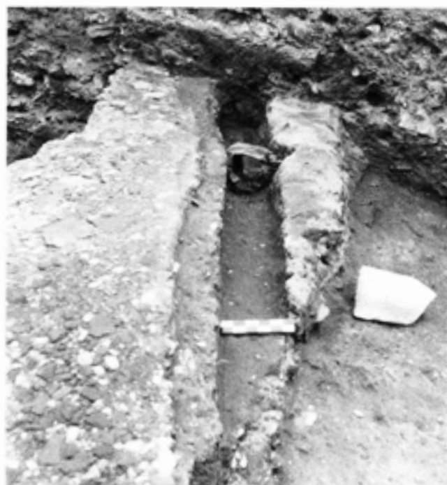
Fig 2.73 Baths precinct, drain F3191, view north-east
