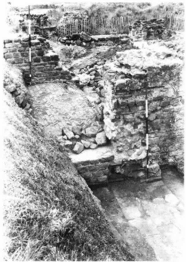
Fig 2.50 Room 11A exterior entrance and herringbone floor; view south
