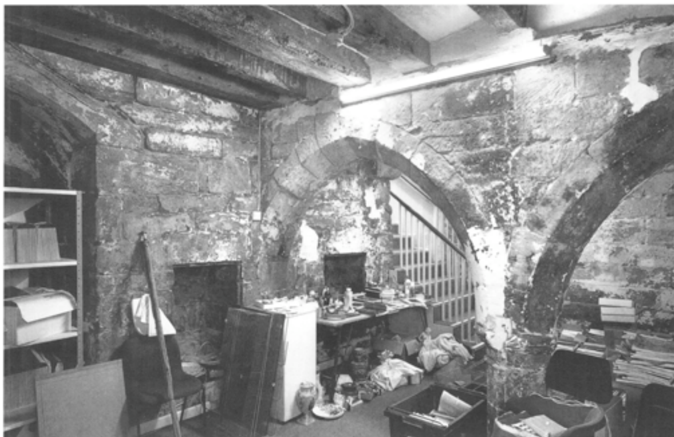
Fig 22 Eastern undercroft at Booth Mansion, 28–34 Watergate Street, showing the stone arcade, wall cupboards, and part of the rear doorway (RCHME © Crown Copyright)
