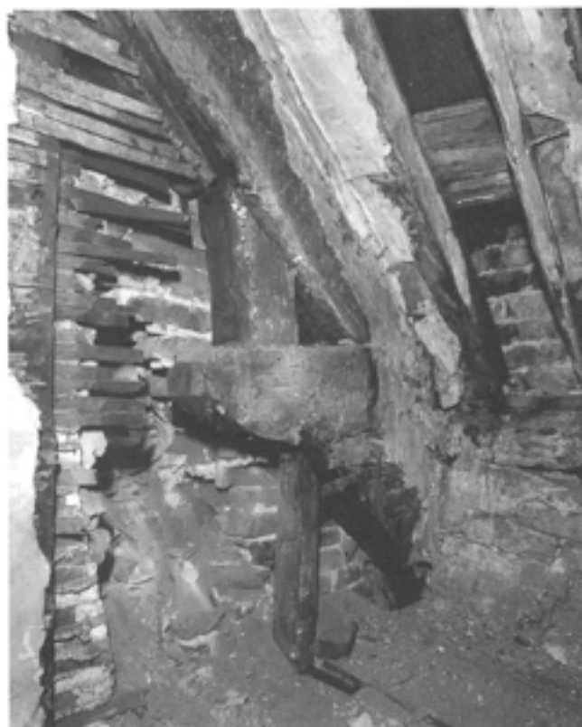
Fig 75 False hammer beam truss over the Roto chamber at the Leche House, 17 Watergate Street: also showing the moulded bressumer reused as a purlin (RCHME © Crown Copyright)
