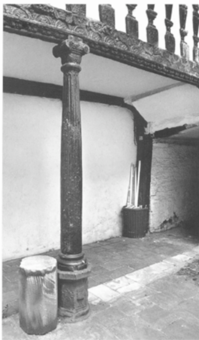
Fig 89 Timber post with classical details supporting the gallery at the rear of the Leche House, 17 Watergate Street (RCHME © Crown Copyright)
