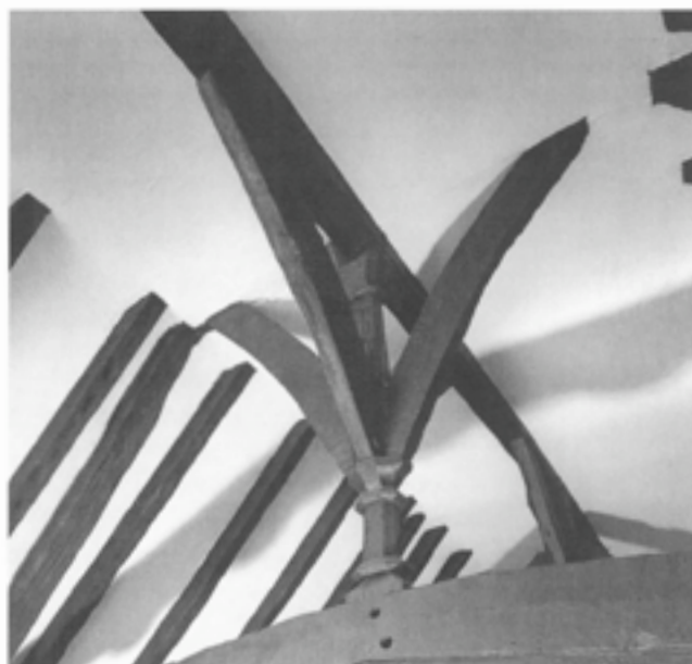
Fig 174 Crown-post roof in the Blue Bell, 63–65 Northgate Street (RCHME © Crown Copyright)
