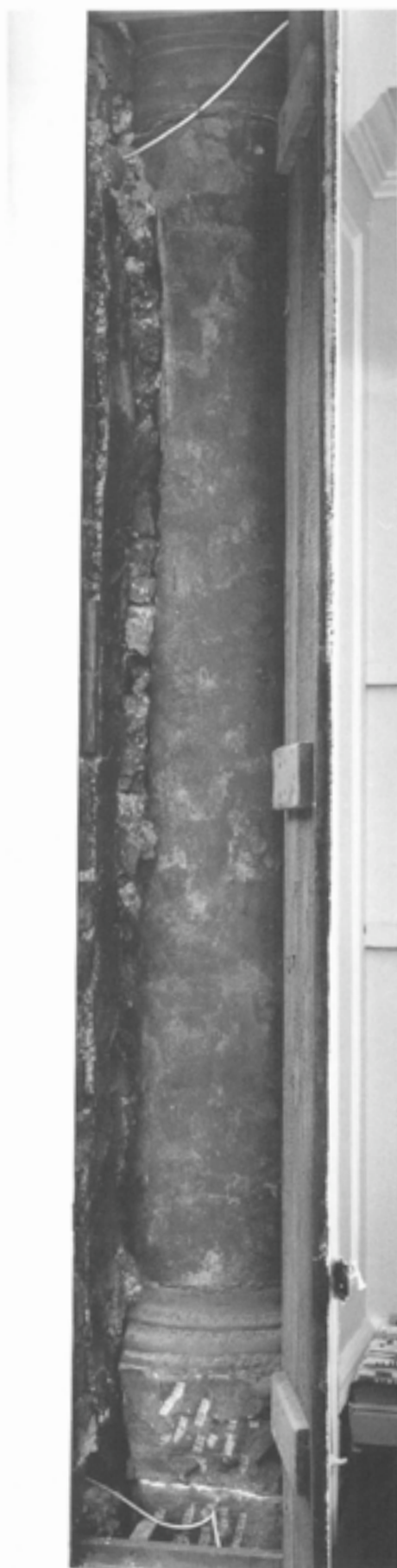
Fig 103 Tuscan column within the shutterbox at 48-50 Watergate Street (RCHME © Crown Copyright)
