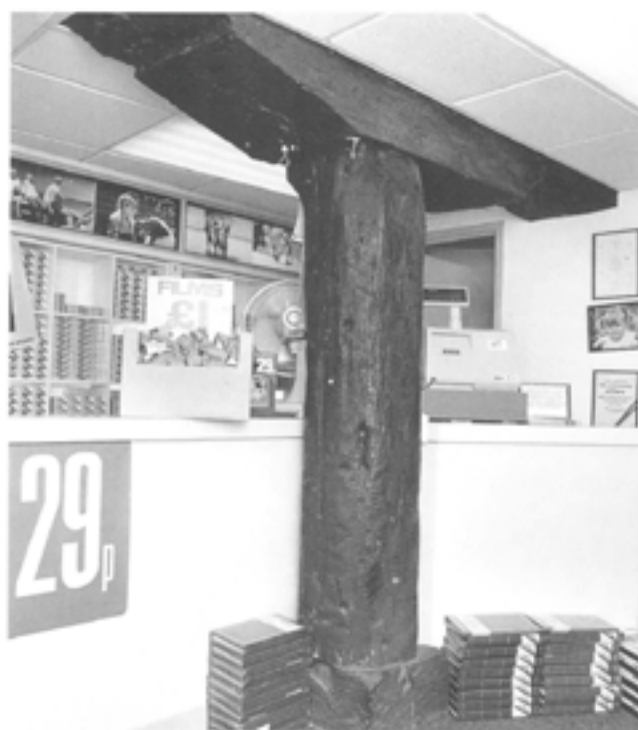
Fig 151 Timber arcade post in undercroft of 11 Bridge Street (RCHME © Crown Copyright)
