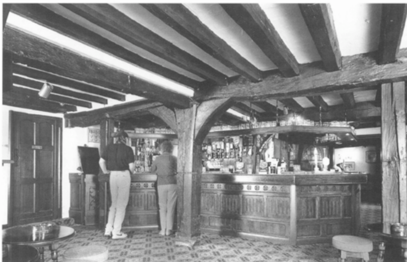
Fig 72 Timber arcade at the Old King's Head, 48–50 Lower Bridge Street (RCHME © Crown Copyright)
