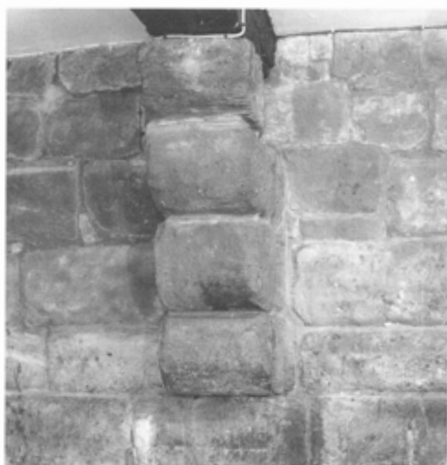
Fig 43 Corbels in undercroft at 39 Bridge Street (RCHME © Crown Copyright)
