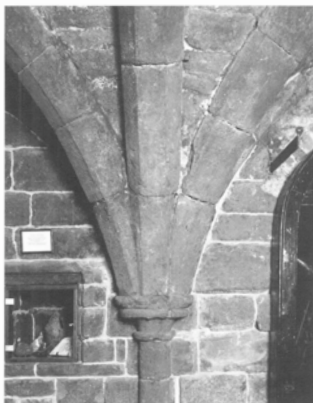
Fig 35 Respond of vaulting in undercroft at 11 Watergate Street (RCHME © Crown Copyright)
