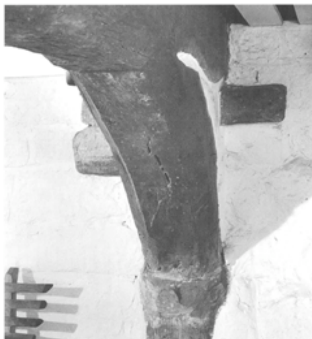
Fig 183 End of arch-braced beam in undercroft of 38-42 Watergate Street (RCHME © Crown Copyright)
