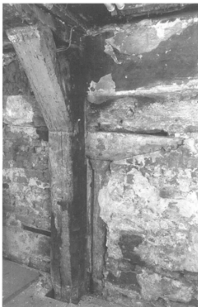
Fig 49 Part of the timber arcade in the western undercroft at Booth Mansion, 28–34 Watergate Street; the post in front belongs to later alterations when the ceiling was raised (RCHME © Crown Copyright)
