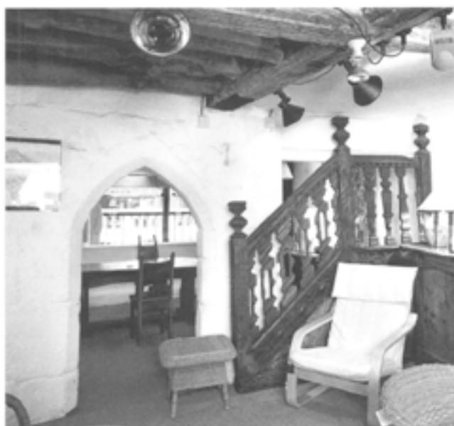
Fig 182 Roto level in 38-42 Watergate Street showing fourteenth-century doorway and displaced balustrade of Jacobean stair (RCHME © Crown Copyright)
