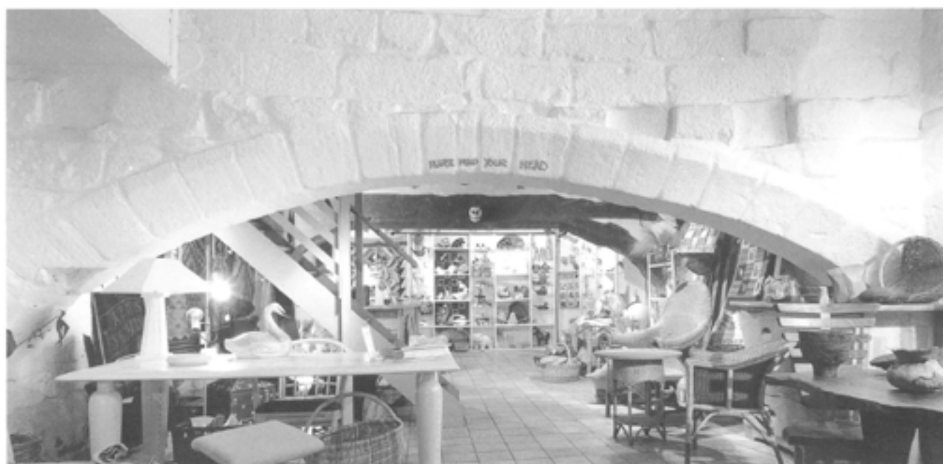
Fig 54 Depressed arch and arch-braced beam in undercroft at 38–42 Watergate Street (RCHME © Crown Copyright)
