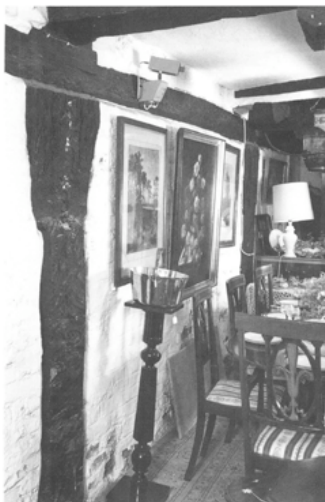
Fig 181 Timber arcade in west wall of undercroft in 22 Watergate Street (RCHME © Crown Copyright)
