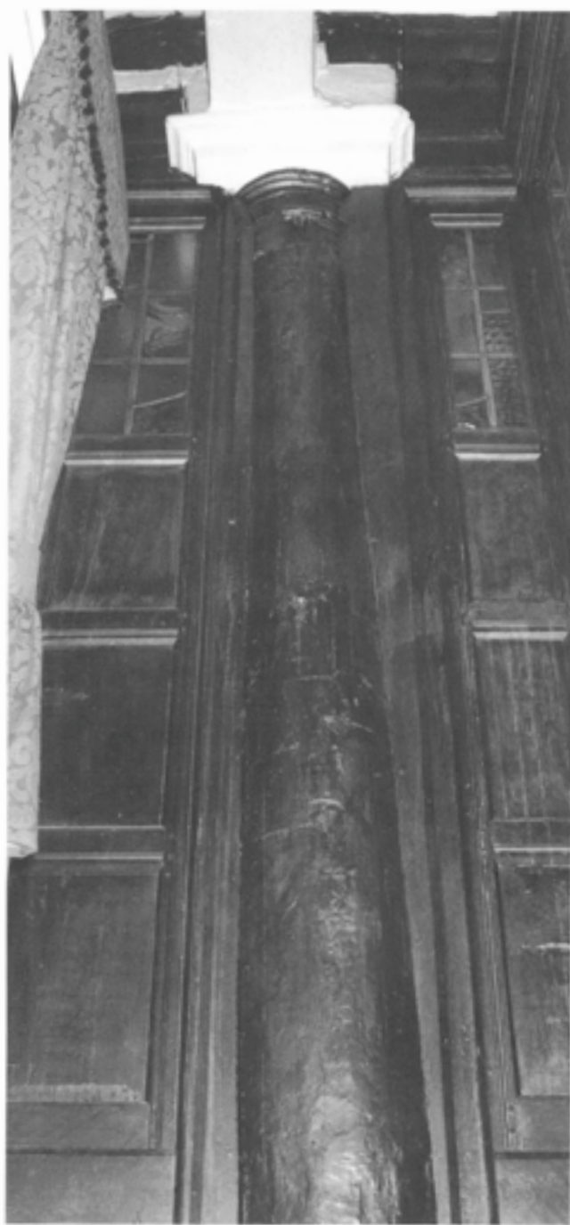
Fig 111 Tuscan column carved from a timber post at the Old King's Head, 48–50 Lower Bridge Street (RCHME © Crown Copyright)
