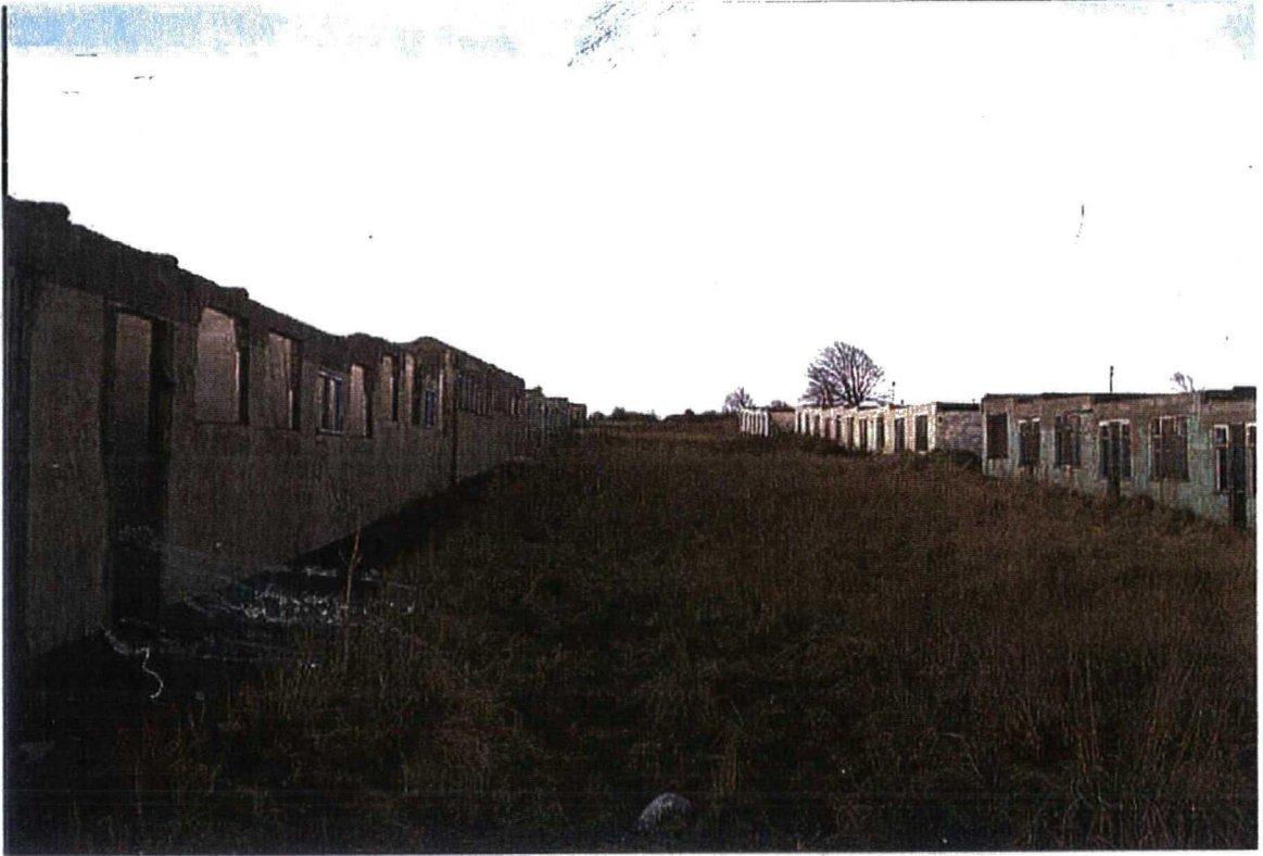
Plate 10 Roofless chalets in the north-east camp, with wide grassed strips surviving between, looking west
