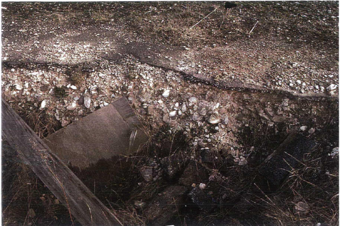
Plate 15 Excavated services in the south-east camp, showing what appears to be a considerable depth of made ground beneath the tarmac, although this could represent packing around the original service trench
