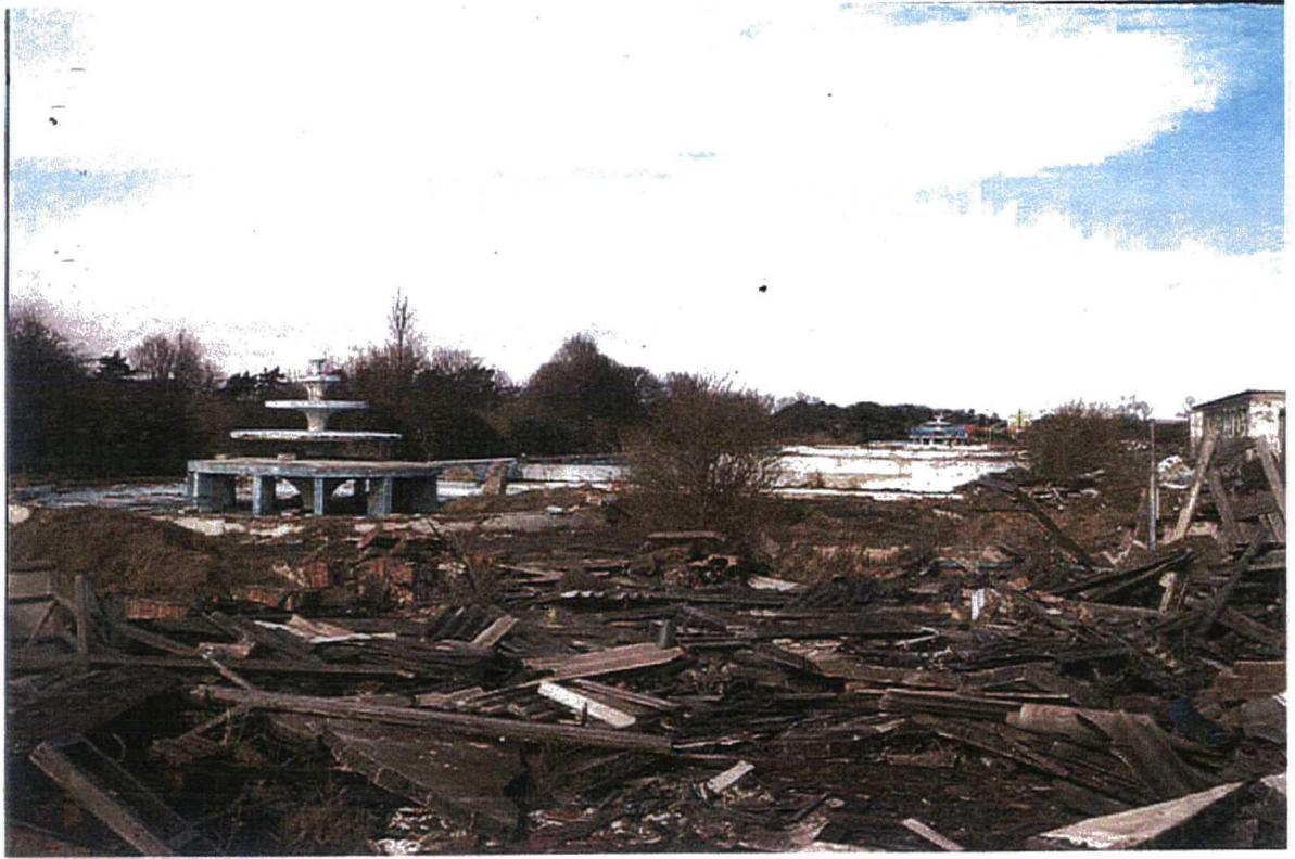
Plate 22 The outdoor swimming pool, looking north. The twin fountains were part of the original filtration system. The reinforced standing shell of the 1953 indoor swimming pool can be seen to the right
