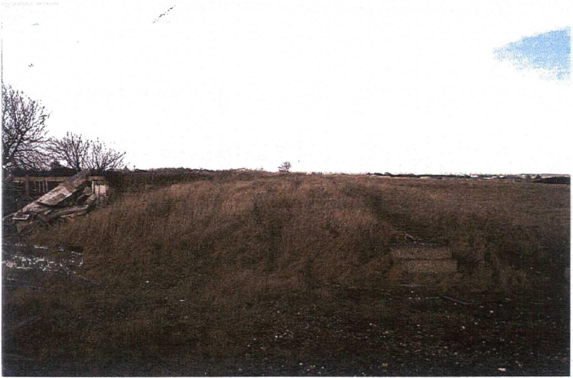
Plate 16 East-west artificial embankment leading between the original south-east camp (left) and 1969 chalets (right) towards the sports ground and undeveloped field in the distance, looking north. The unsurfaced track is reached by steps leading from the main track skirting the southern edge of the camp (foreground)
