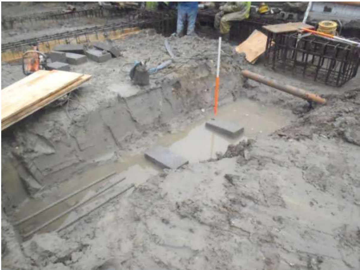
Plate 2 East-west trench in centre of site for concrete ring beam.
