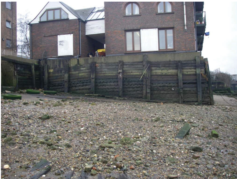
Fig 7: Revetment a340, looking west
