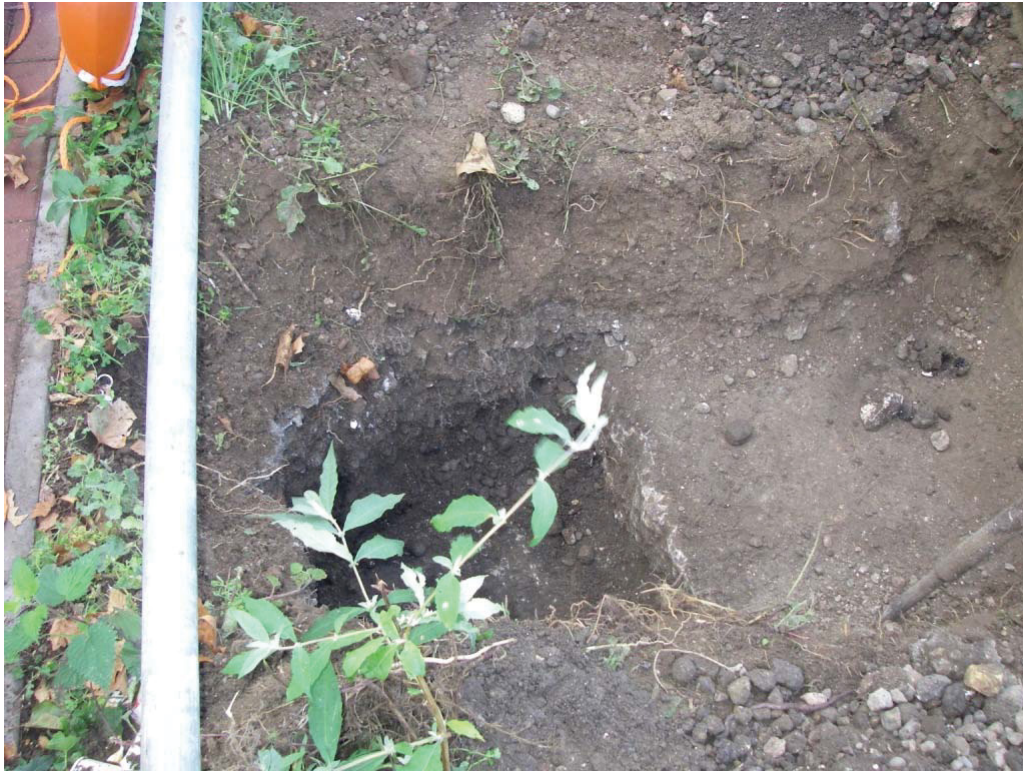
Fig 19: Trial Pit 06 looking west
