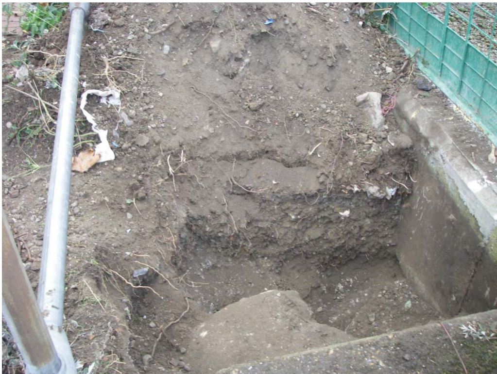
Fig 20: Trial Pit 07 looking west
