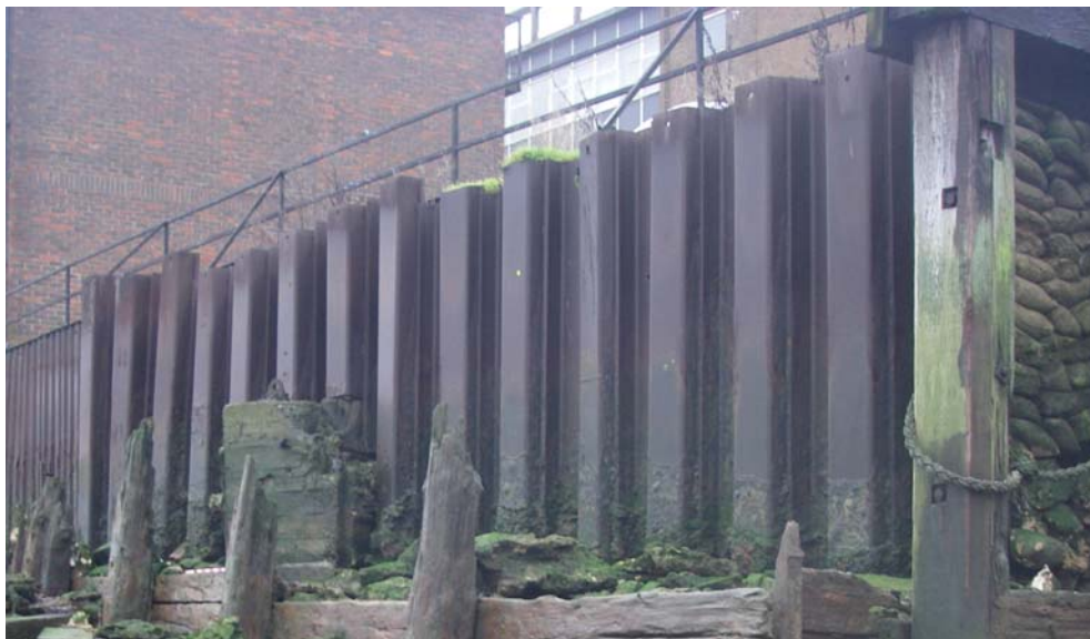
Fig 20: Revetment α338 Looking southeast © MoLA/TDP
