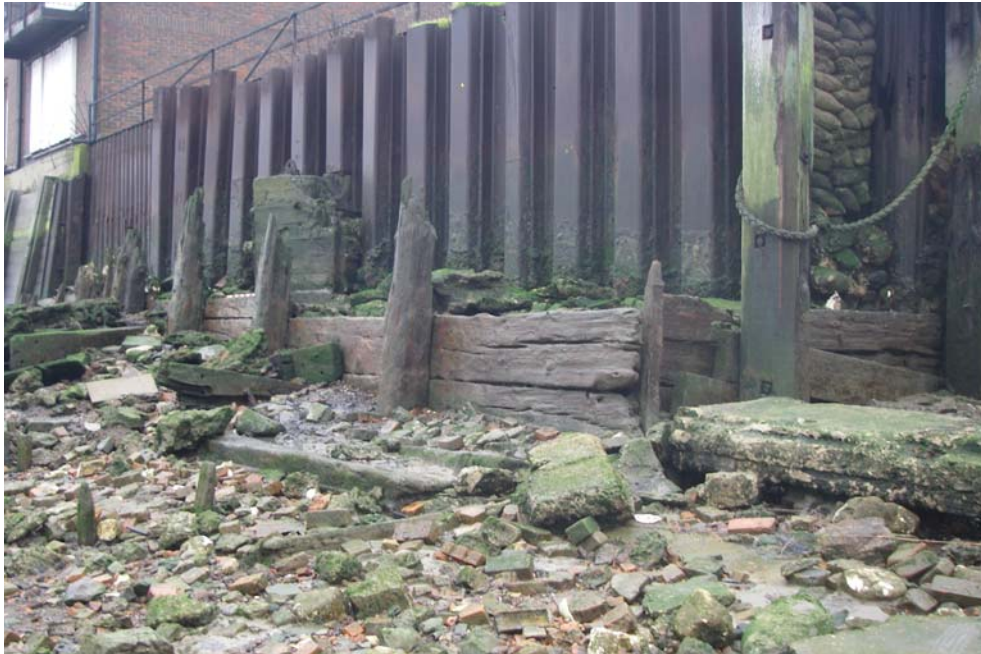
Fig 13: Revetment α336. Looking southeast. © MoLA/TDP
