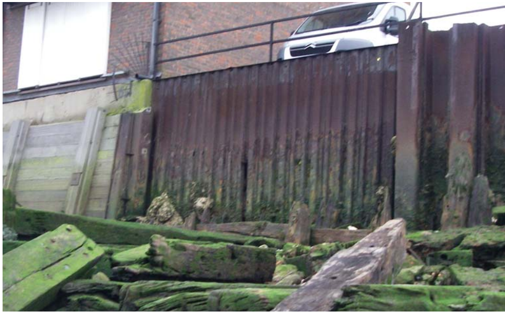
Fig 19: Revetment α339 Looking southeast © MoLA/TDP
