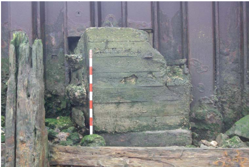
Fig 10: Crane base a341 Looking south © MoLA/TDP
