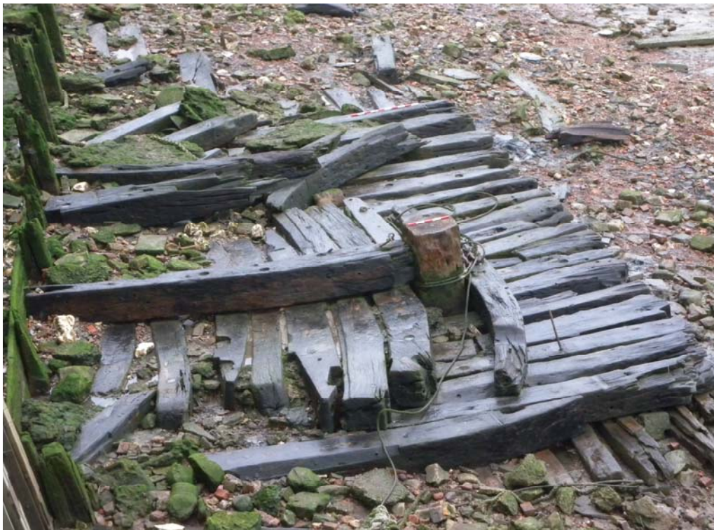
Fig 3: α333 looking west. Part of study site on left. ©TDP
