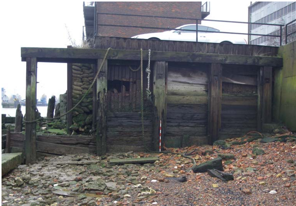
Fig 21: Revetment α314 Looking east © MoLA/TDP
