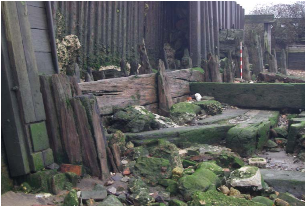
Fig 14: Revetment α336. Looking southwest. © MoLA/TDP
