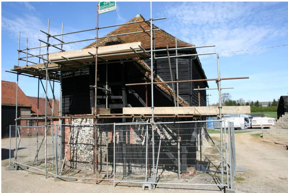
The south elevation shrouded in scaffolding.
