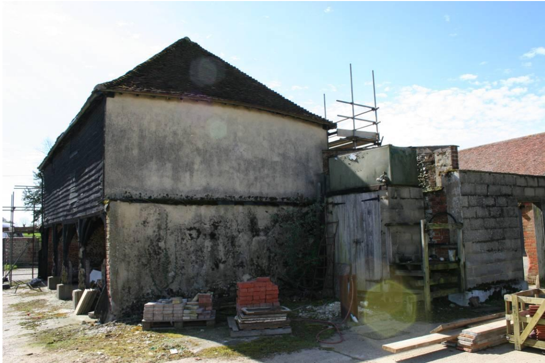
Northern elevation has been lath and plastered.
