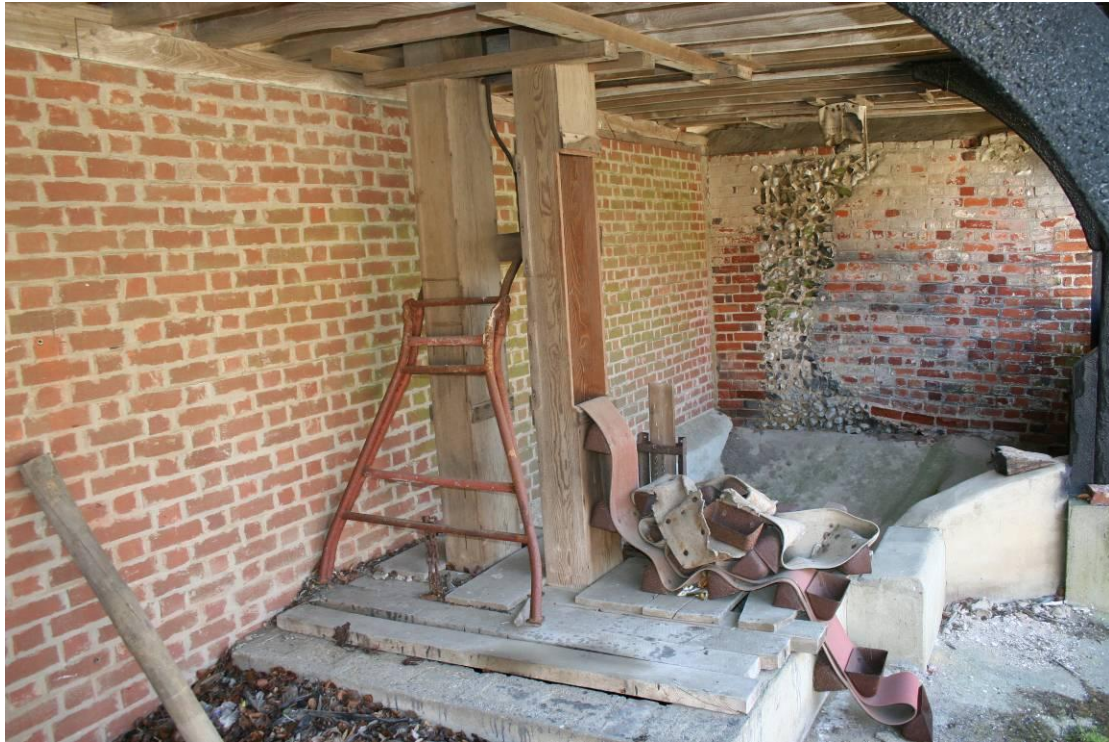
The grain elevator and hopper. The bucket belt has rotted away and fallen out.
