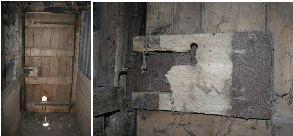
Door into the granary and its Woodstock lock decorated with mild steel plate.
