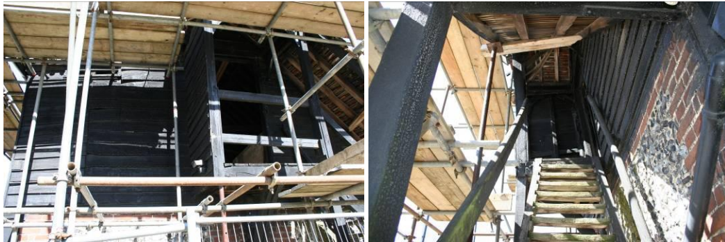
The lucam from the south. Looking up the ladder. Note iron bracket at top right.
