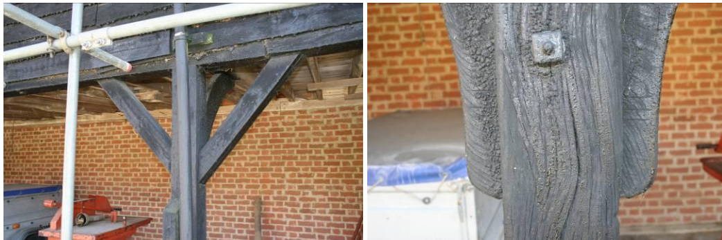
Central post has replaced braces. The others are numbered through.
