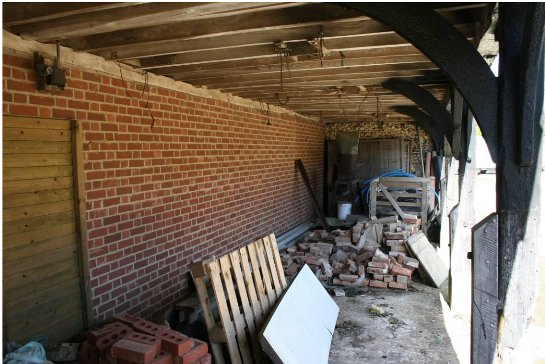
Modern spine wall replaces the original.
