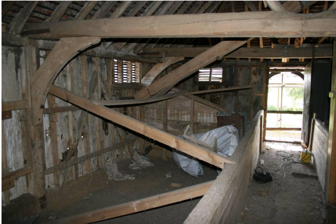
Tie-beams are supported on sculpted spandrels. Looking SE.
