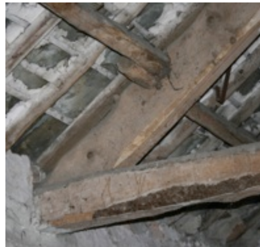
Plate 9. Part of the Roof Truss.
