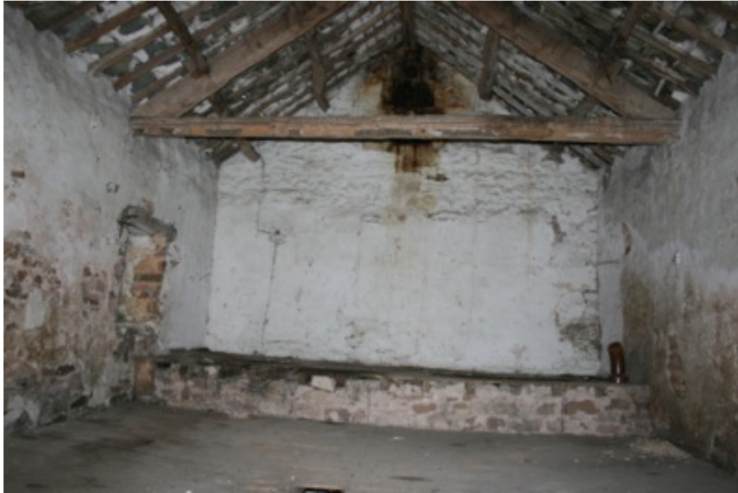
Plate 7. Interior of Granary Showing Raised Section of Wall and Floor.
