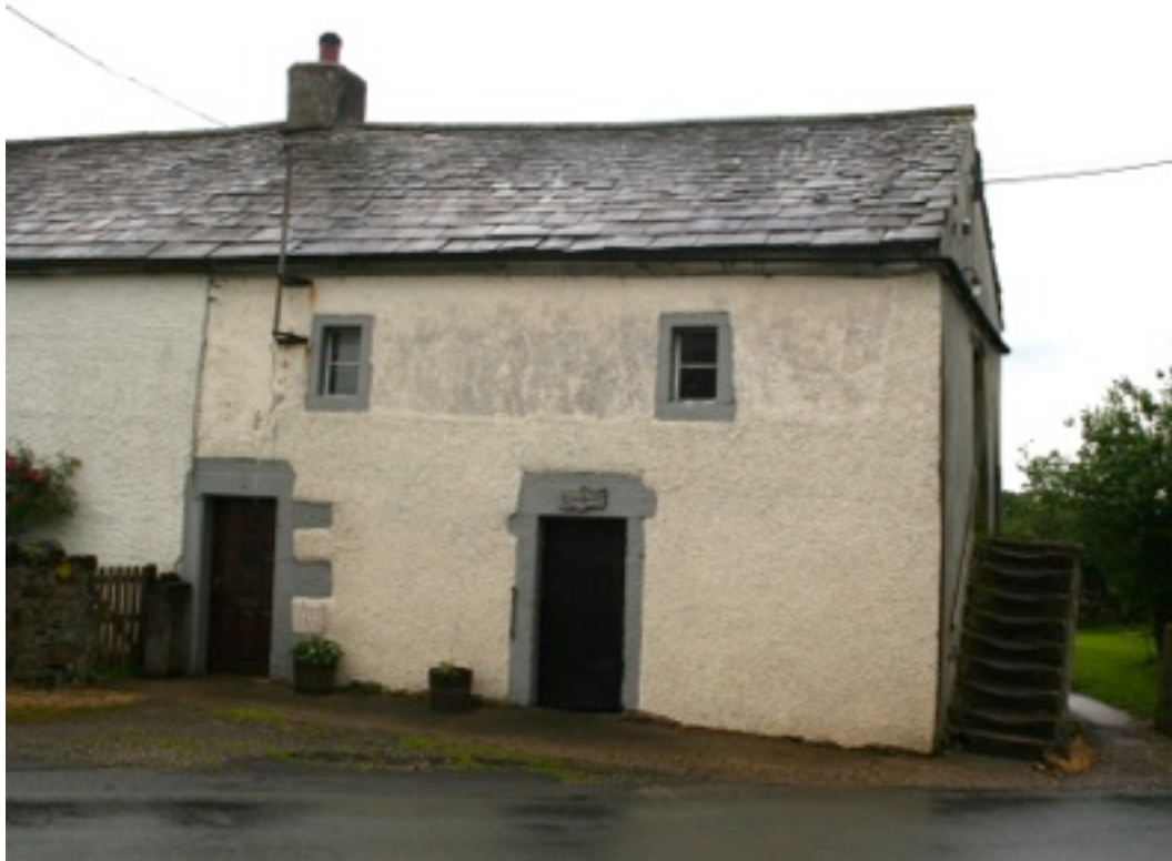
Plate 1. South East Elevation Showing Stone Dressings Around Openings.
