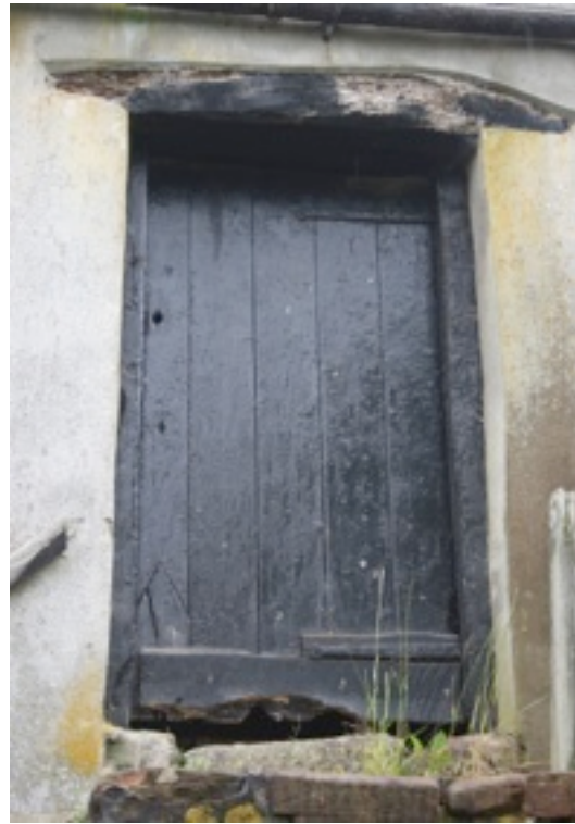
Plate 6. External Door to Granary.
