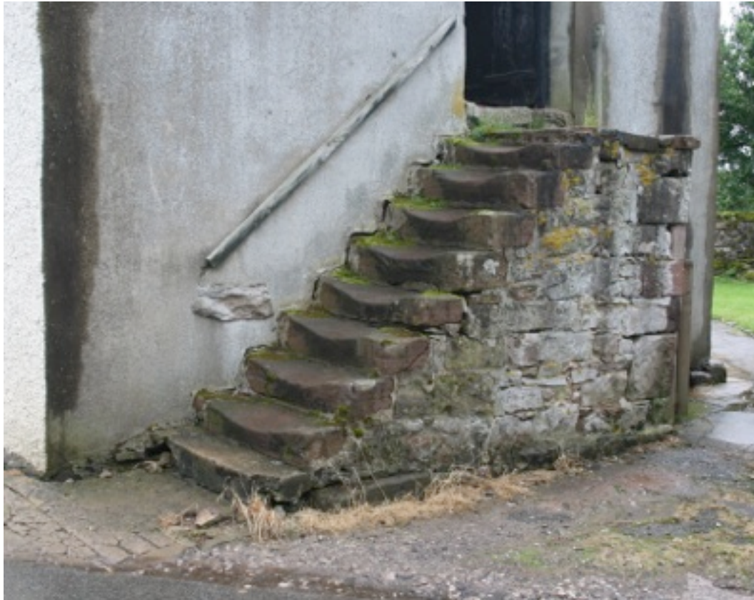
Plate 11. External Stone Staircase.
