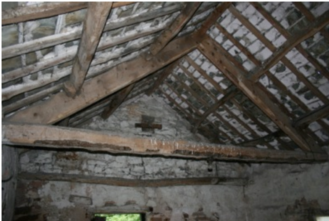
Plate 10. Inside of Gable to Granary.
