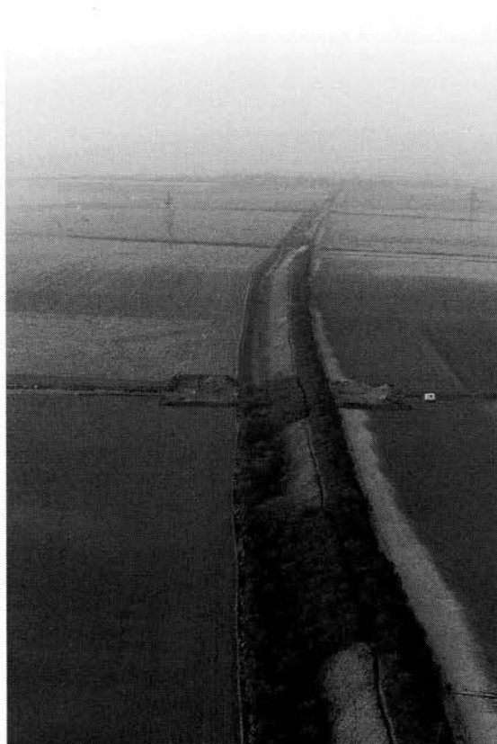
Figure 46. Devils Dyke from the air looking north-west, with the 1991 pipeline in the foreground and Gallows Hill beyond. Note the marked change in direction of the Dyke at this point. The 1991 excavation was in the scrub-covered ditch on the line of the water-pipe (photo: Ben Robinson, 1991).
