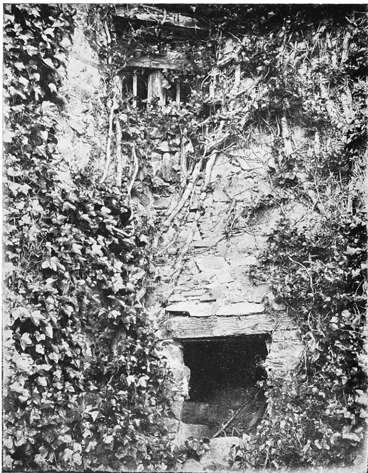
CONISTON HALL ; WINDOWS OF THE SPIRAL STAIR.
