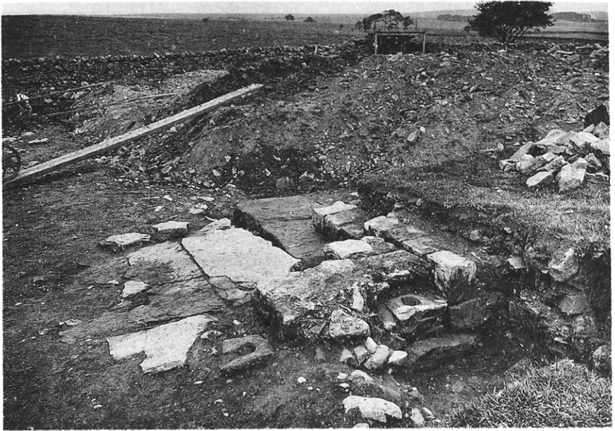
FIG. 21.—E. SIDE OF S. GATE, FROM S., SHOWING PIVOT-HOLES OF LEVELS IA, IB AND 2.
