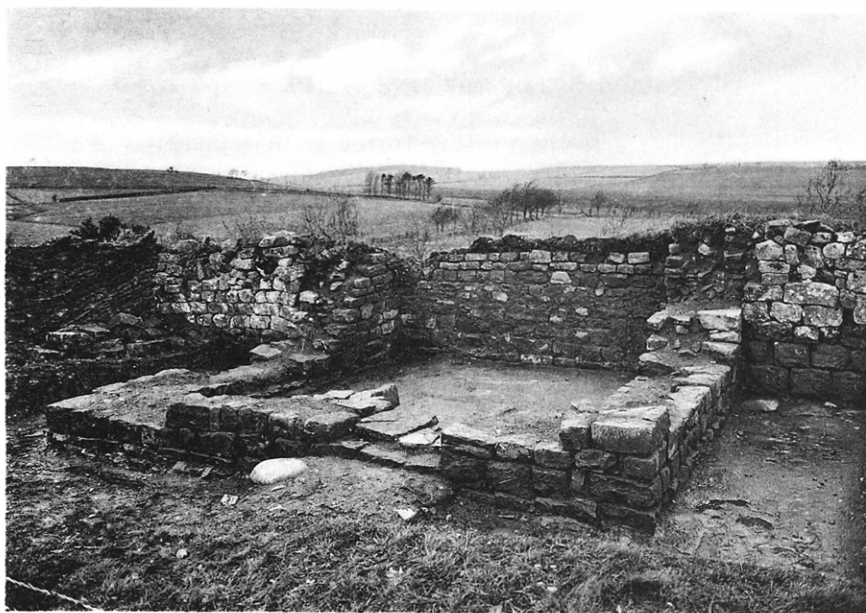
FIG. 1.—BIRDOSWALD TURRET, LOOKING N.W.
