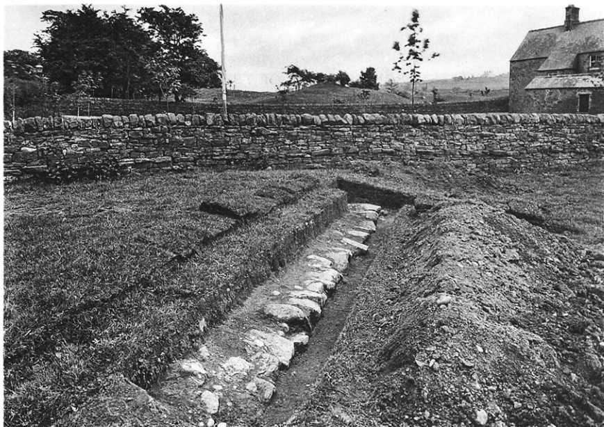
FIG. 46.—SOUTH KERB OF MILITARY WAY AT SECTION 7, LOOKING E.
