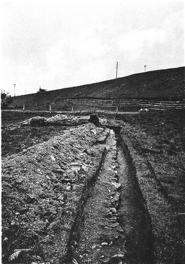
FIG. 43.—SOUTH KERB, BETWEEN SECTIONS 3 AND 4, LOOKING E
