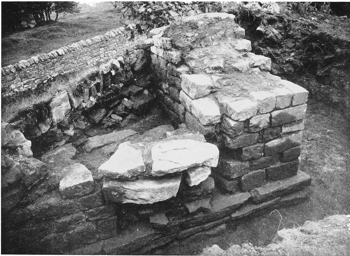
FIG. 25.—PIKE HILL SIGNAL-TOWER: showing rough walling in doorway tcwaas_002_1933_vol33_0020
