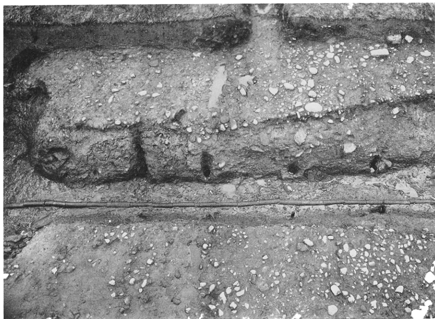
FIG. 8.—Causeway and culvert at Turf-Wall milecastle 50 TW, from the north.
