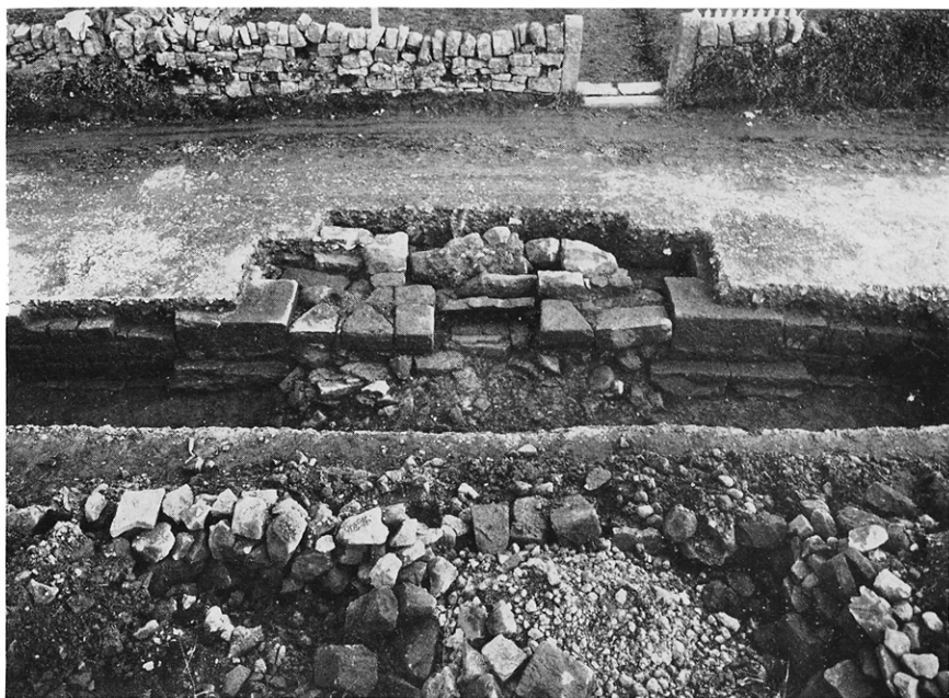
FIG. 24.—Bankshead milecastle, 52, north gate from the north.
