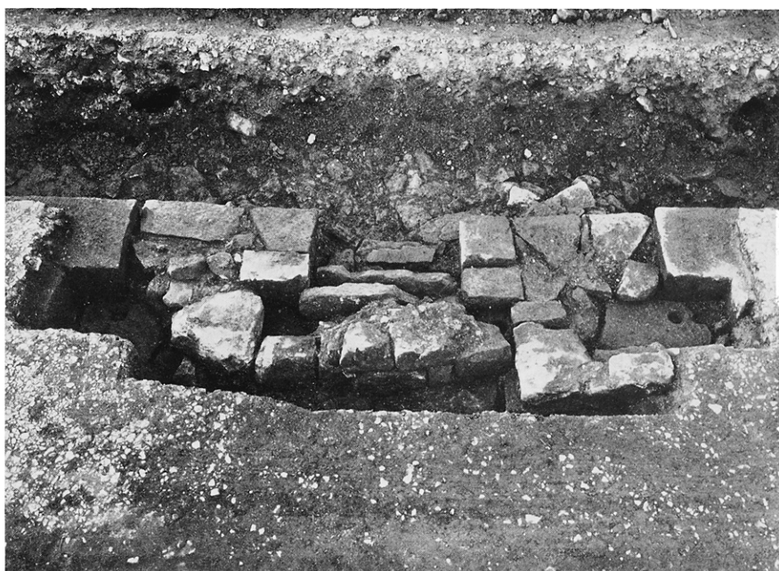
FIG. 25.—Bankshead milecastle, 52, north gate from the south, showing reducing-walls and later blocking.
