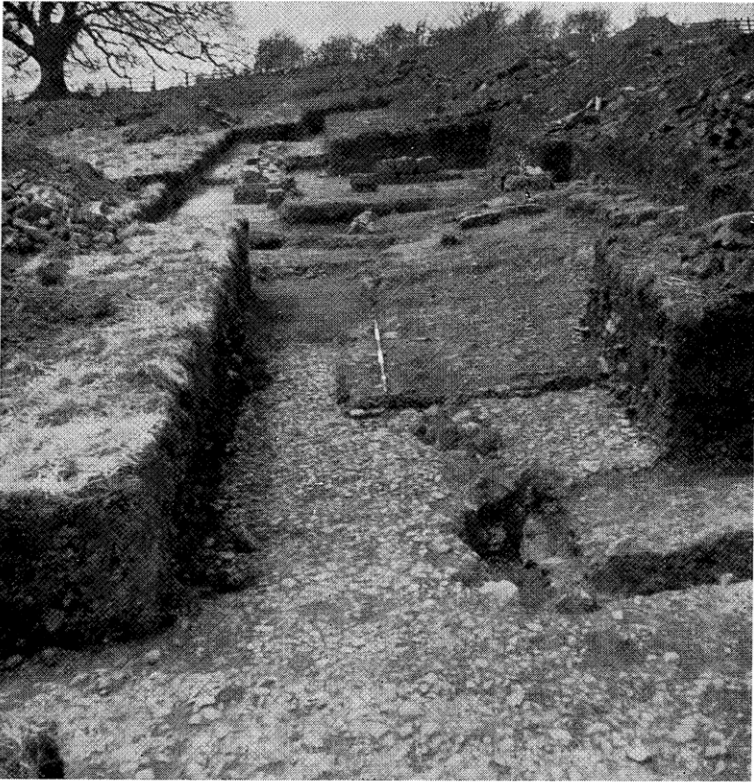
PLATE I, a.—Barrack block, looking east.
