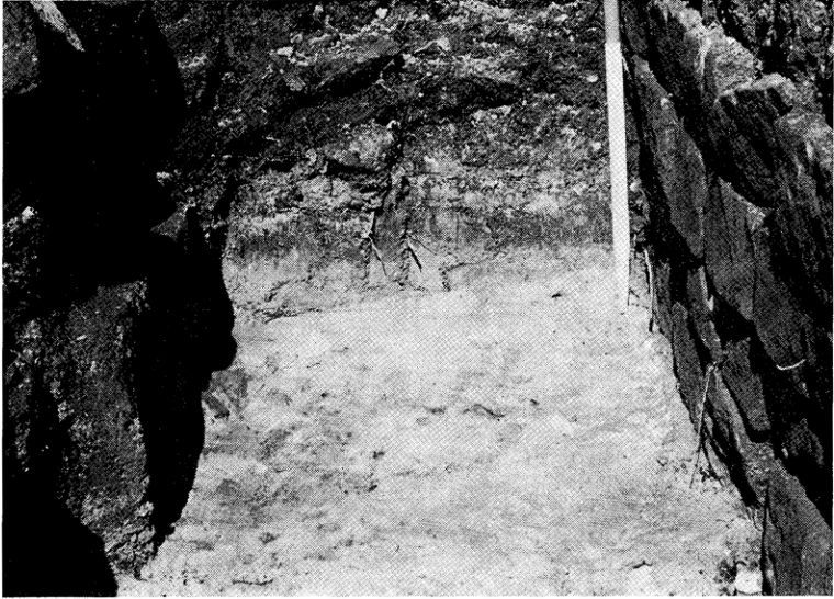
PLATE I.—Turret west wall and remains of Turf Wall.
