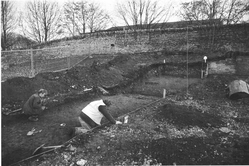
Plate 1: Excavation of Trench 01 in 1997 showing, in the background, the exposed rubble core of the Outer Bailey bank.
