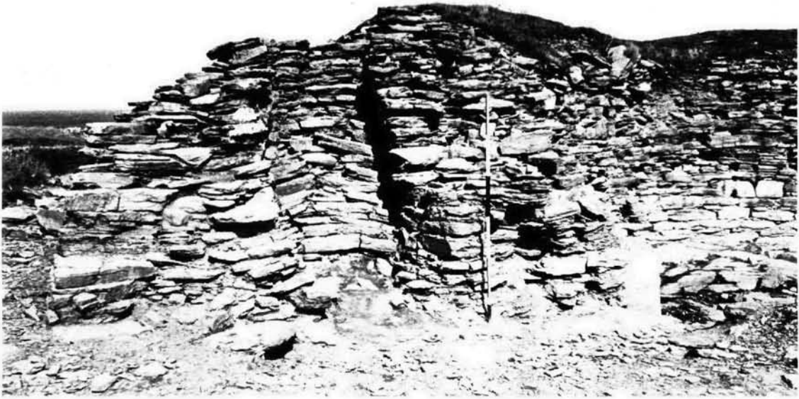
ILL. 17 : The buckled steps of the intra-mural stair: the breach in the foreground was made by later stone-robbers
