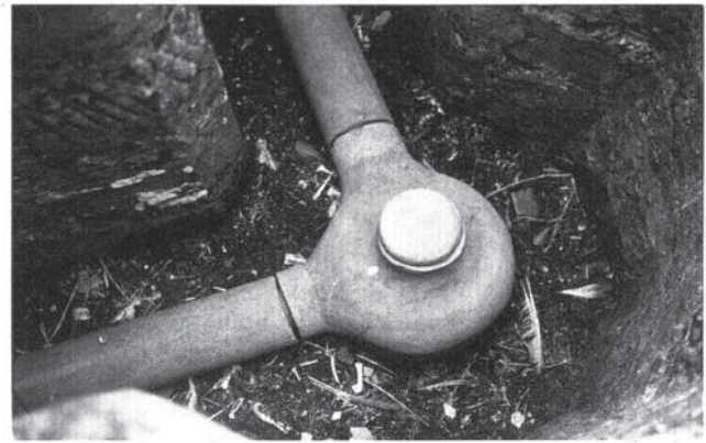
Figure 9.13 Ceramic junction box and pottery water pipes, part of an extensive and sophisticated medieval pottery water system uncovered at Glenluce Abbey, Dumfries, during clearance work in the 1930s (Photo: J le Patourel)
