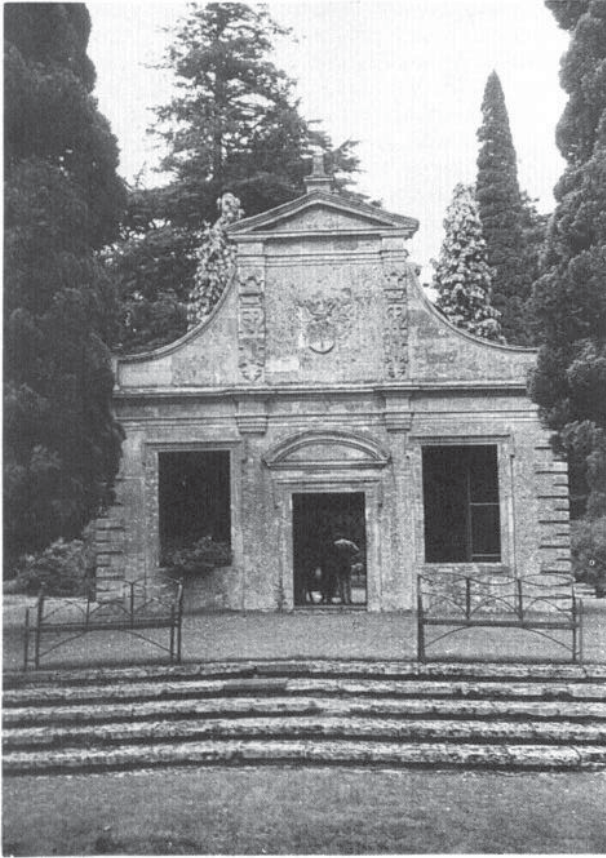
Figure 11.6 The garden pavilion dated 1641 at Easton Neston, Northamptonshire, surviving from an earlier garden layout
