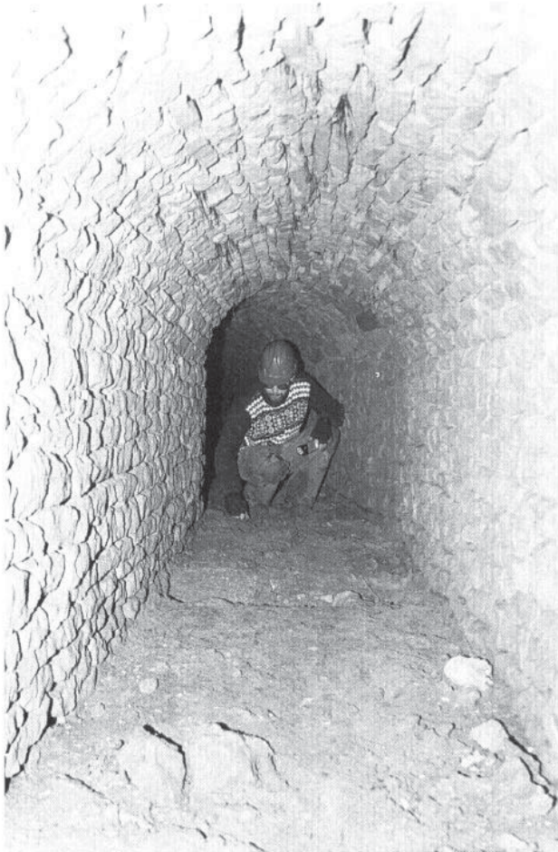
Figure 6.5 Kirby Hall: tunnel beneath part of the West Terrace
