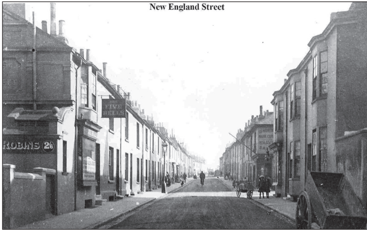
Fig. 3. New England Street — typical of houses demolished.
