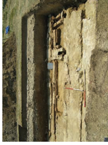
Wall [3/003] and associated drains looking south
