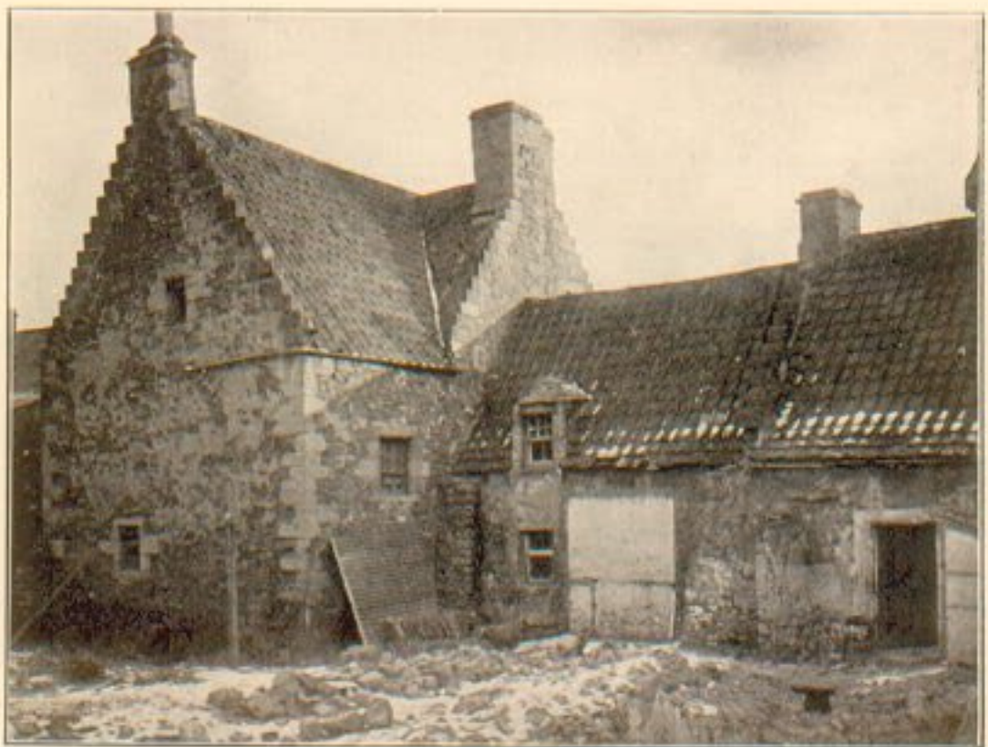
Fig. 2. Back view of Houses at Inverkeithing.
