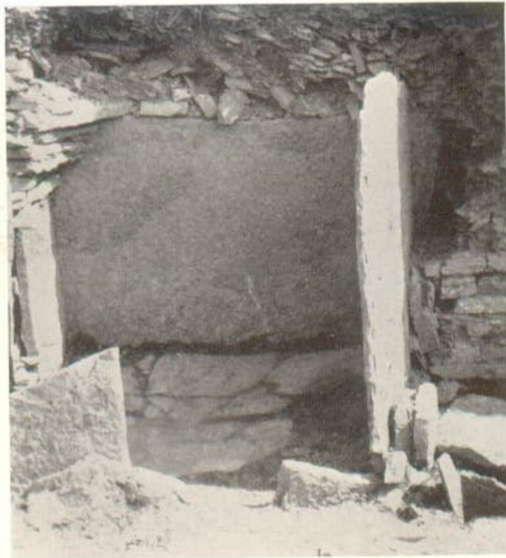
2. Radial Compartment No. 11, showing inserted packing-stones between broken wall of tower and side slab.
