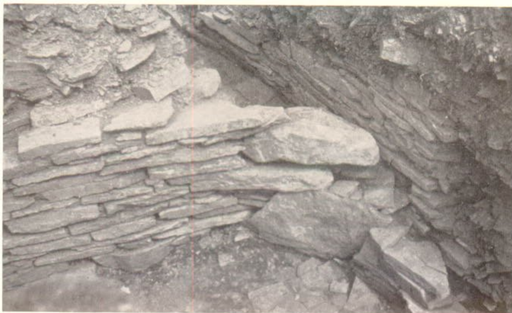
3. Chamber No. I: south-east corner, showing wall of chamber abutting against original rampart and backed by core of addition to rampart.
