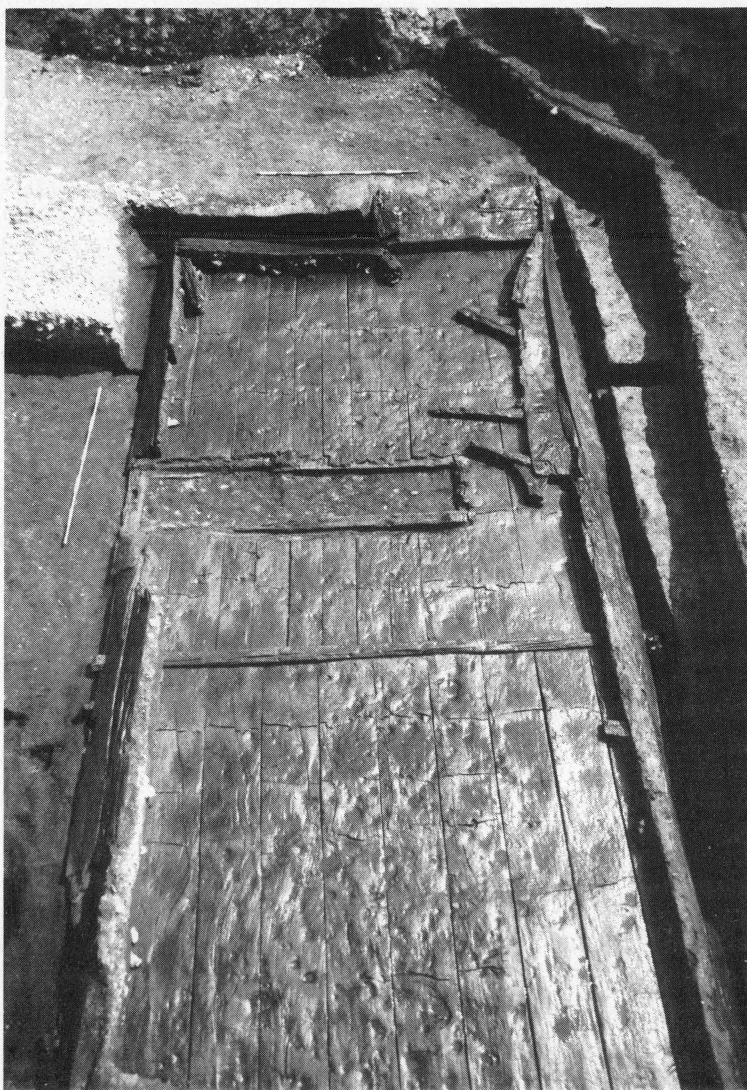
Fig 7. Courage Brewery site, Park Street, Southwark: wooden floor of dockside Roman warehouse, with entrance ramp in the top right hand corner. Photography by courtesy of the Museum of London
