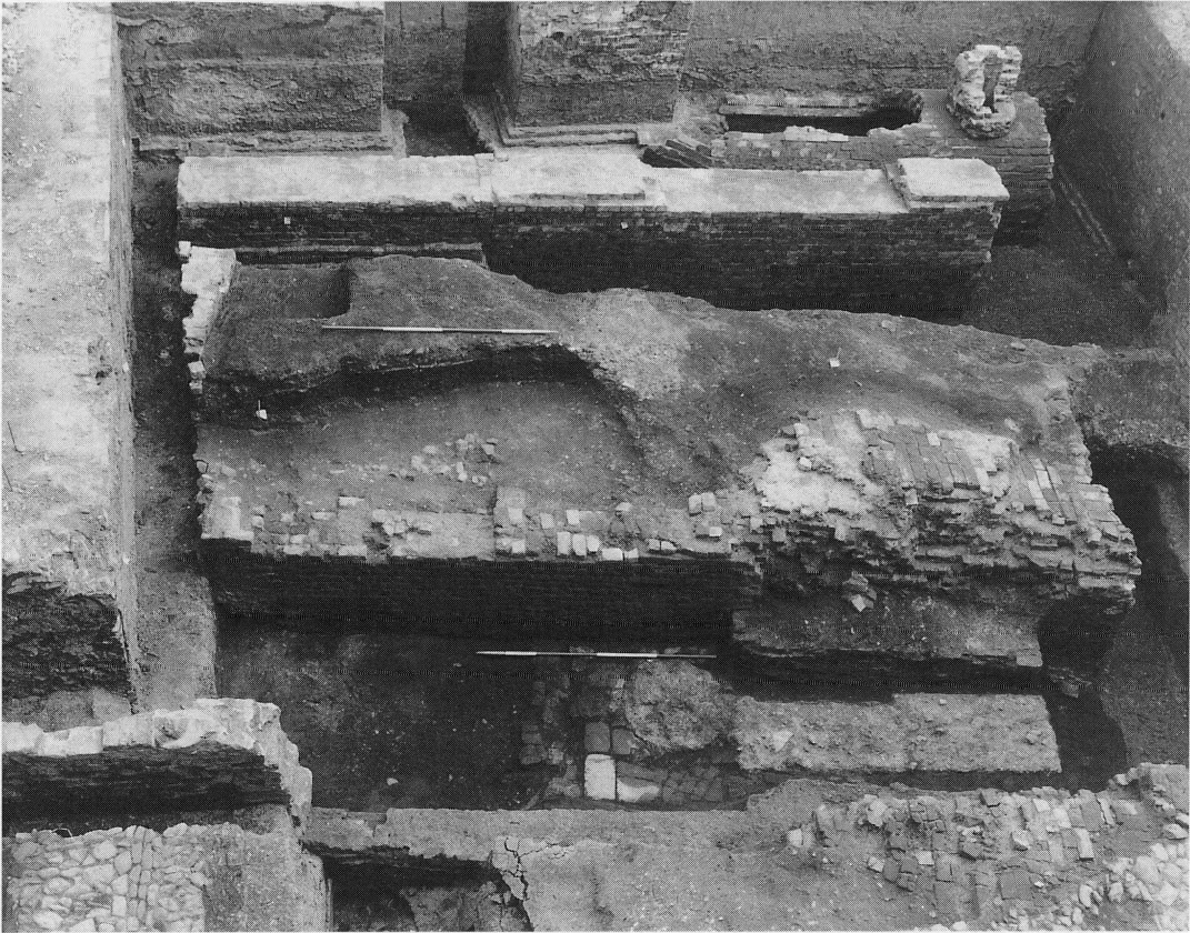
Fig 7 Hopton Street: furnace and flues of a late 18th century glassworking kiln with part of a 19th century Pellatt glass house in the background. (Photograph by Tim Loveless for PCA)
