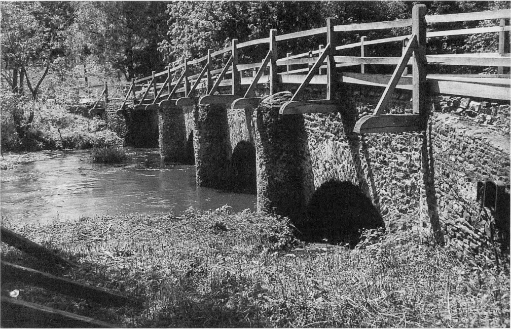
Fig 4 Tilford west bridge, Tilford. (Photograph by SCAU)
