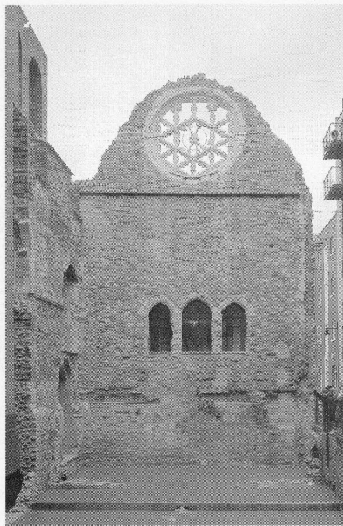
Fig 10 Winchester Palace, Clink Street: rose window of the great hall of medieval Winchester Palace after recent cleaning and repair. (Photograph by MoLAS)
