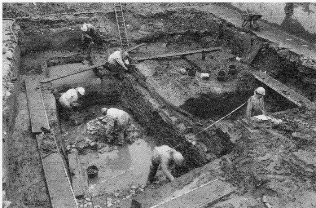
Fig 12 Bermondsey Wall West, Chambers Street, SE16: overview of site showing wattle revetment under excavation. (Photograph by PCA)
