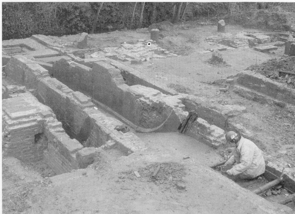
Fig 8 Bennett's Mill, Merantun Way, SW19: showing the main race and wheel pit. (Photograph by MoLAS)
